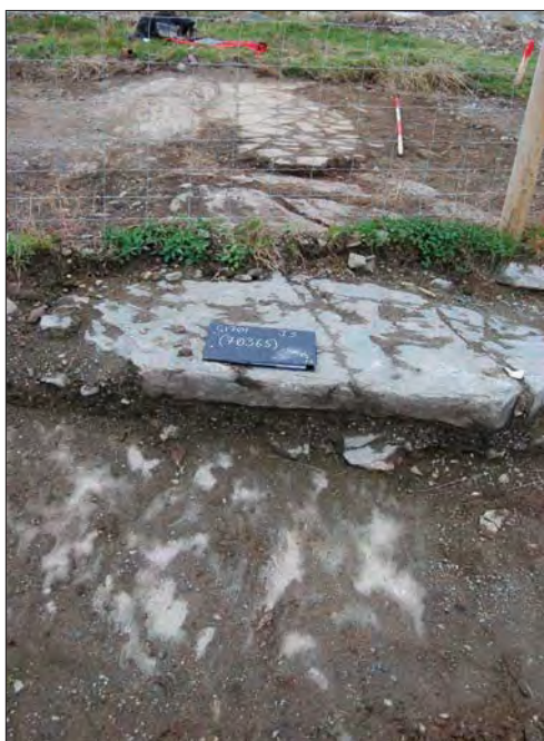
Plate 211. Large stone threshold slab leading to an internal concrete floor (70365) leading into the Trefignath Farmhouse
