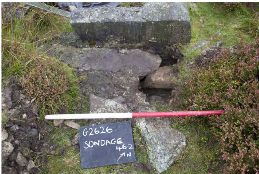
Plate 13: Plan shot of sondage 46.2 showing stone and concrete capping of culvert [4603]; scale: 1x1m (archive reference: G2626_035).
