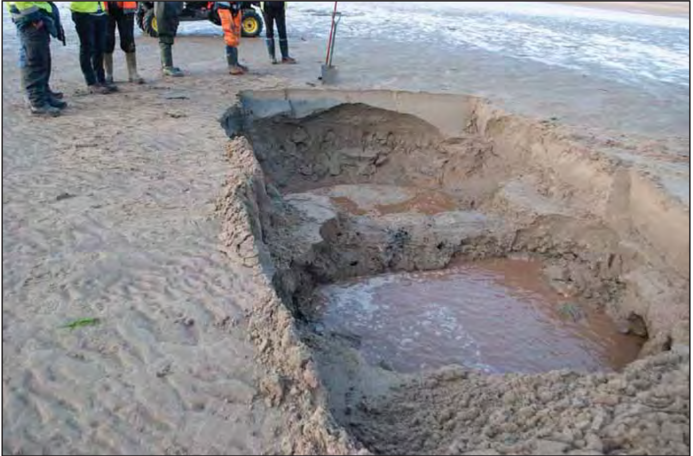
Plate 05: Excavation 1; no scale (archive reference: G2619_032).
