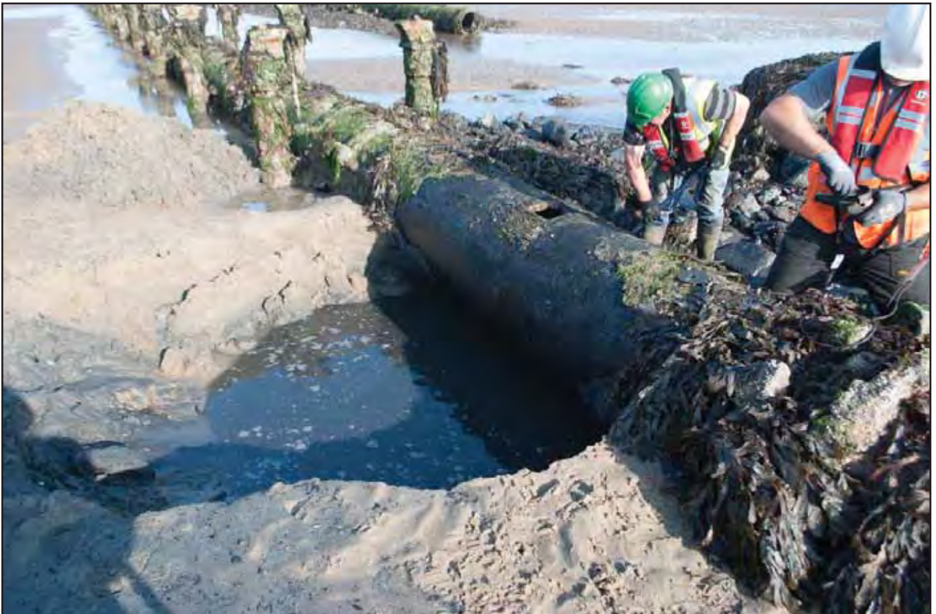
Plate 16: Excavation 9; no scale (archive reference: G2619_015).
