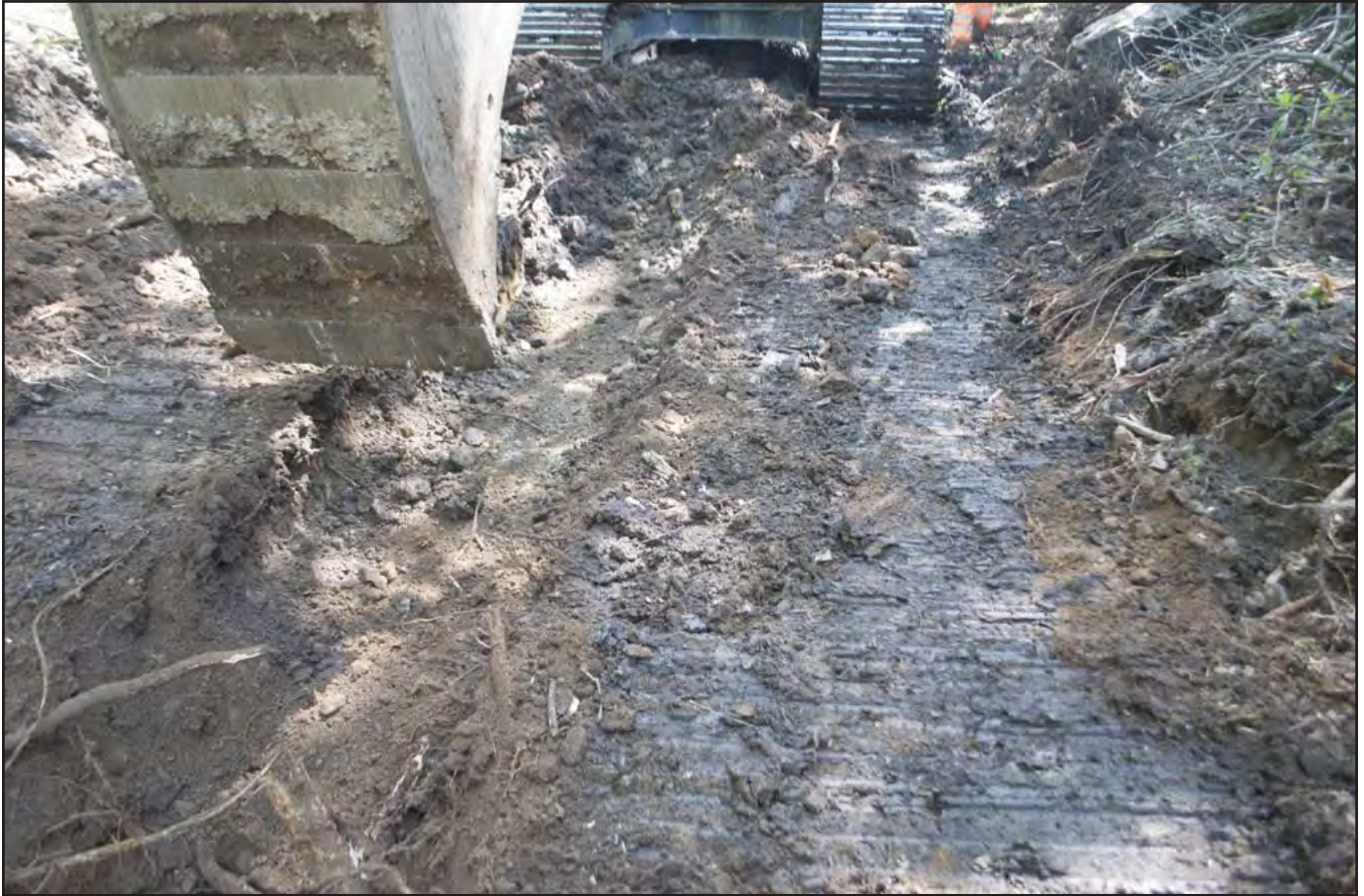
Plate 09: Pipe trench stripped to natural; scale not used; view from N (archive reference: G2601_117).
