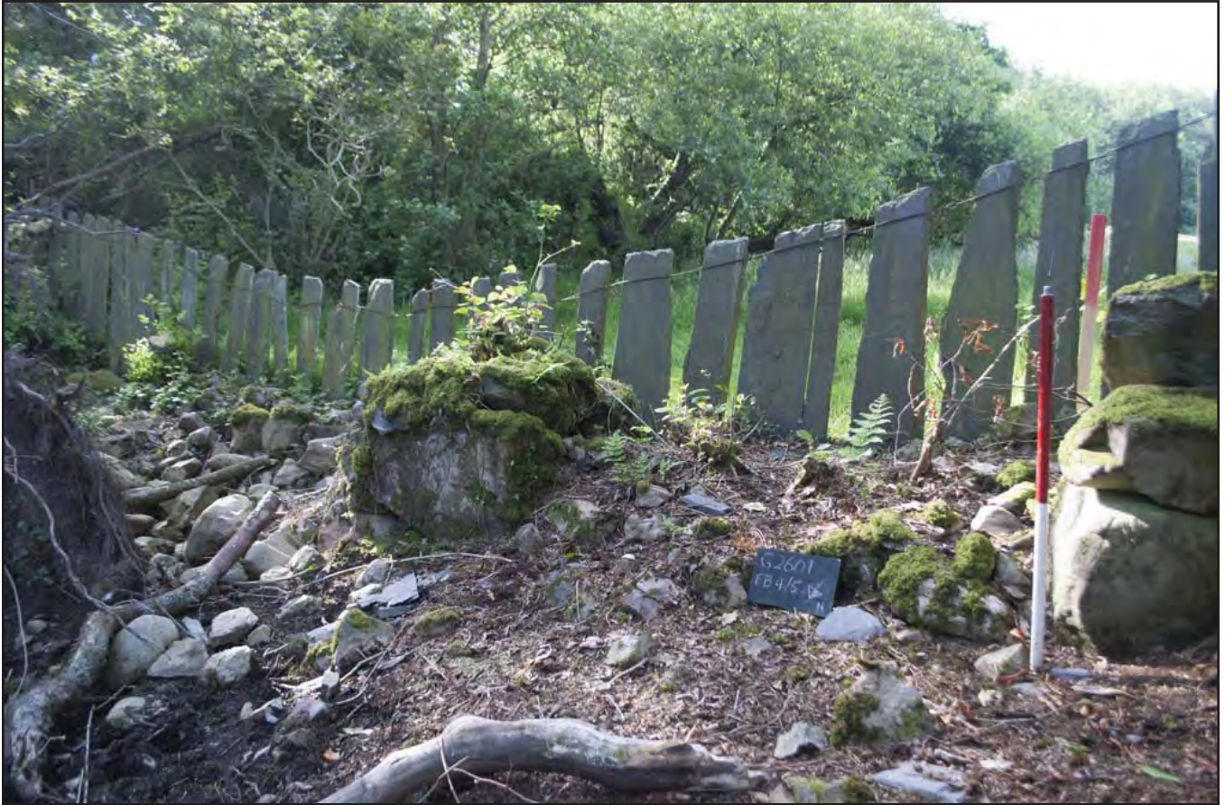
Plate 07: Fallen stone wall on NW side of slate fence; scale 1x1m; view from NW (archive reference: G2601_090).
