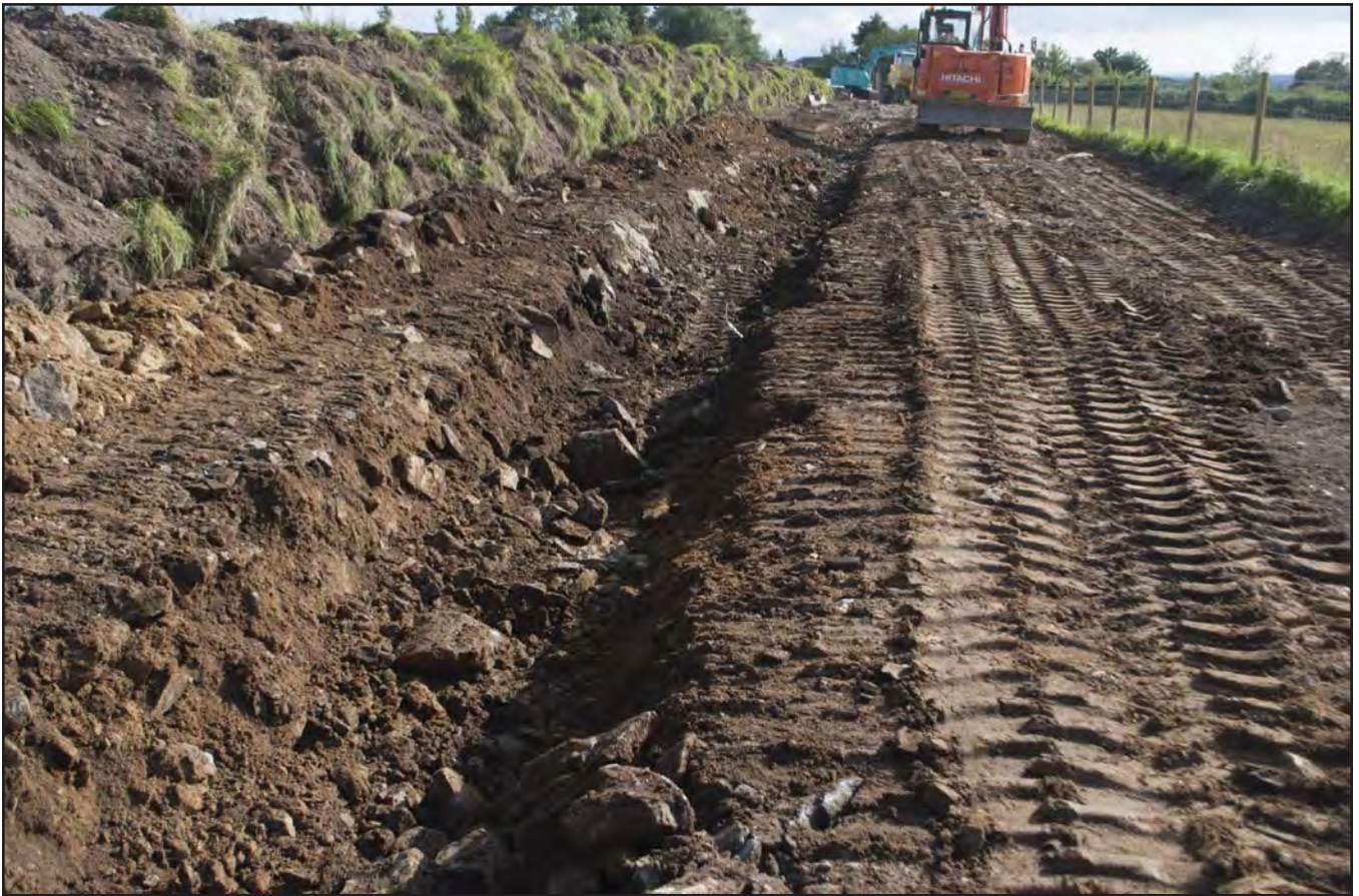
Plate 29: Pipe trench through bedrock; scale not used; view from SE (archive reference: G2601_243).
