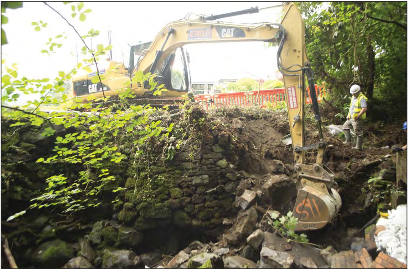
Plate 15: General view of revetment wall removal by machine; scale ; view from E (archive reference: G2616_055).
