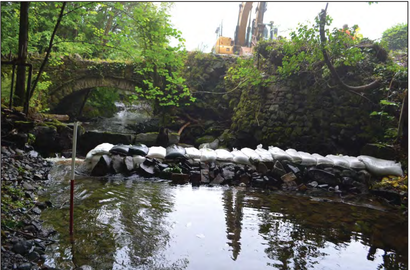
Plate 14: View from NE of weir showing sandbagging and the bridge to the rear; scale 1 x 1m; view from NE (archive reference: G2616_039).
