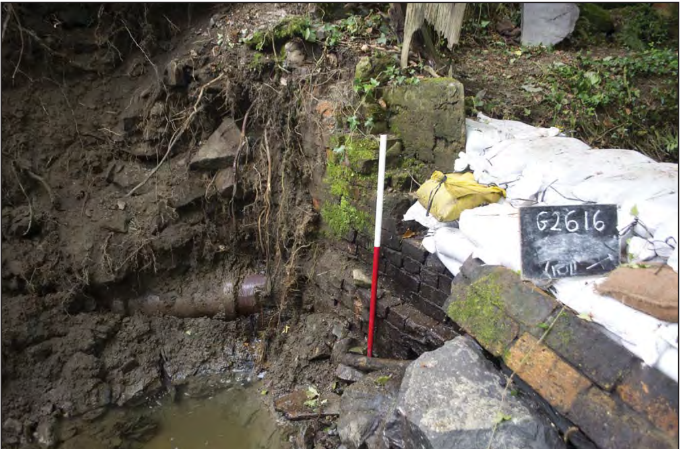
Plate 18: Detail showing the clay pipe and base of weir ; scale 1 x 1m; view from S (archive reference: G2616_066).
