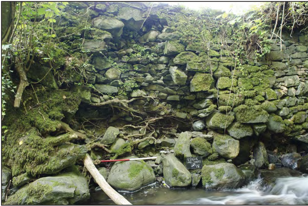
Plate 3: Breached section at wall; scale: 1 x 1m; view from: SE (archive reference: G2616_014).
