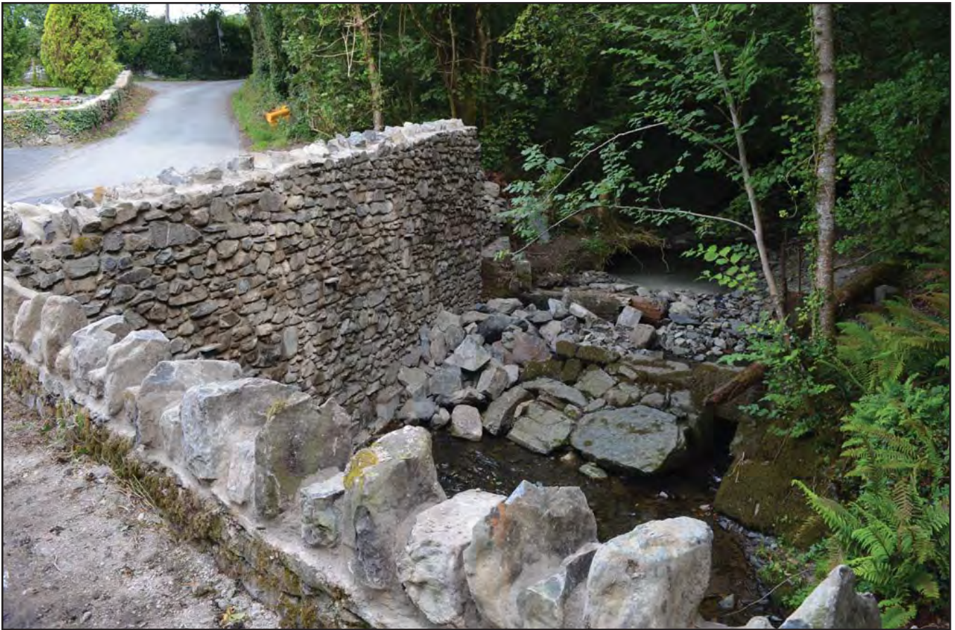
Plate 31: General view of revetment walling from the bridge showing bonding with the sluice; scale not used; view from SSW (archive reference: G2616_152).
