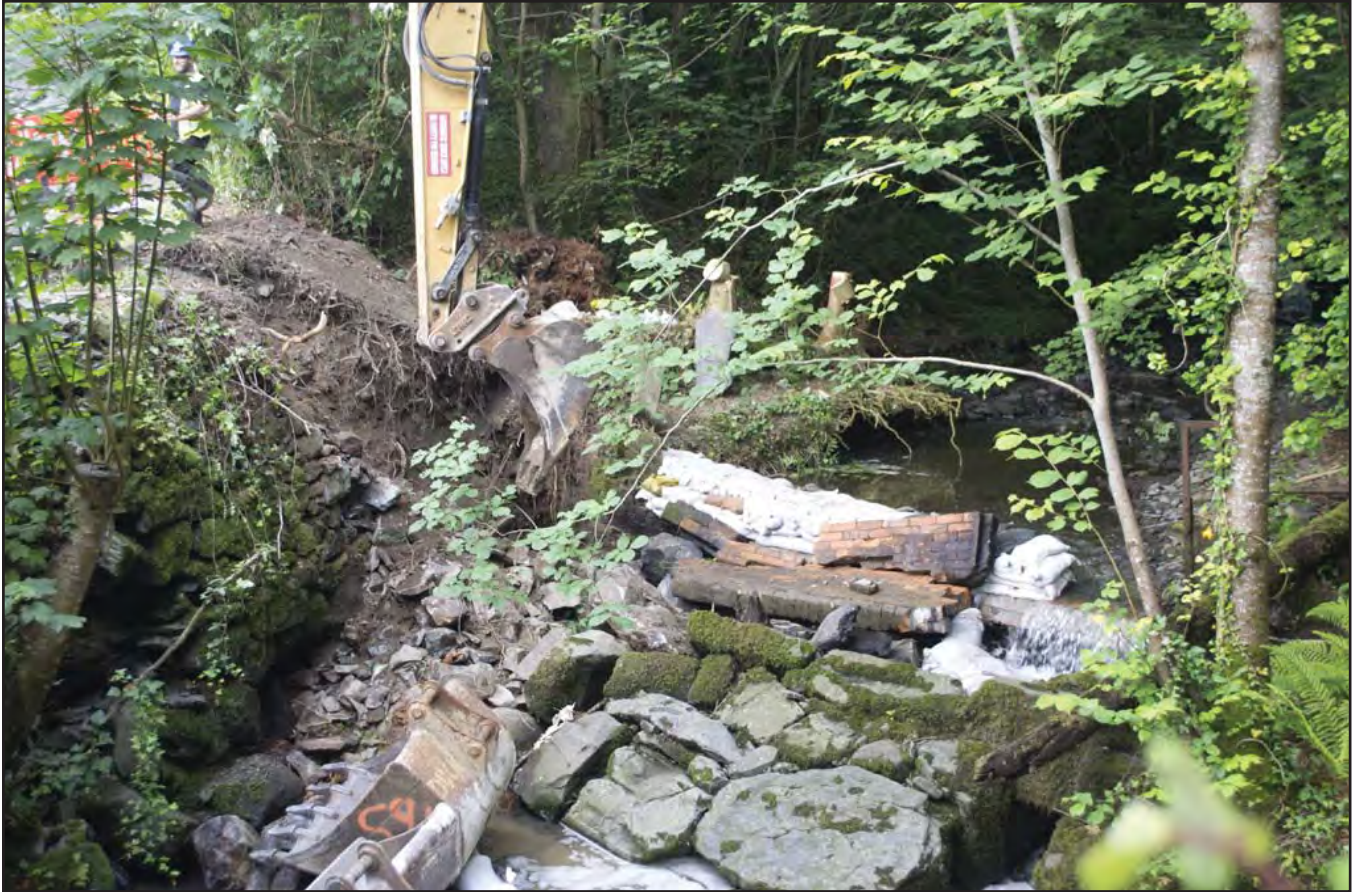
Plate 17: As above, but with a clay drainage/sewerage pipe cutting through the base of the weir wall; scale ; view from S (archive reference: G2616_062).
