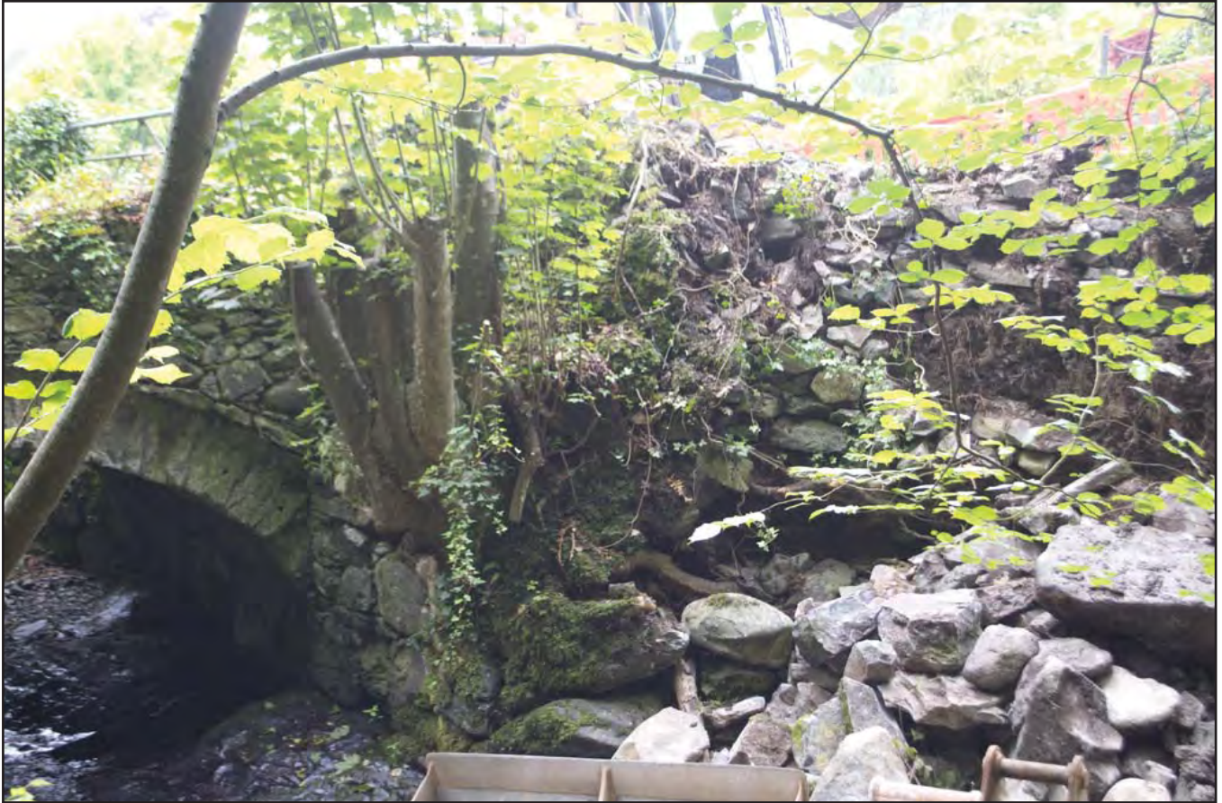
Plate 19: Detail showing collapsed walling in the return of the revetment wall near the bridge; scale: not used ; view from E (archive reference: G2616_072).
