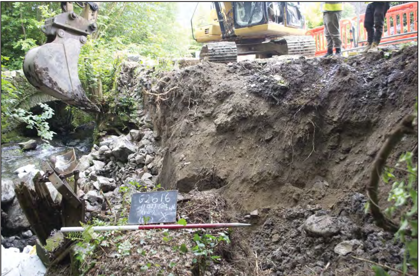
Plate 20: Rough section, machine cut, through revetment 100 and backfill 101, from the NW riverbank; scale 1 x 1m; view from NE (archive reference: G2616_078).
