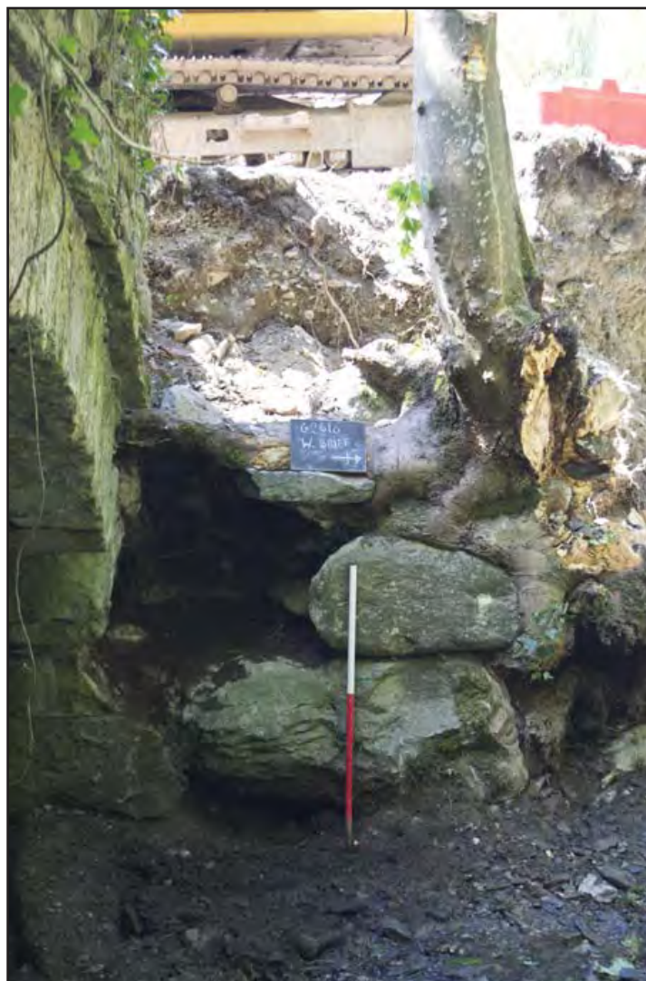
Plate 22: View of revetment walling [104] adjacent to the bridge part removed to enable the tree root removal; scale 1 x 1m; view from SSE (archive reference: G2616_110).
