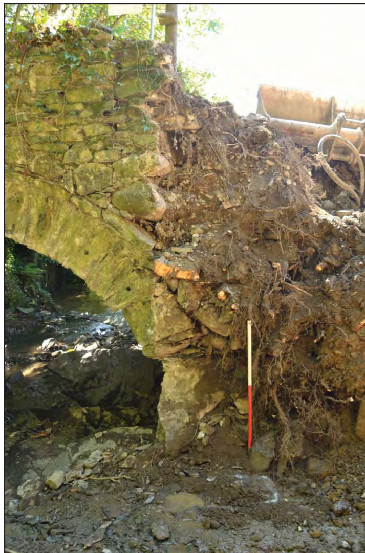
Plate 24: Exposed bridge arch after removal of tree and wall; scale 1x 1m; view from E (archive reference: G2616_119).
