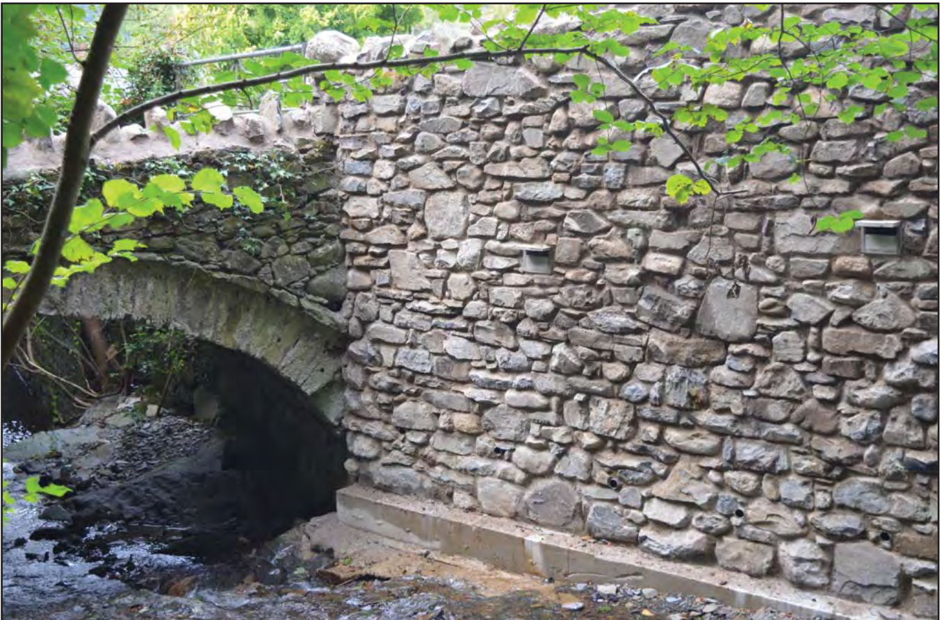
Plate 30: General view showing the butt joint of the revetment walling with the 18th century bridge; scale not used; view from SE (archive reference: G2616_148).
