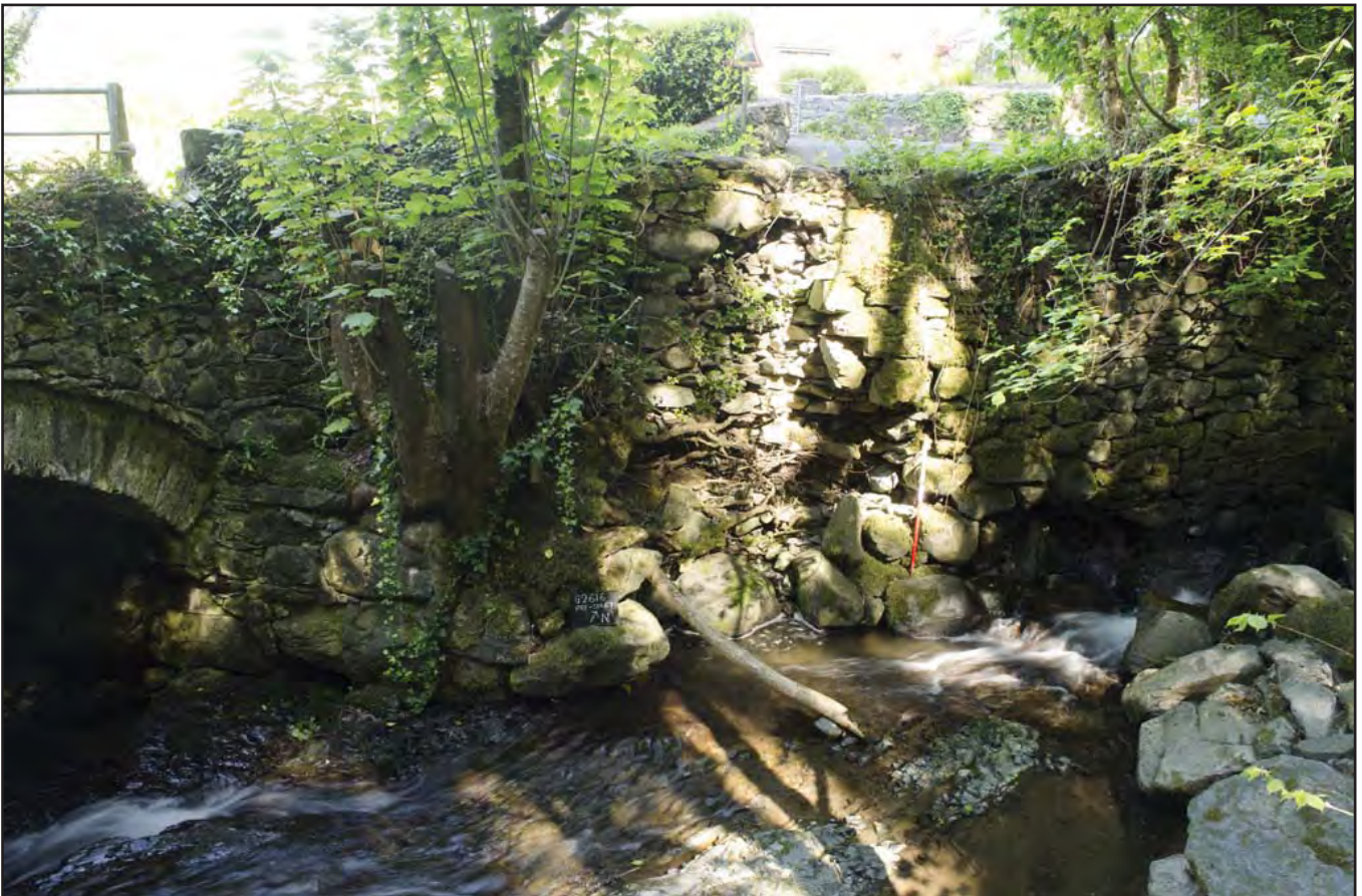
Plate 2: Location at the breach in the retaining wall; scale: 1 x 1m; view from: SE (archive reference: G2616_007).
