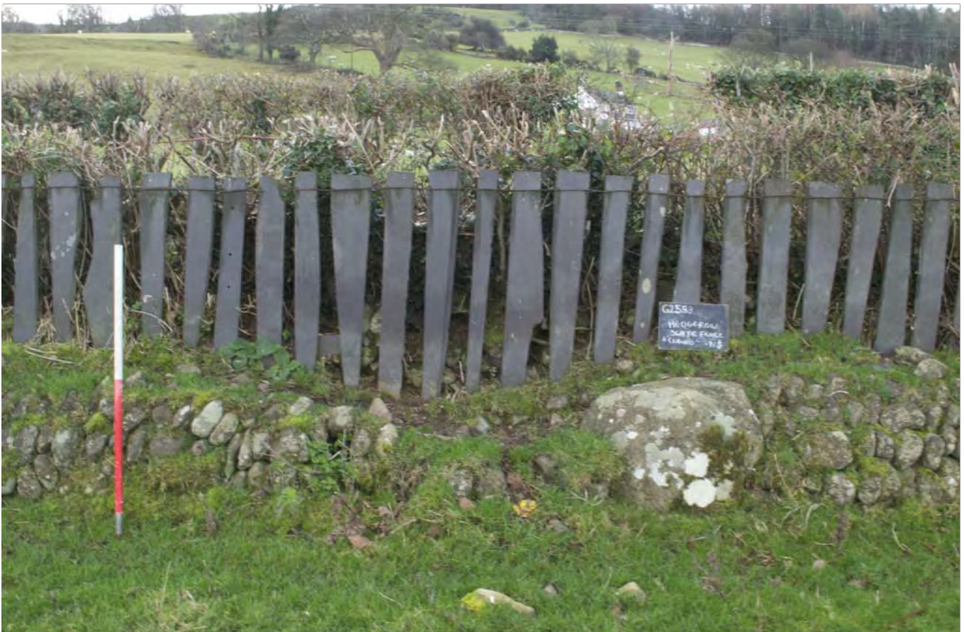
Plate 02: Hedge, clawdd and slate fence, scale: 1x1m (archive reference: G2588_012).
