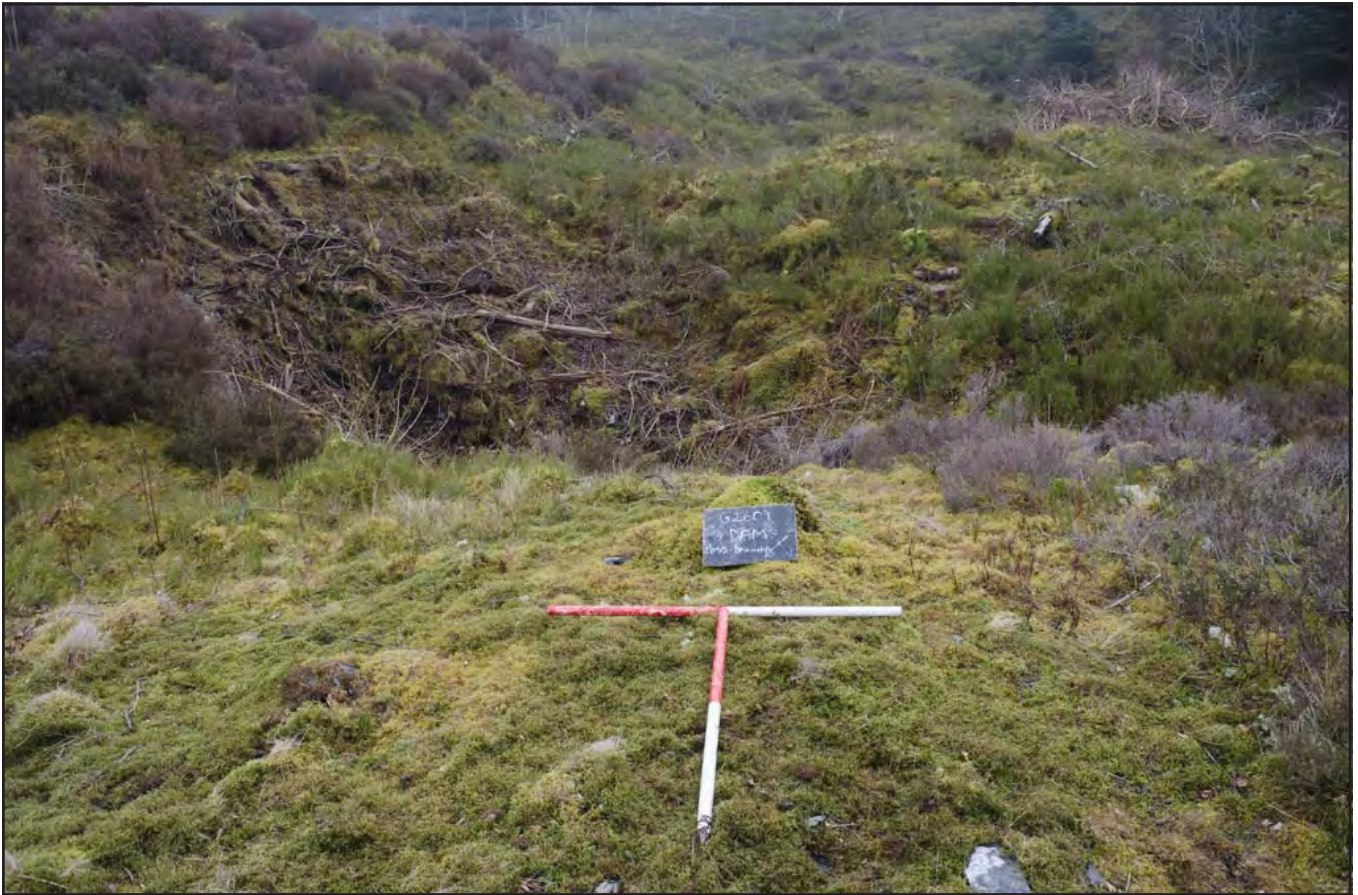
Plate 15: View of possible old breach in dam along with overflow; scale: 2x1m (archive reference: G2609_015).
