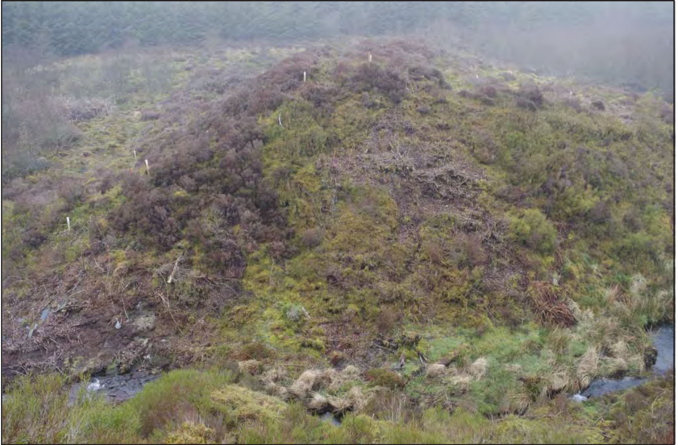
Plate 19: View of north-eastern side of dam showing breach (archive reference: G2609_019).
