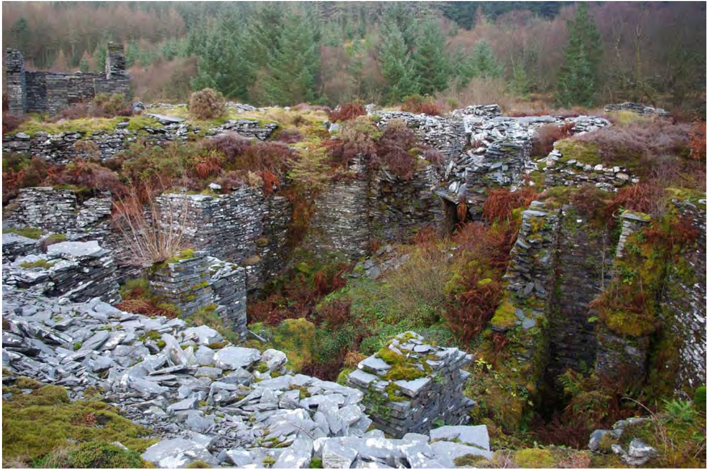
Plate 15 -Bryneglwys south (narrow vein). Wheelpits for water-powered chain incline. Weighbridge house in background
