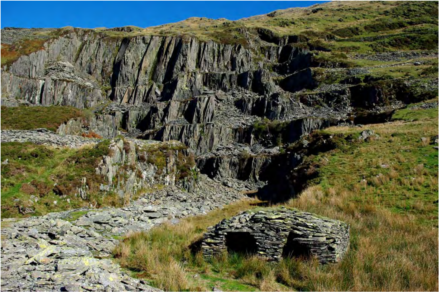
Plate 23 - Gorseddau Slate Quarry. Galleried pit with corbelled blast-shelter in foreground
