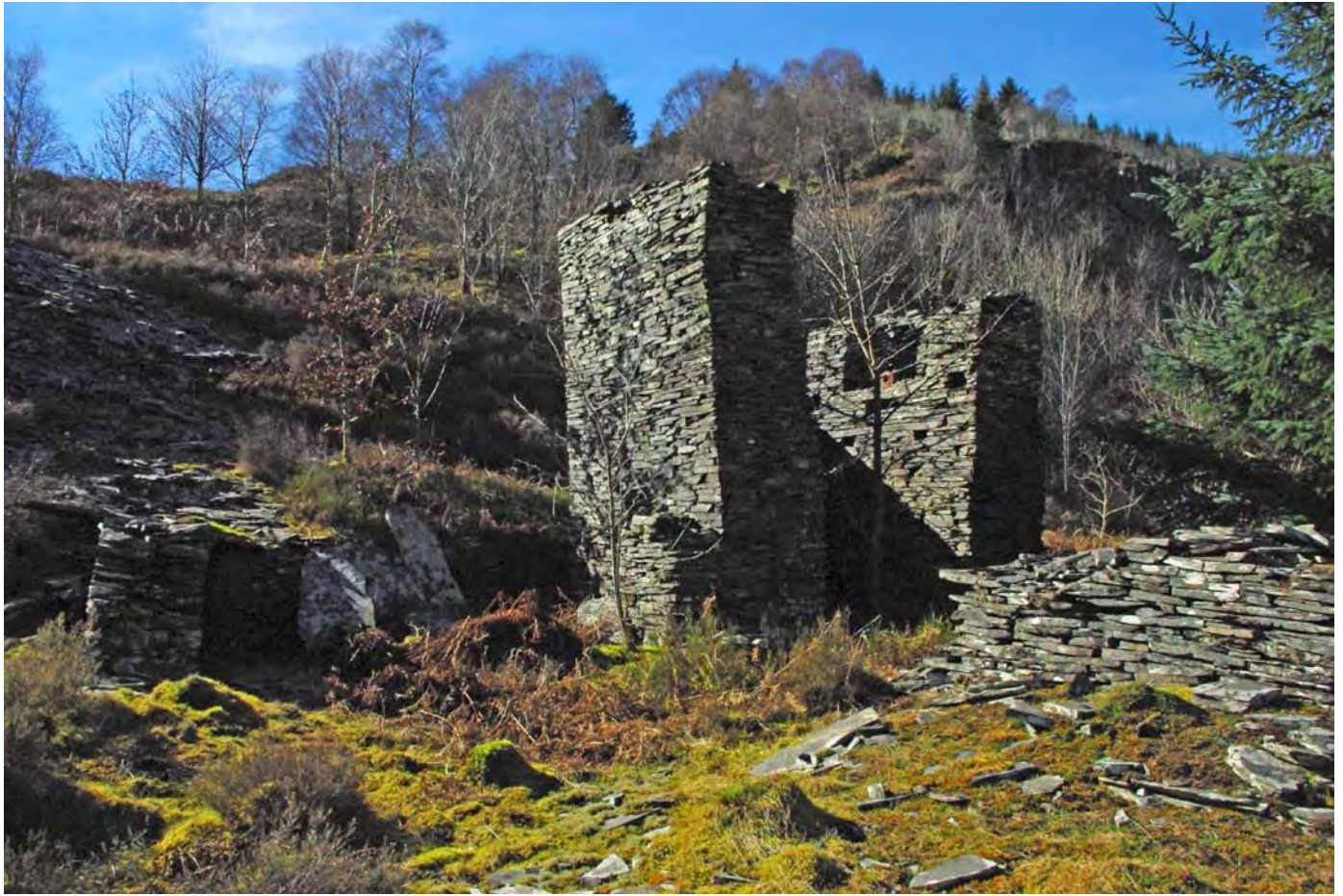
Plate 7 - Hen Gloddfa. Drum house and gwaliau at head of central incline
