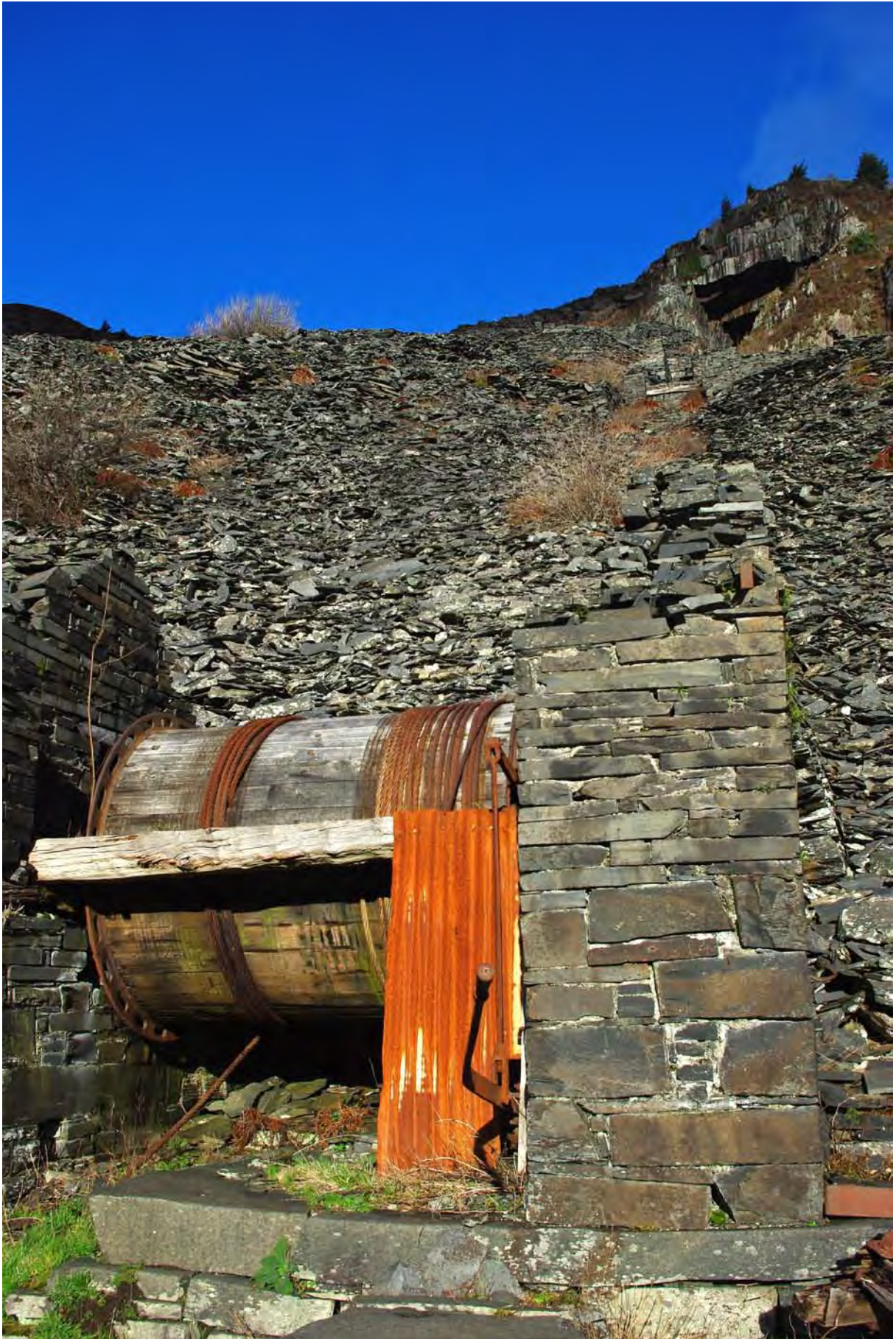
Plate 3 - Foel Grochan, south-west. Drum house one level up from the valley floor. Inclines behind in tips
