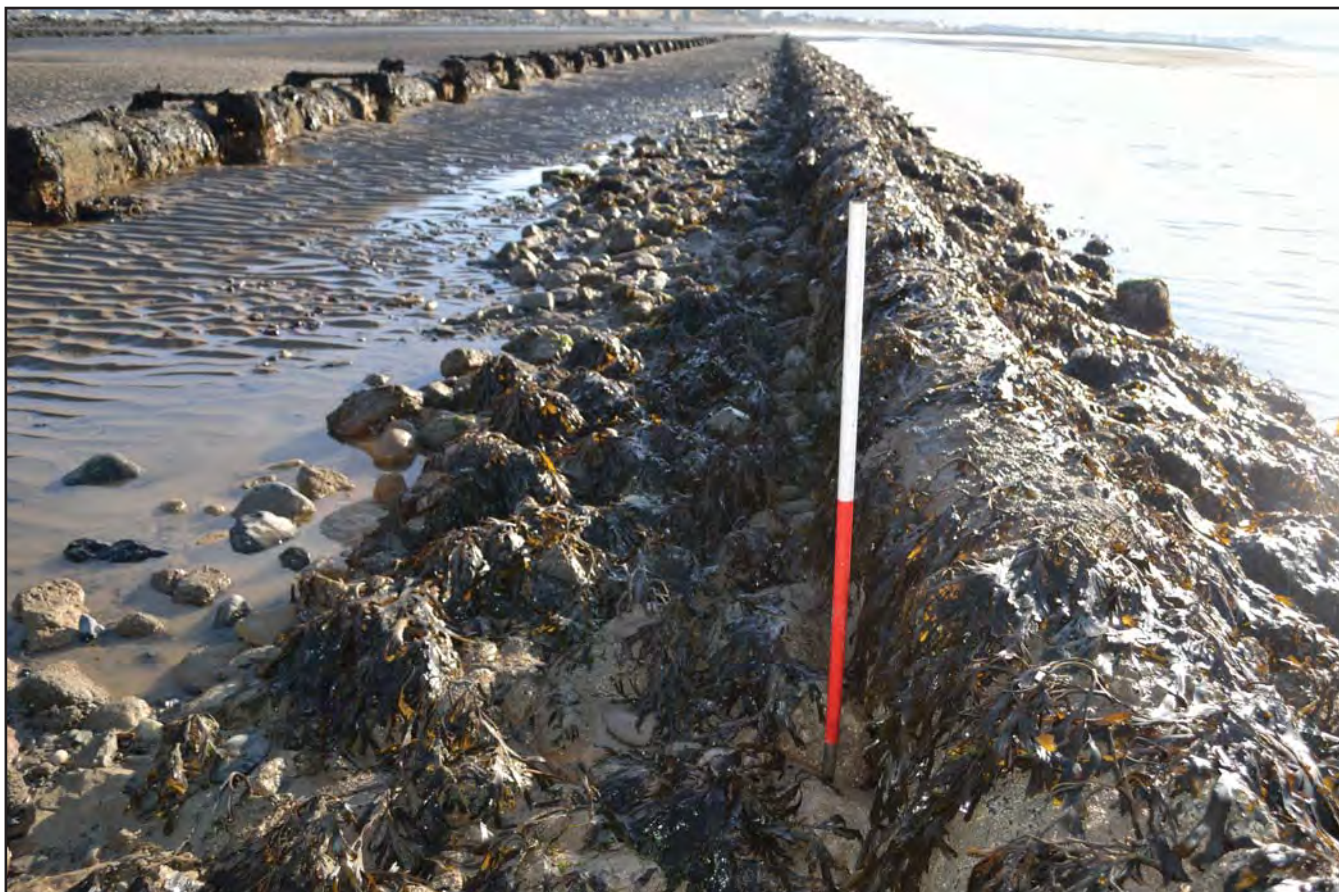
Plate 07: Material collecting around 1845 pipe, view to shore; scale: 1x1m (archive reference: G2600_015).
