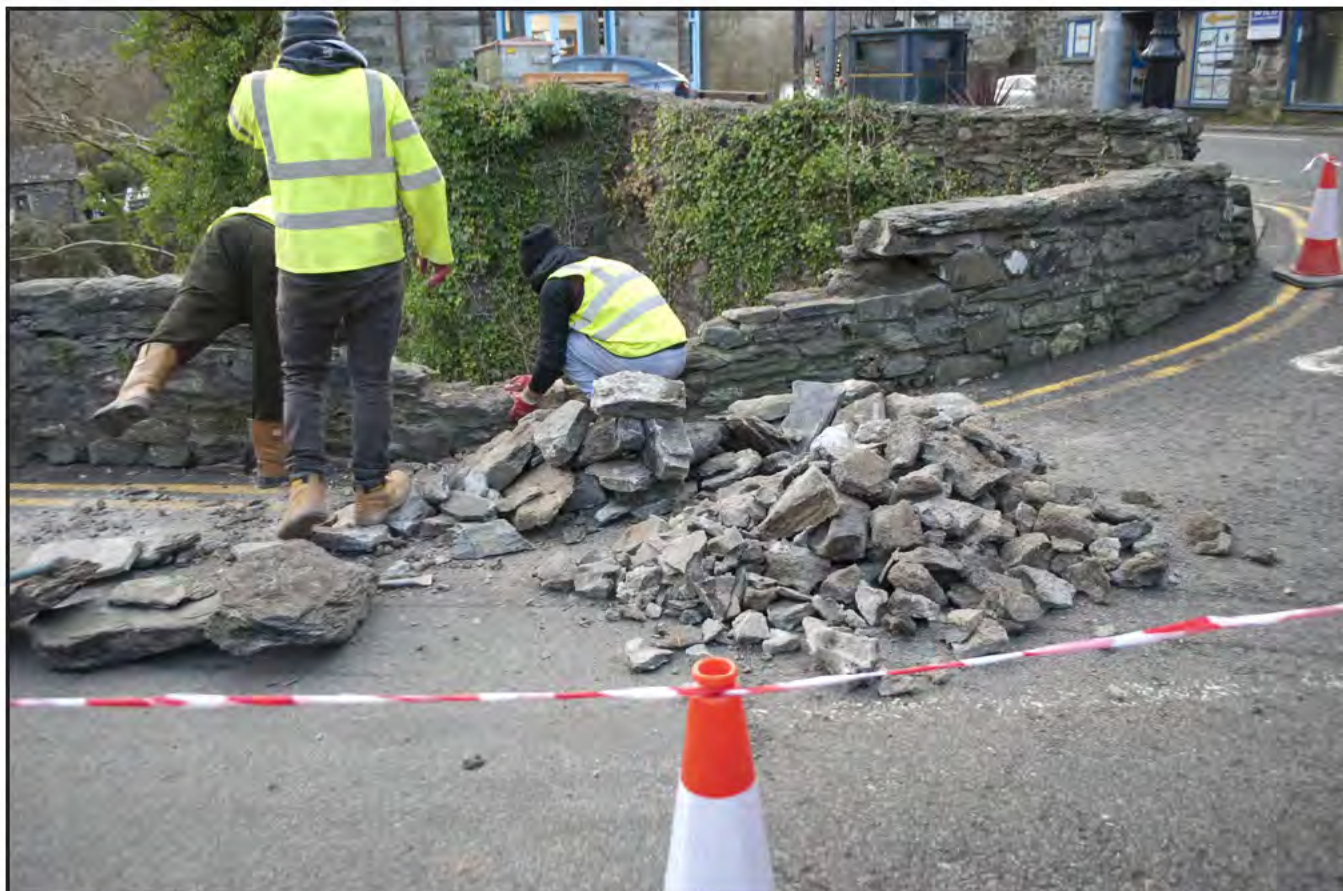
Plate 11: General view during wall demolition showing the hard mortar (in a pile); scale: not used (archive reference: G2587_023).
