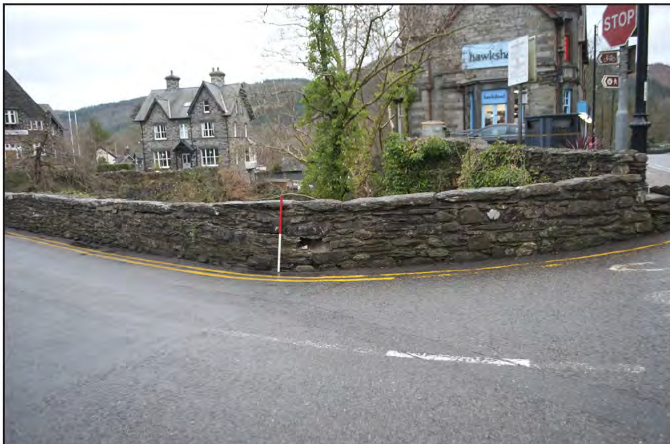
Plate 3: General view of damaged section of walling at southeast corner of Pont y Pair showing the splaying parapet from the A5 junction; scale: 2x1m (archive reference: G2587_004).
