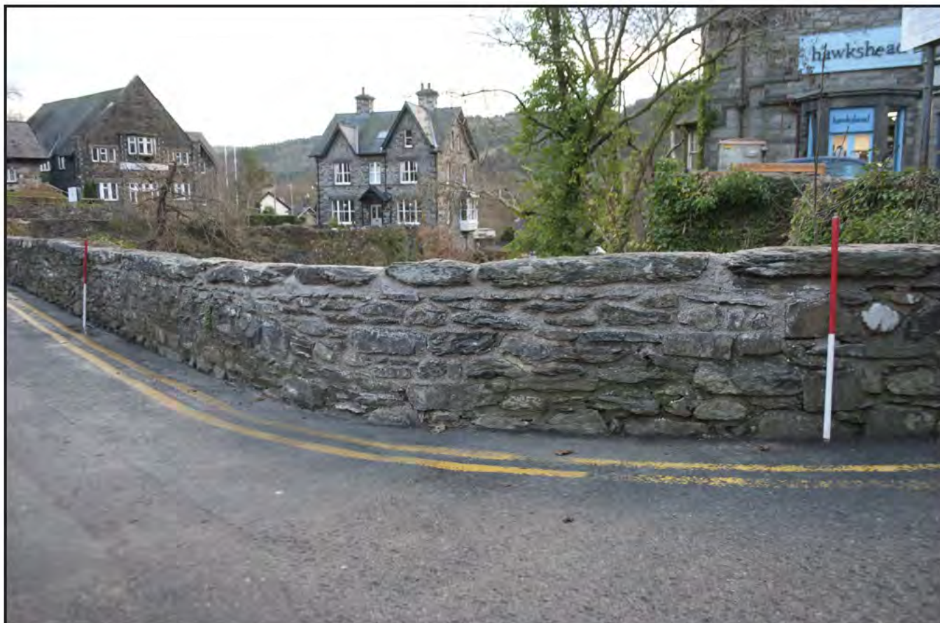
Plate 13: View of repaired southeast corner of the bridge parapet; scale: 2x1m (archive reference: G2587_031).
