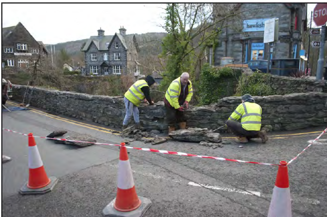
Plate 10: Action shot showing demolition work (by hand) taking place at the southeast corner of the parapet; scale: not used (archive reference: G2587_020).
