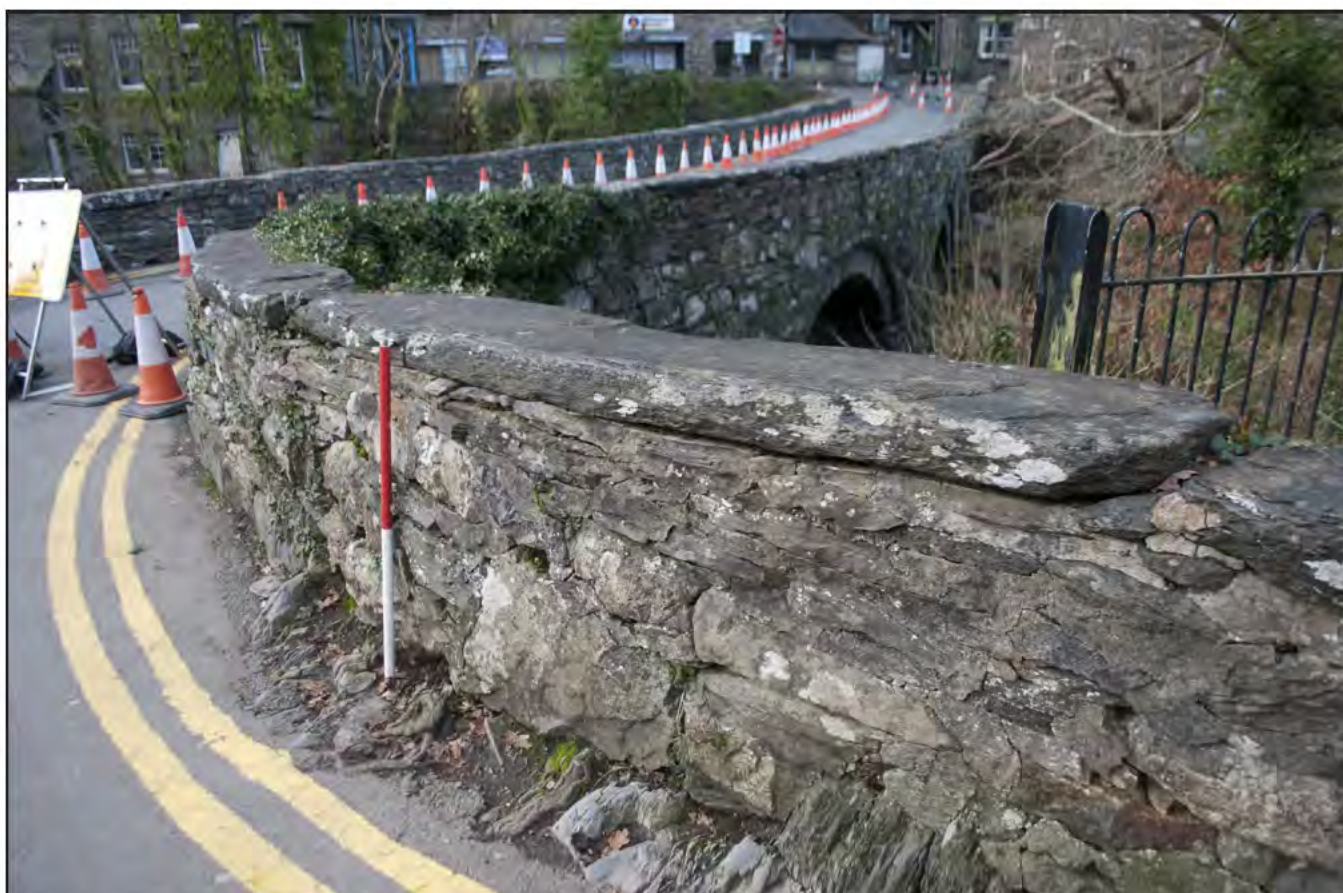
Plate 8: View of slipped coping stone at the northwest corner of the bridge parapet walling; scale: 1x1m (archive reference: G2587_016).
