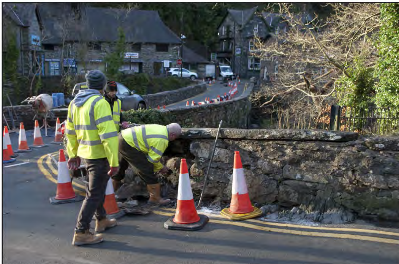
Plate 17: General shot of repair work to stones below the large coping stone at the northwestern end of the parapet; scale: not used (archive reference: G2587_037).
