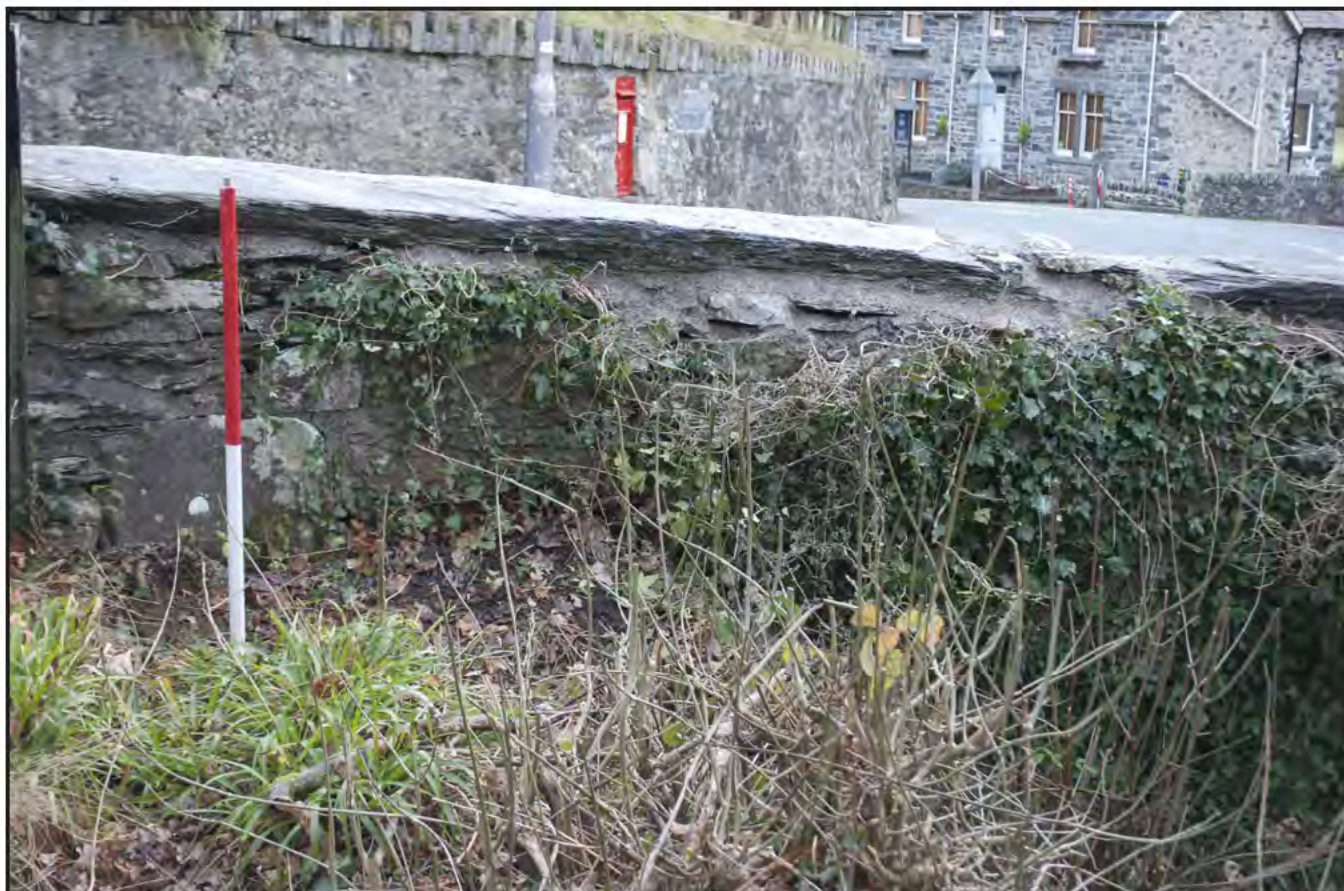
Plate 19: View of riverward side of the repaired northwest section of Pont y Pair parapet; scale: 1x1m (archive reference: G2587_039).
