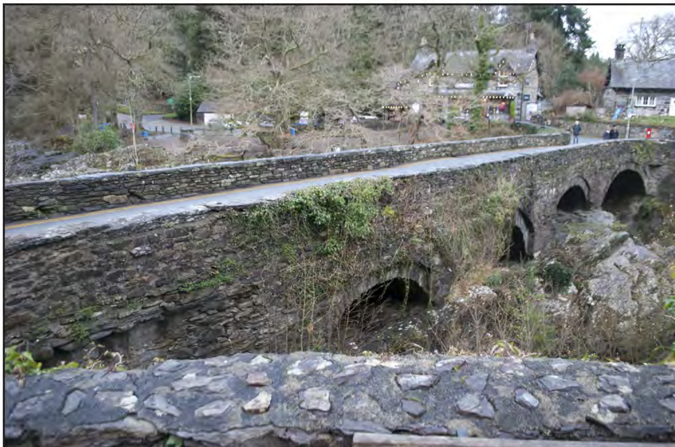
Plate 1: General view of Pont y Pair showing the side elevation with arches, reveals and voussoirs; scale: not used (archive reference: G2587_006).
