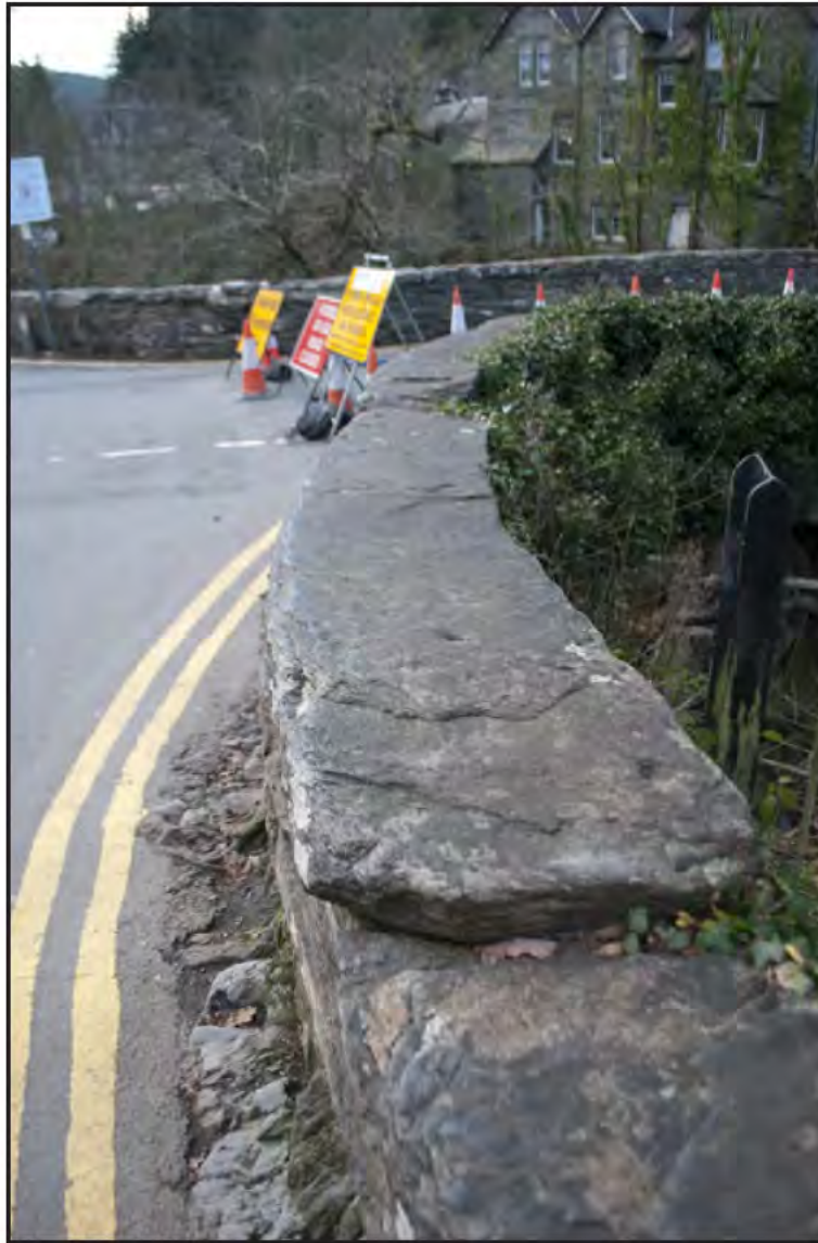
Plate 9: Detail of very large (3.2m long by 0.1m high) slipped coping stone; scale: not used (archive reference: G2587_017).
