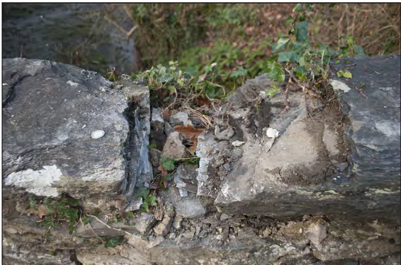
Plate 16: Area of damaged coping at the northwest end of the parapet; scale: not used (archive reference: G2587_034).
