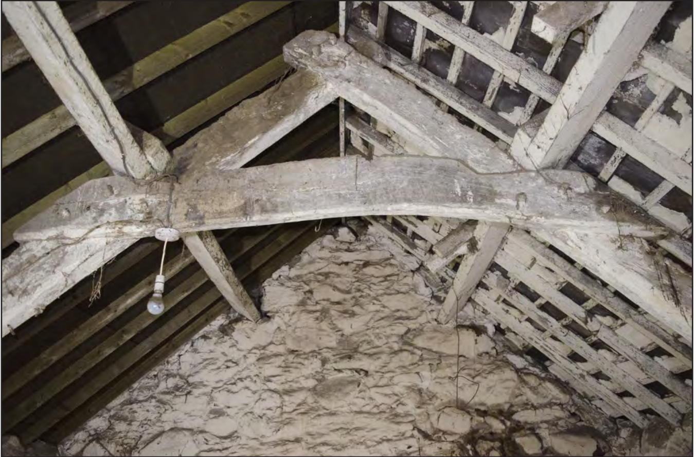
Plate 27: Stable 2: detail of A-Frame Truss from southwest wall; scale: not used (archive reference: G2586_038).
