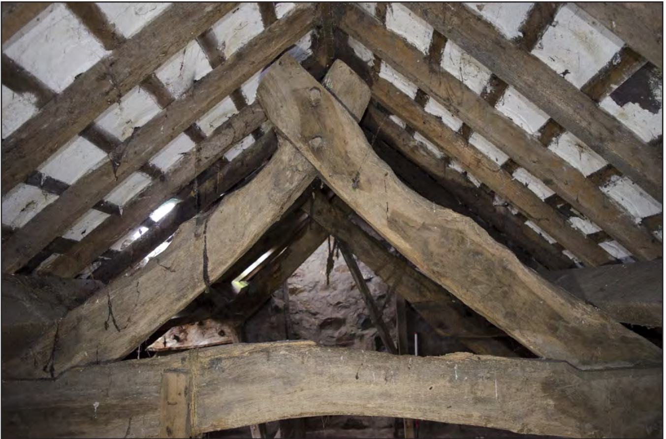
Plate 39: Store Room 3: detail of upper portion of A-Frame Truss (a); scale: not used (archive reference: G2586_052).
