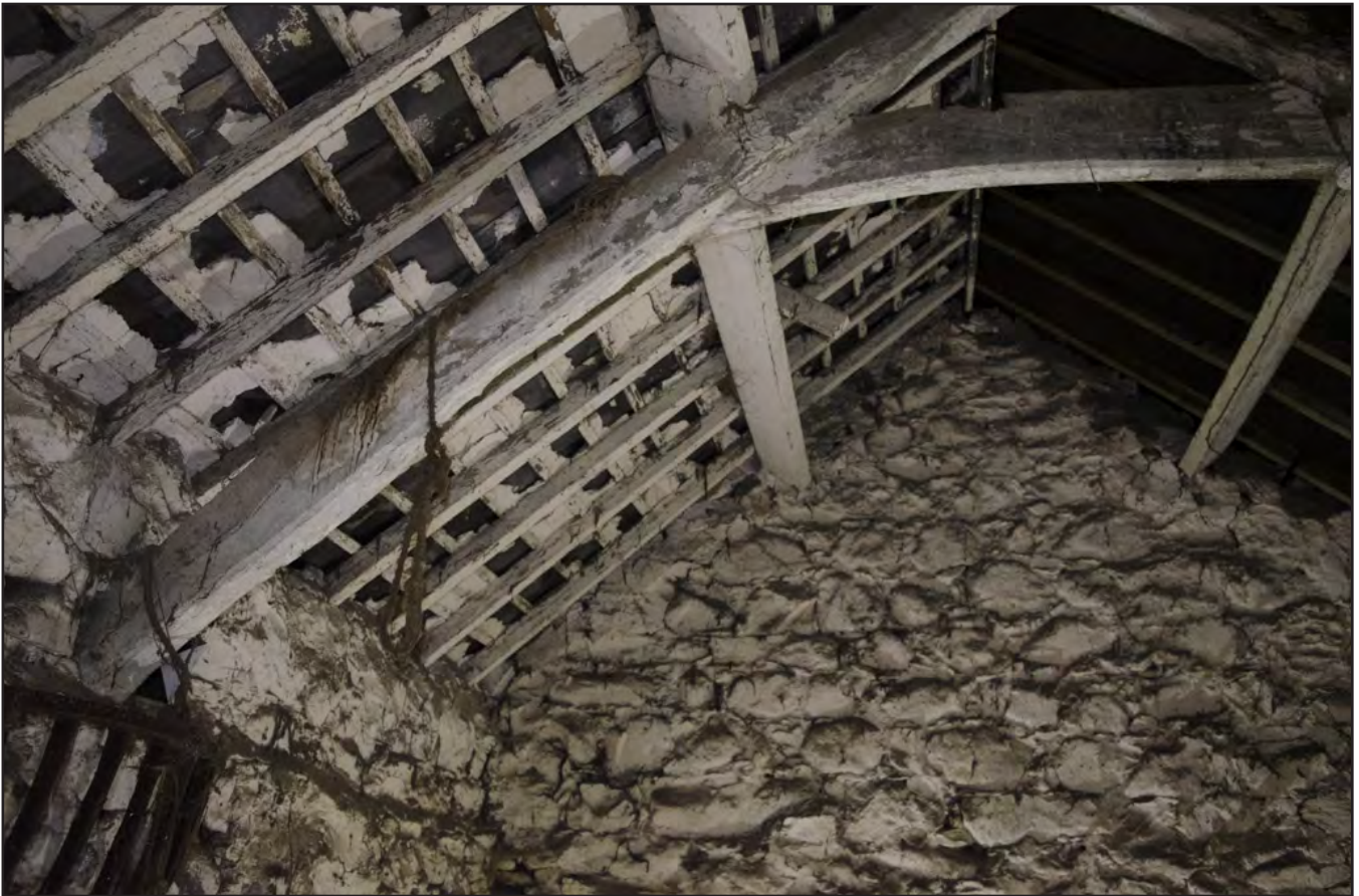
Plate 29: Stable 2: detail of A-Frame Truss from northeast wall; scale: not used (archive reference: G2586_040).
