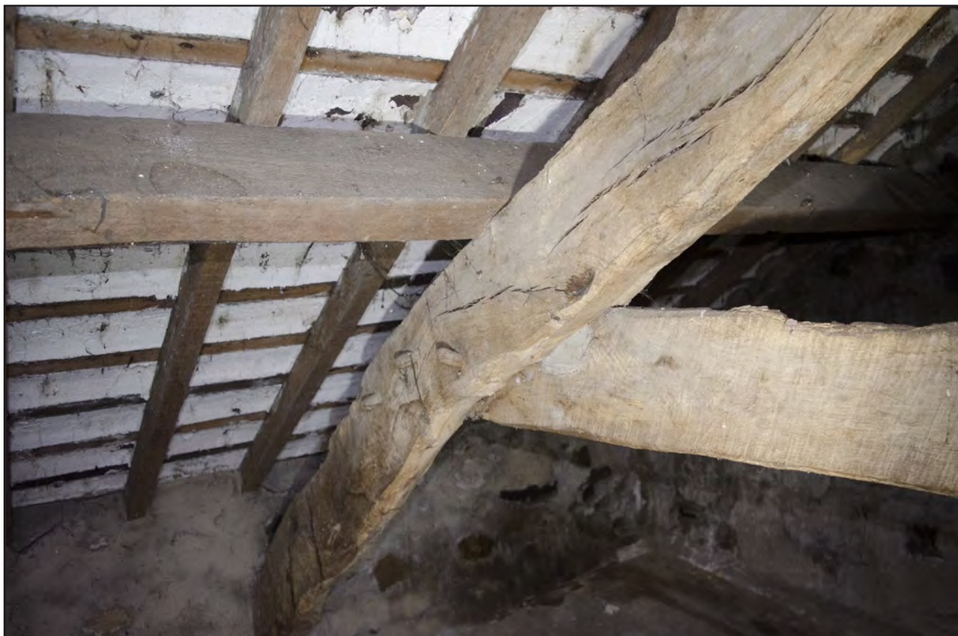
Plate 37: Store Room 3: detail of pegging apex on A-Frame Truss (a); scale: not used (archive reference: G2586_050).
