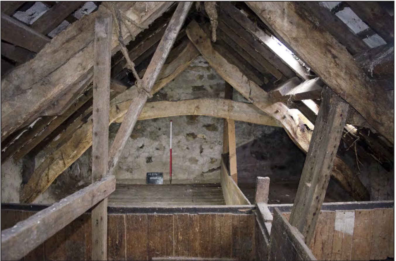
Plate 31: Store Room 3: detail of A-Frame Truss (a); scale: 1x1m (archive reference: G2586_043).
