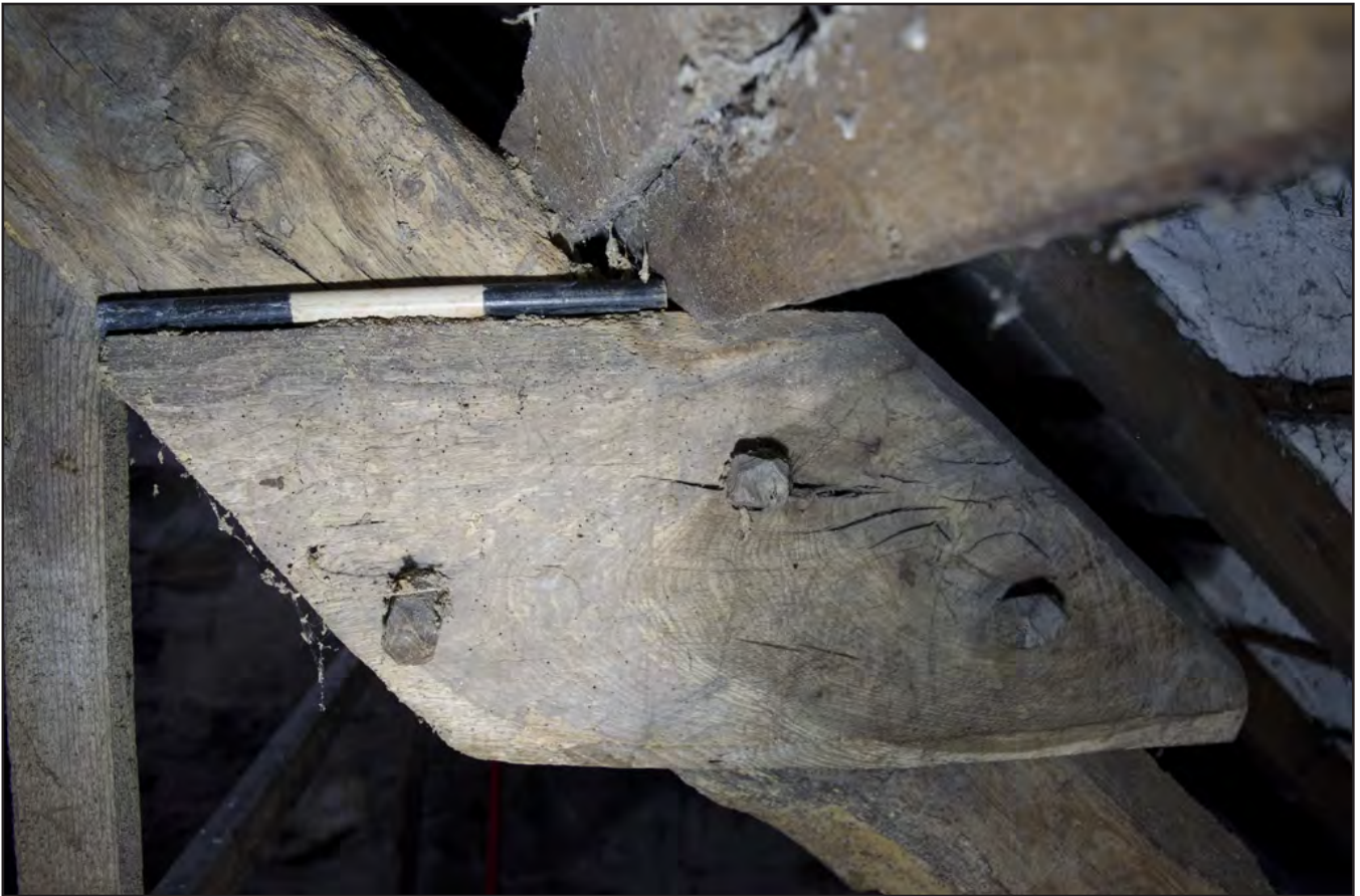
Plate 33: Store Room 3: detail of pegged attachment on A-Frame Truss (b); scale: 1x0.3m (archive reference: G2586_046).
