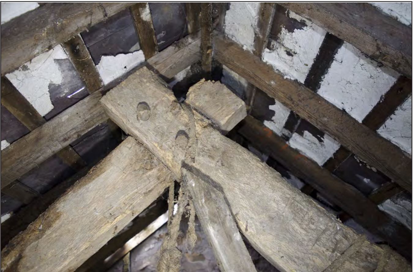
Plate 34: Store Room 3: detail of pegged apex on A-Frame Truss (b); scale: not used (archive reference: G2586_047).
