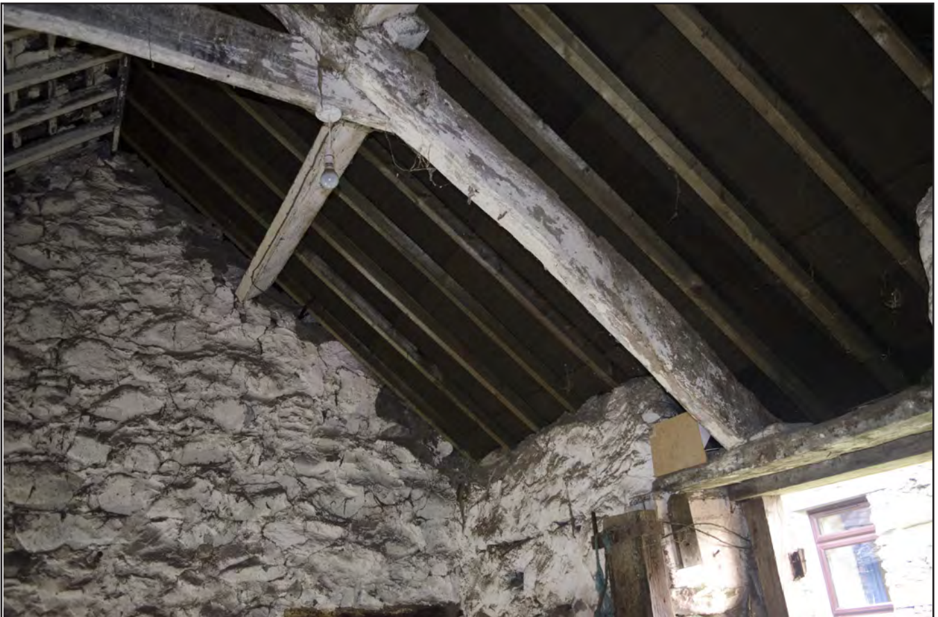
Plate 30: Stable 2: detail of A-Frame Truss from northeast wall; scale: not used (archive reference: G2586_042).
