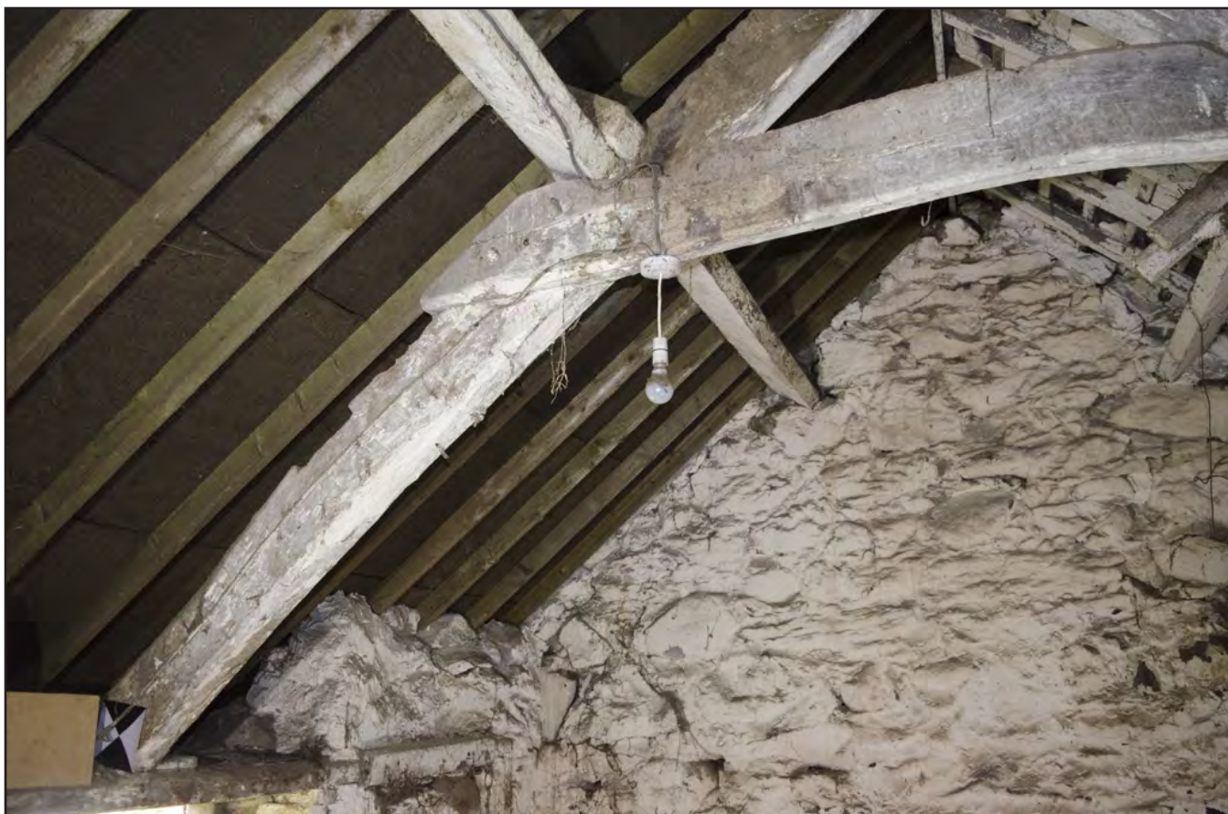
Plate 26: Stable 2: detail of A-Frame Truss from southwest wall; scale: not used (archive reference: G2586_037).
