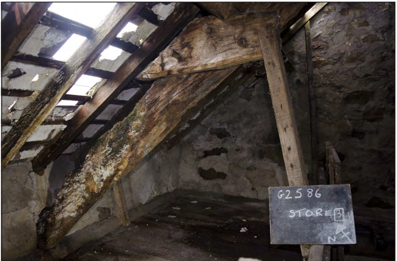
Plate 36: Store Room 3: detail of rotted end on A-Frame Truss (b); scale: not used (archive reference: G2586_048).
