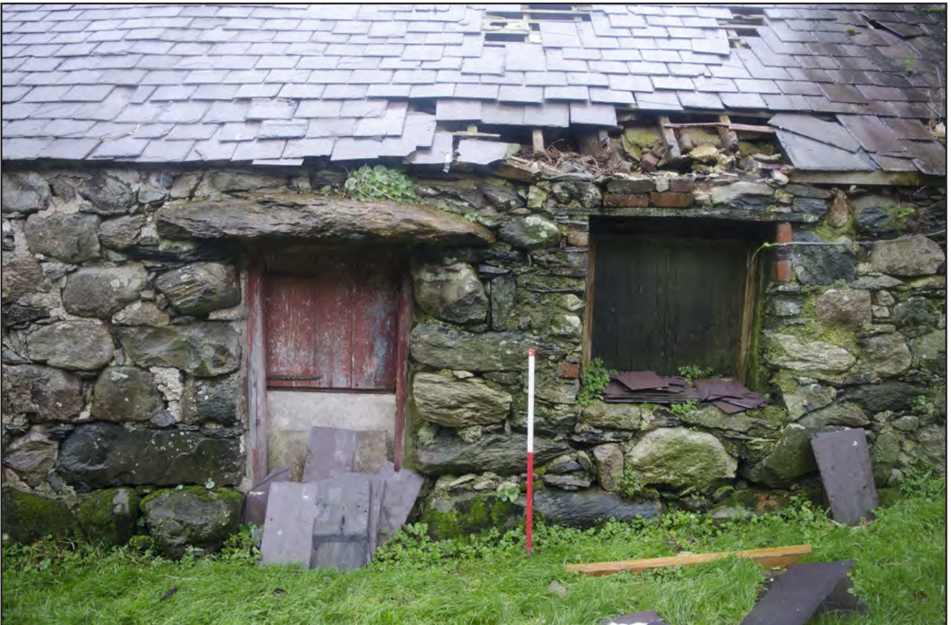
Plate 8: Southwest facing elevation: modern window and doorway with large stone lintel at rear of building; scale: 1x1m (archive reference: G2586_010).
