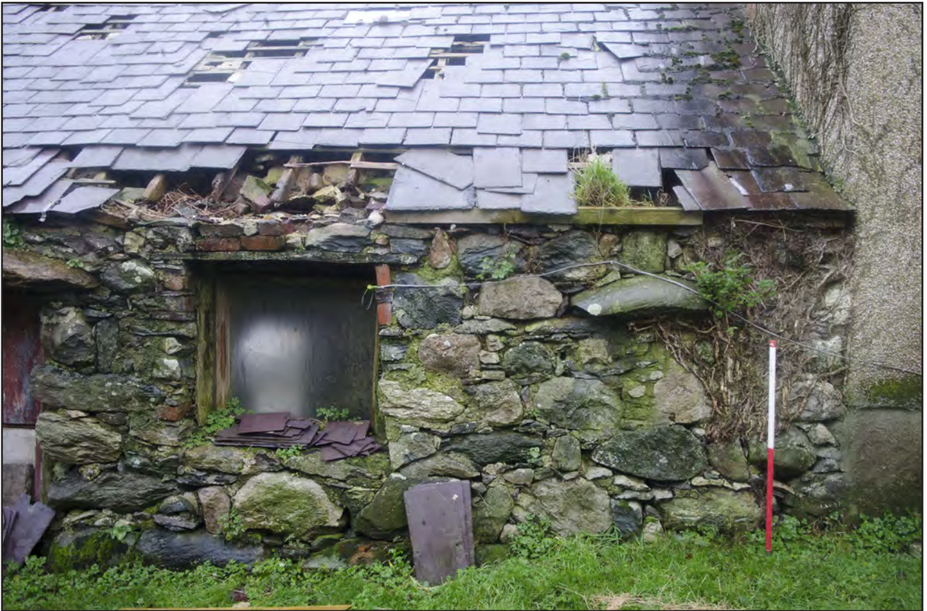
Plate 7: Southwest facing elevation: modern window and blocked up window at rear of building; scale: 1x1m (archive reference: G2586_009).
