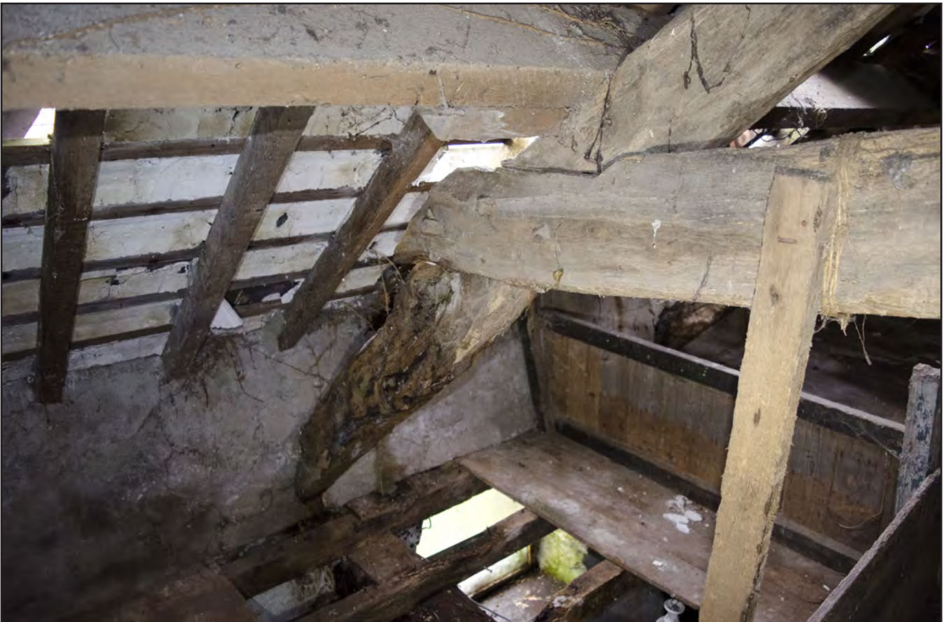
Plate 40: Store Room 3: detail of rot on A-Frame Truss (a); scale: not used (archive reference: G2586_054).
