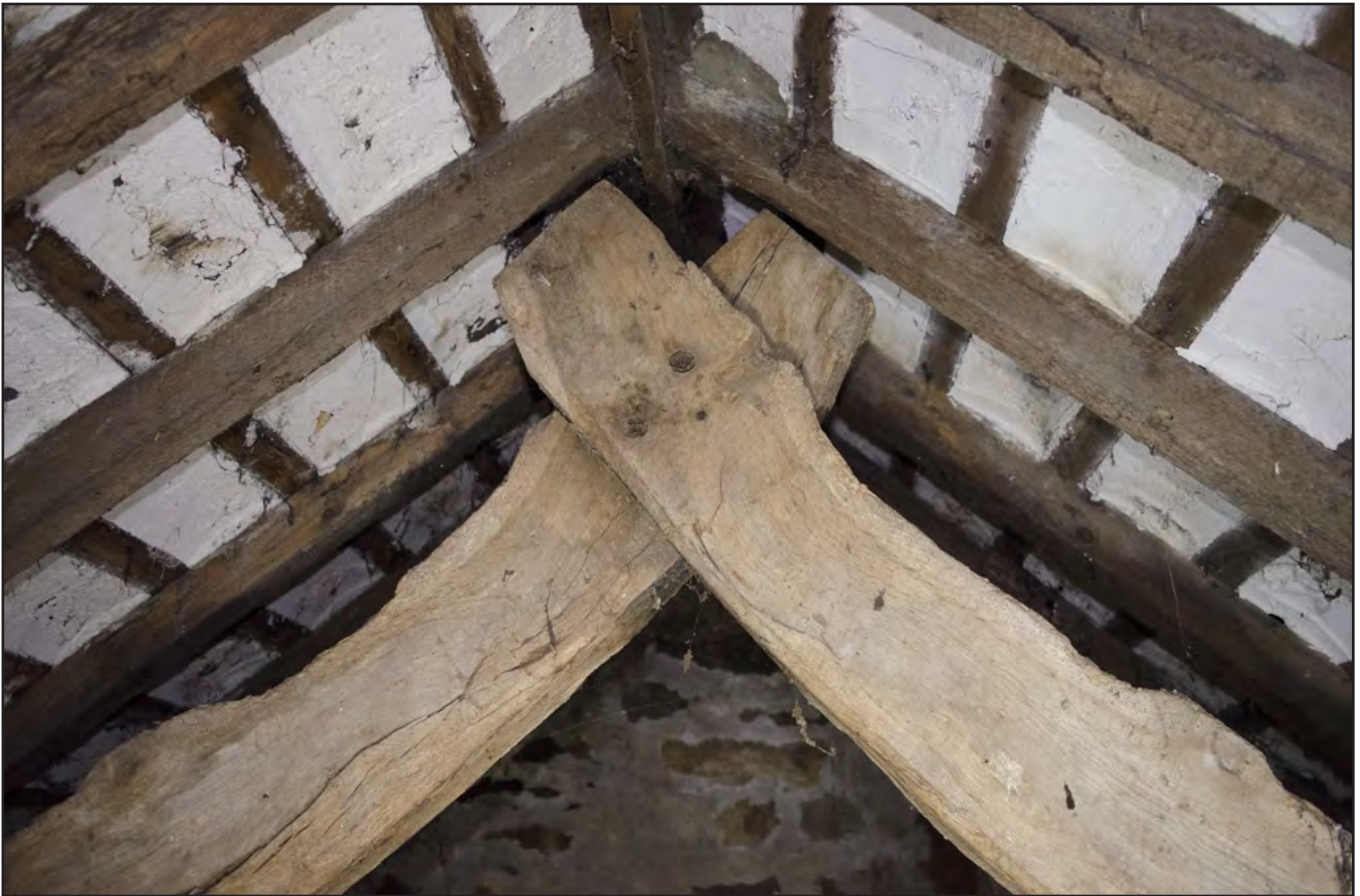
Plate 35: Store Room 3: detail of pegged apex on A-Frame Truss (a); scale: not used (archive reference: G2586_049).
