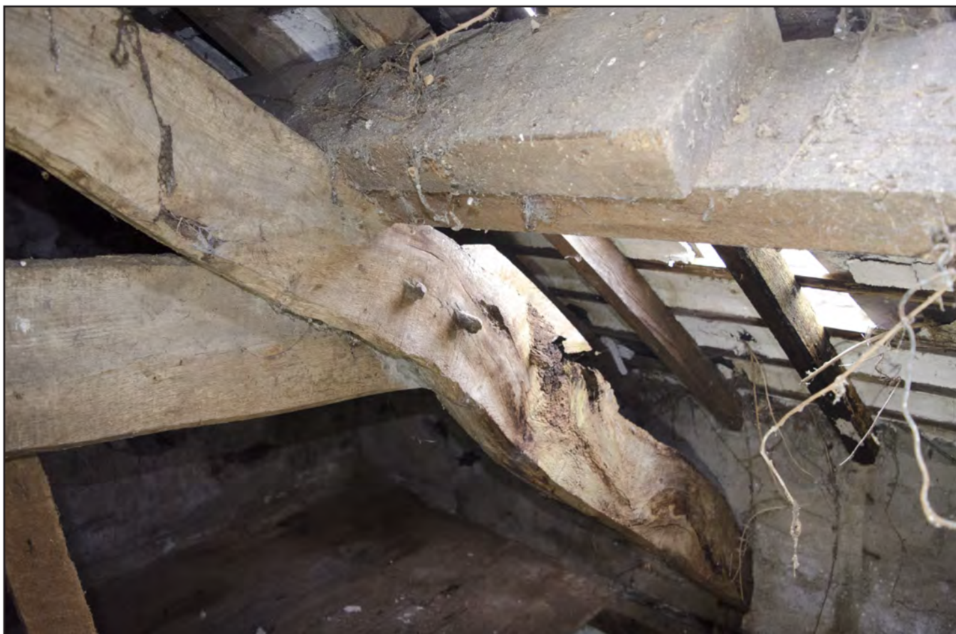
Plate 38: Store Room 3: detail of pegging apex on A-Frame Truss (a); scale: not used (archive reference: G2586_051).
