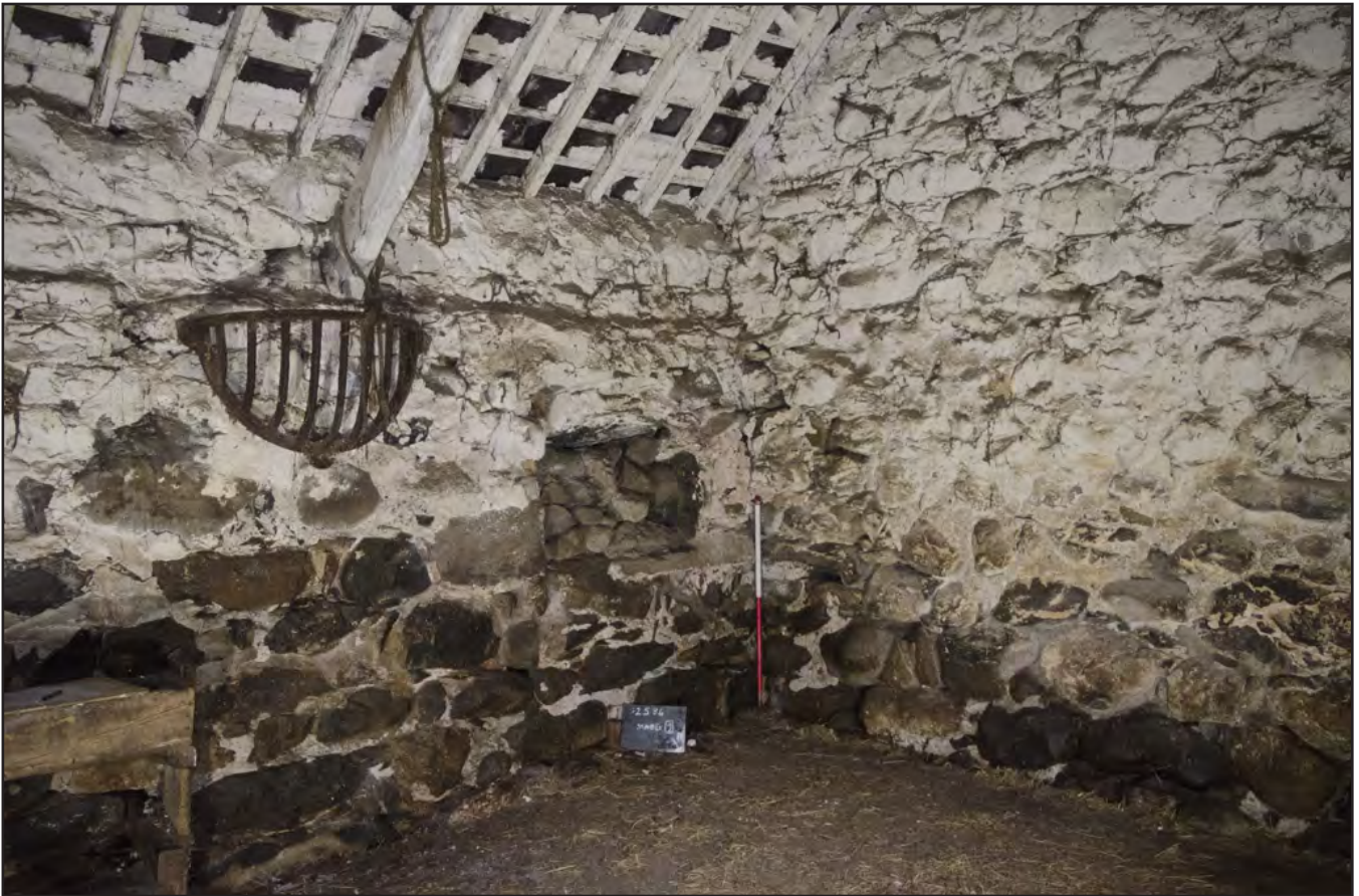
Plate 21: Stable 2: detail of southeast wall from doorway along with blocked window and manger; scale: 1x1m (archive reference: G2586_032).
