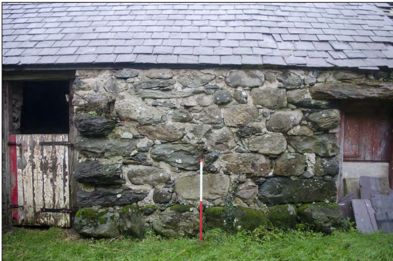
Plate 9: Southwest facing elevation: large block construction wall with two doorways at rear of building; scale: 1x1m (archive reference: G2586_011).
