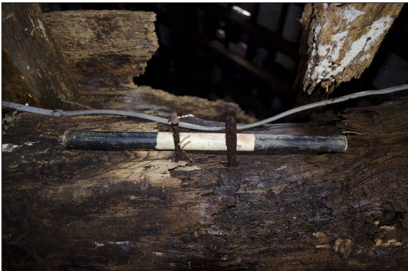
Plate 18: Store Room 1: detail of blacksmith nails within beam; scale: 1x0.3m (archive reference: G2586_028).
