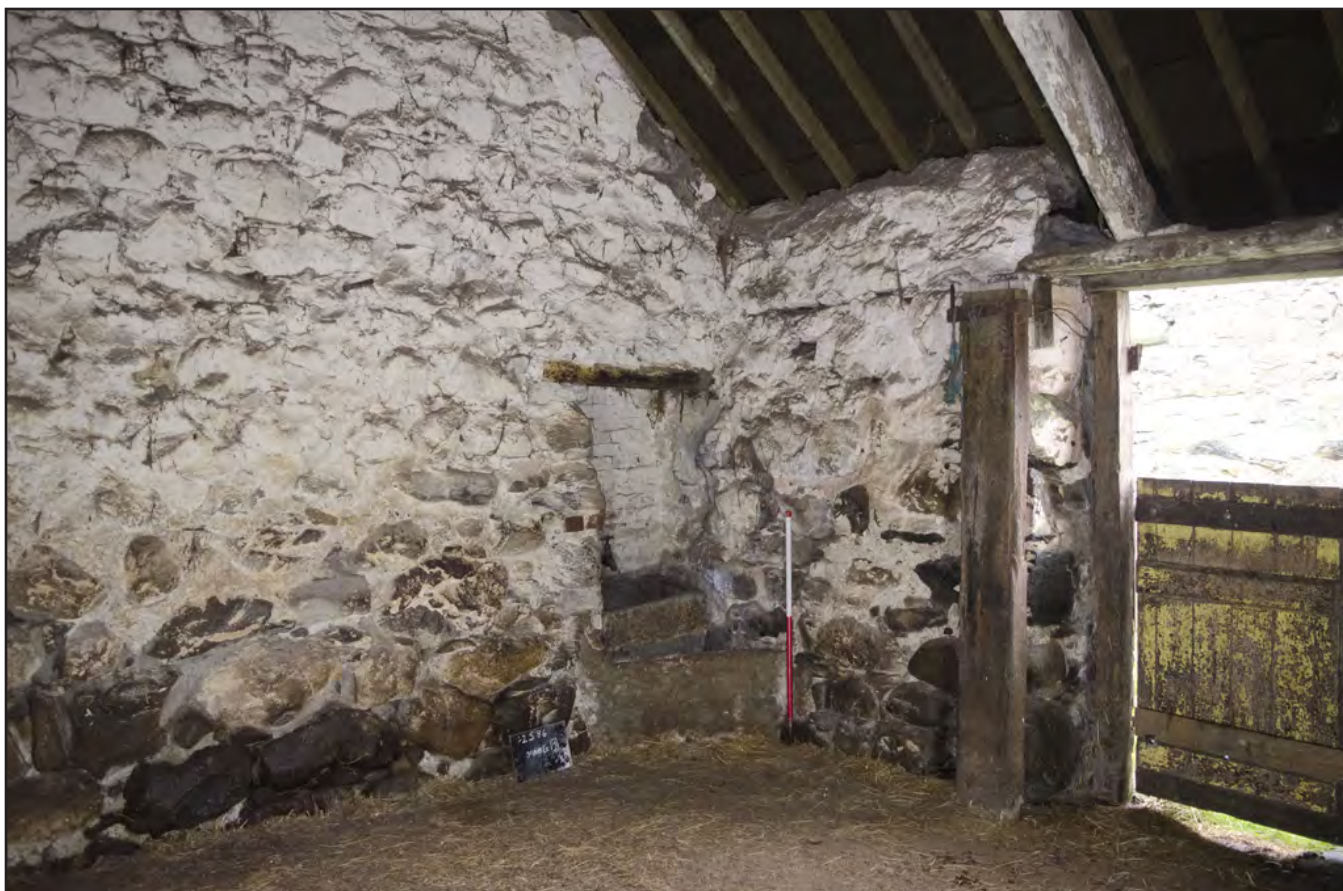
Plate 20: Stable 2: detail of western corner showing blocked doorway; scale: 1x1m (archive reference: G2586_030).
