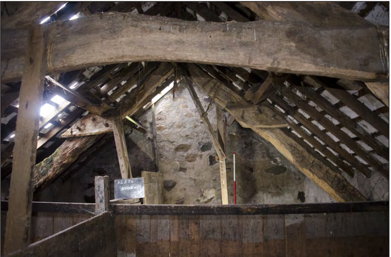
Plate 32: Store Room 3: detail of A-Frame Truss (b); scale: 1x1m (archive reference: G2586_045).
