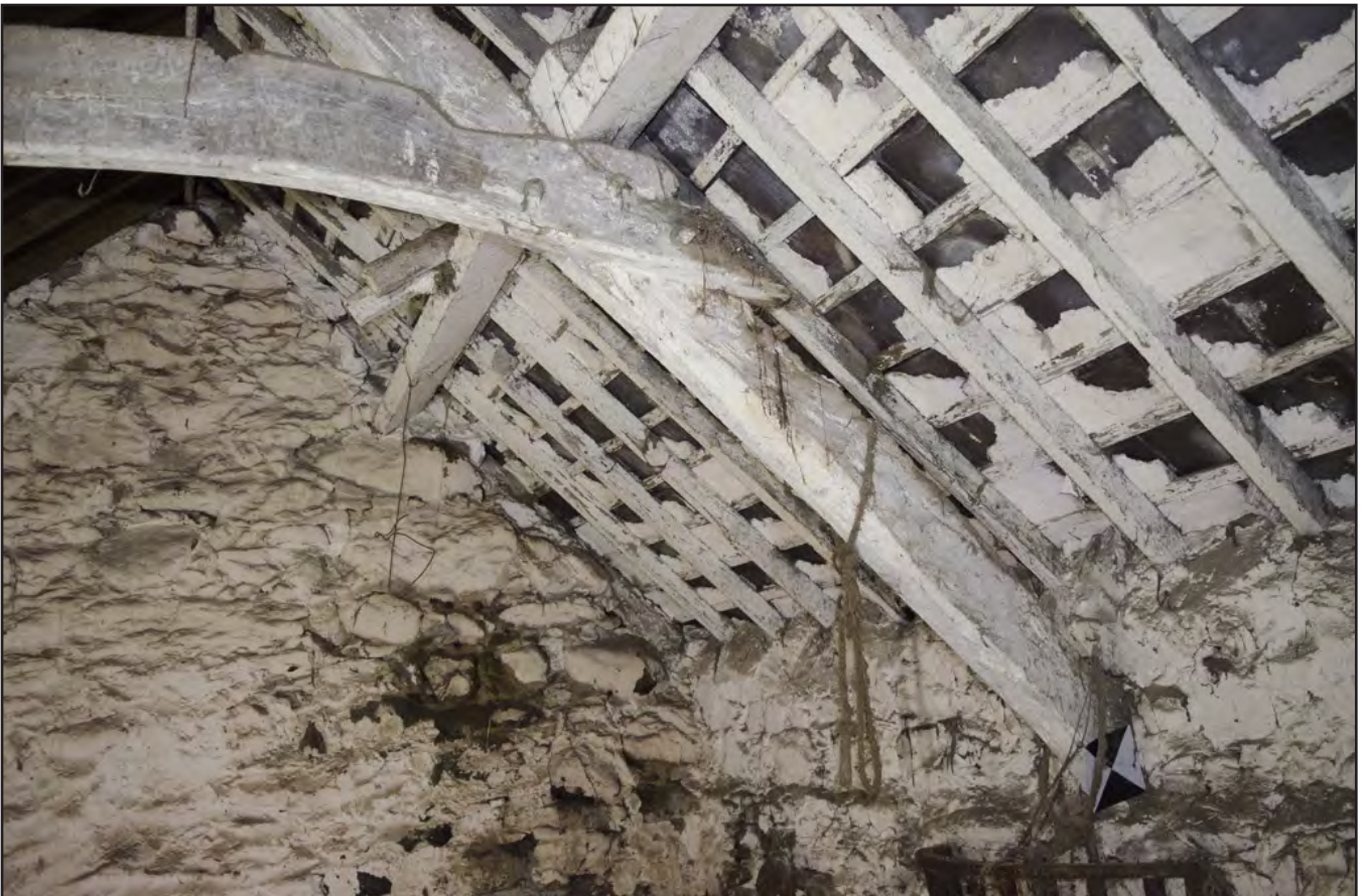
Plate 28: Stable 2: detail of A-Frame Truss from southwest wall; scale: not used (archive reference: G2586_039).
