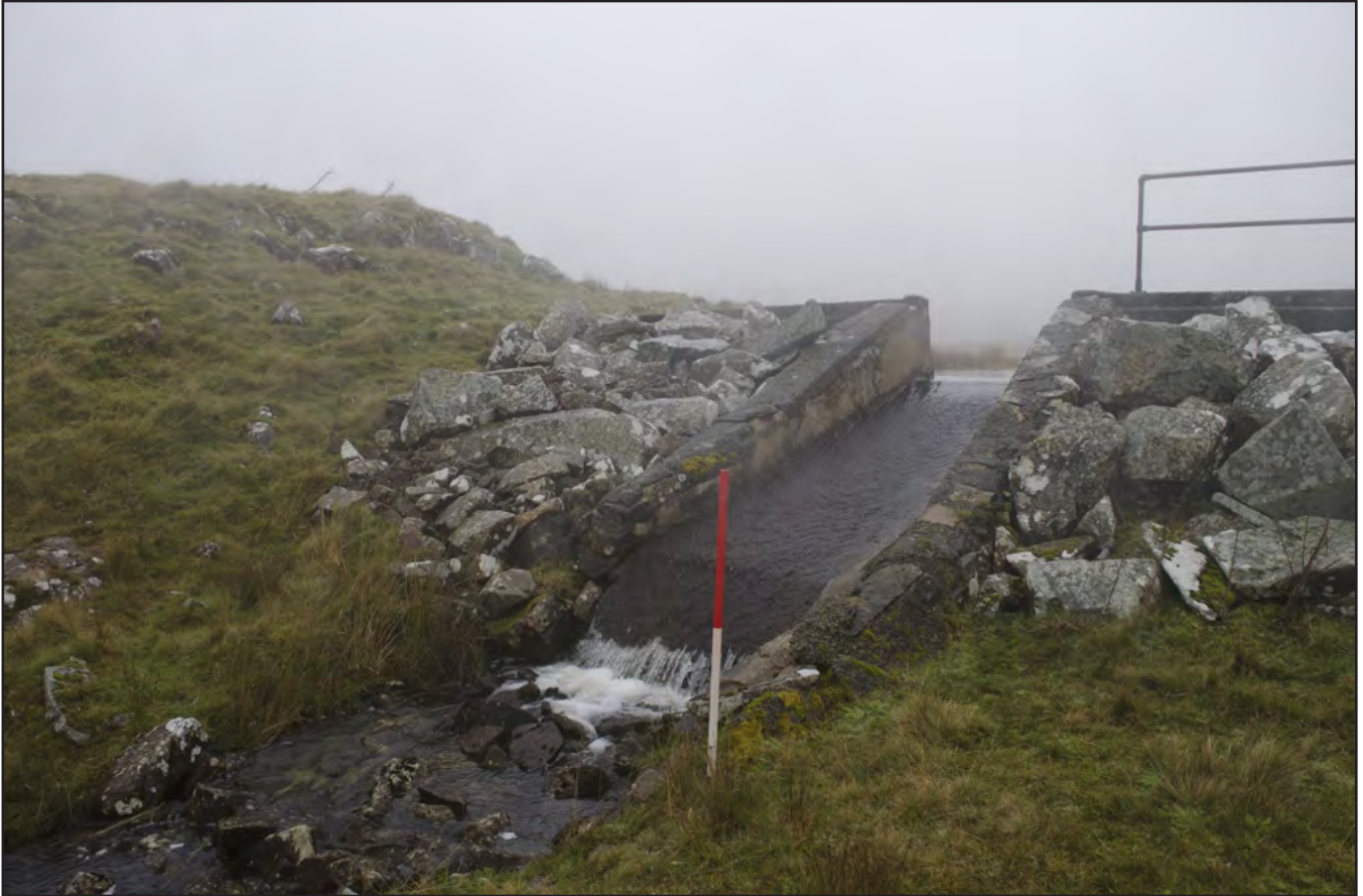
Plate 3: View of weir in dam wall; scale: 1x1m (archive reference: G2579_003).
