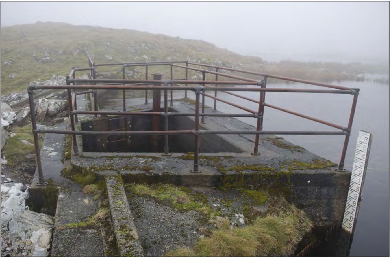
Plate 5: Detailed view of central inspection chamber structure; scale: not used (archive reference: G2579_006).
