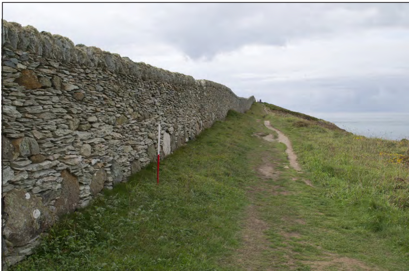
Plate 13: 2m high drystone walling, made of small shale slabs with cock and hen capping; scale: 1 x 1m (archive reference: G2565_065).
