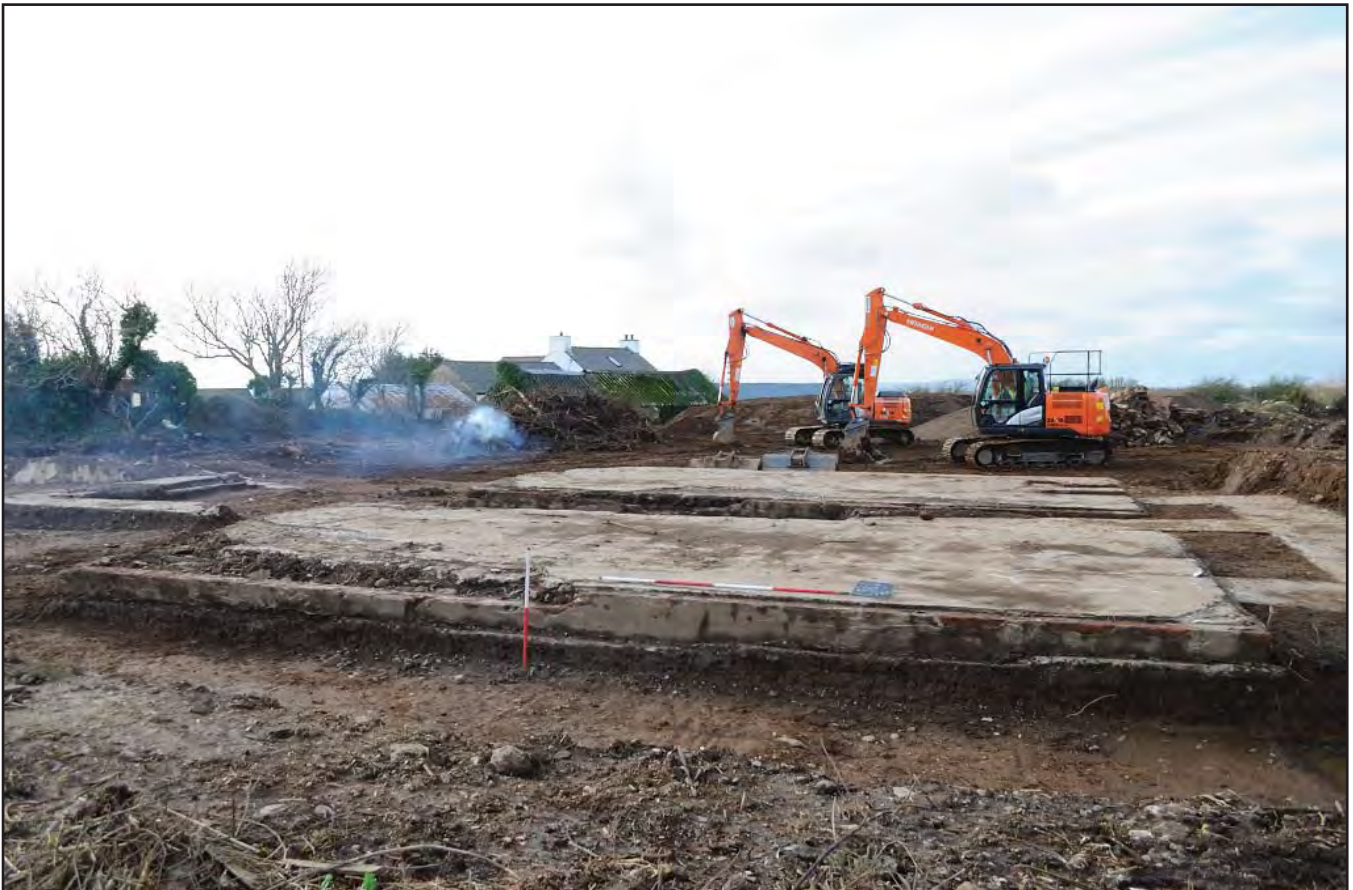
Plate 20: View of east side of platform base [07] showing cement render, concrete base and brick lining Scale 1x1m (archive reference: G2543_086)
