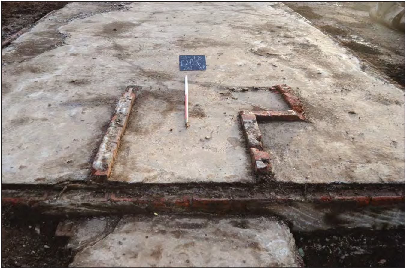
Plate 23: Brick foundations set in concrete for porch [21], at entrance of Base [08] Scale 1x1m (archive reference: G2543_089)
