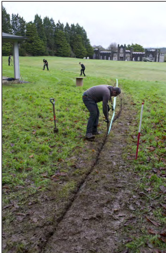
Plate 6: General shot from the east of pavilion, showing cable trench hand excavation in progress; scale: 1x1m (archive reference: G2542_016).
