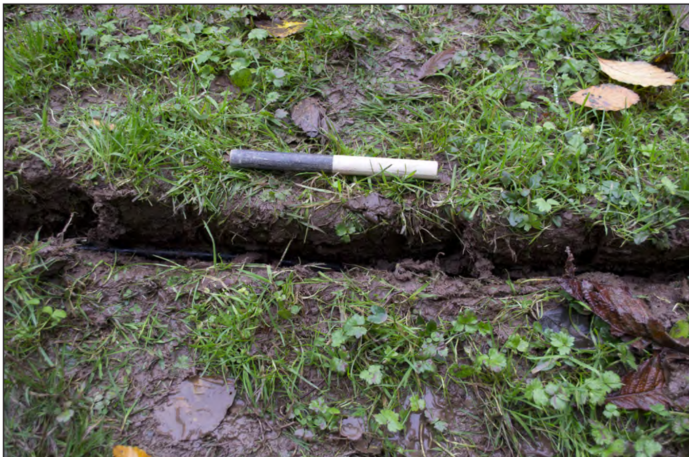
Plate 7: View of 'section' of cable trench through topsoil, with cable in place; scale: 1x0.2m (archive reference: G2542_015).
