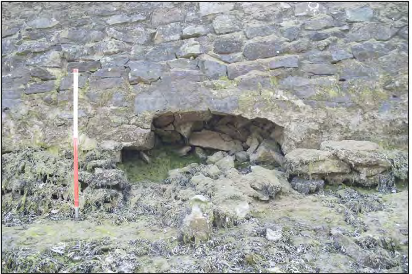
Plate 23: Collapsed part of wall, possibly a culvert, to the north of the bowling green, viewed from the NNE (scale: 1x1m, archive image ref G2527_019).
