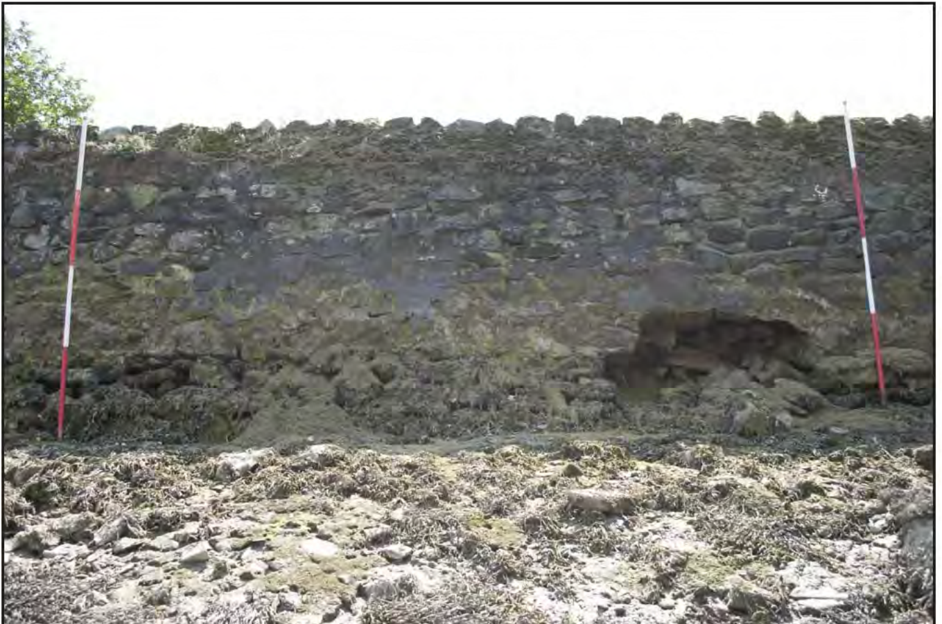
Plate 08: Pre-commencement photographic survey of section of retaining wall to be repaired, perpendicular shot 2 of 13, viewed from the NNE (scales: 2x2m (spaced at 5m), archive image ref G2527_002).
