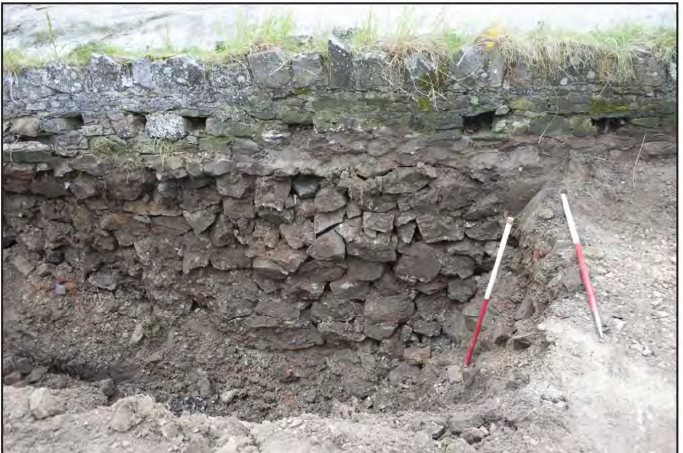
Plate 24: Revetment wall [001] showing the larger stones towards the bottom of the wall, viewed from the S (scales 2x1m, archive image ref G2527_031).
