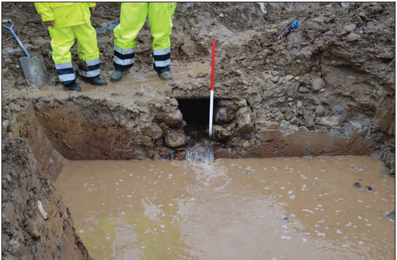
Plate 08: Slate topped culvert [007] in Field 6. View from N. Scale 1x1m. (G2424_WB_2017_067).
