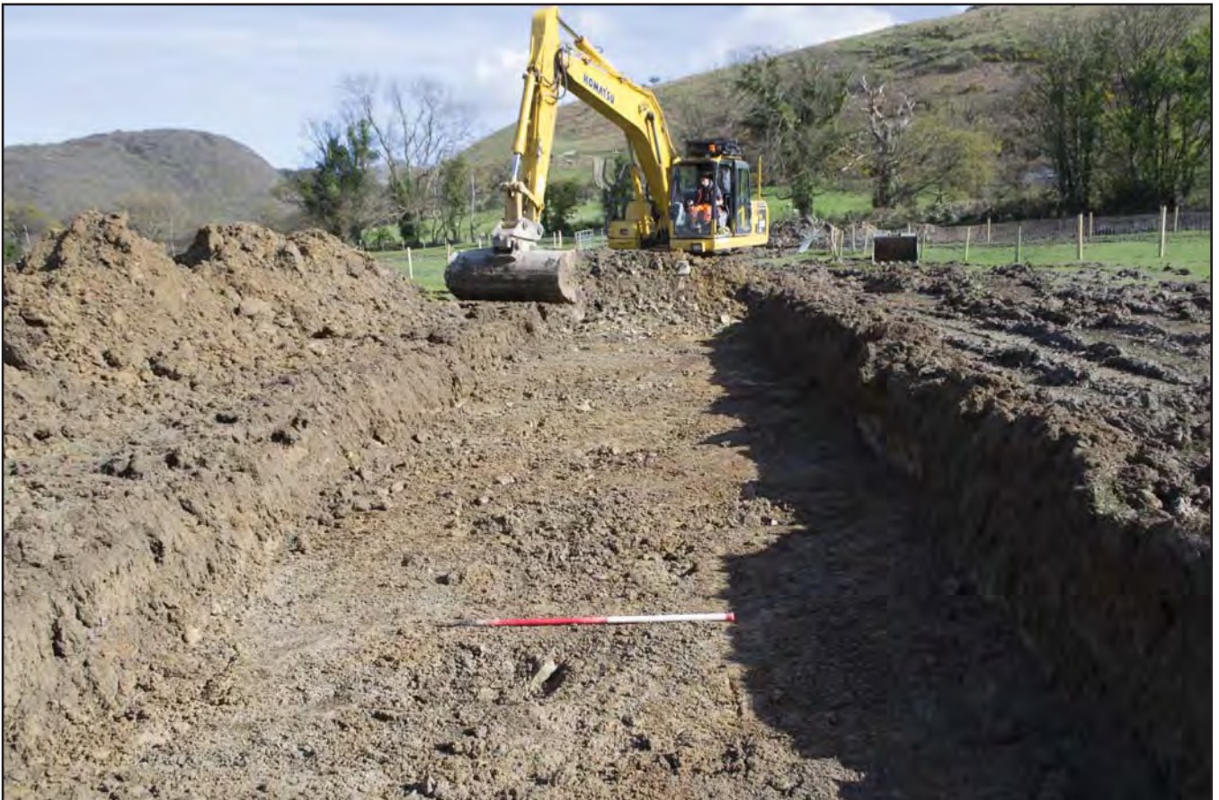
Plate 26: Strip in advance of 450mm pipe in Field 1. View from NW. Scale 1x1m (G2424_WB_2017_044).
