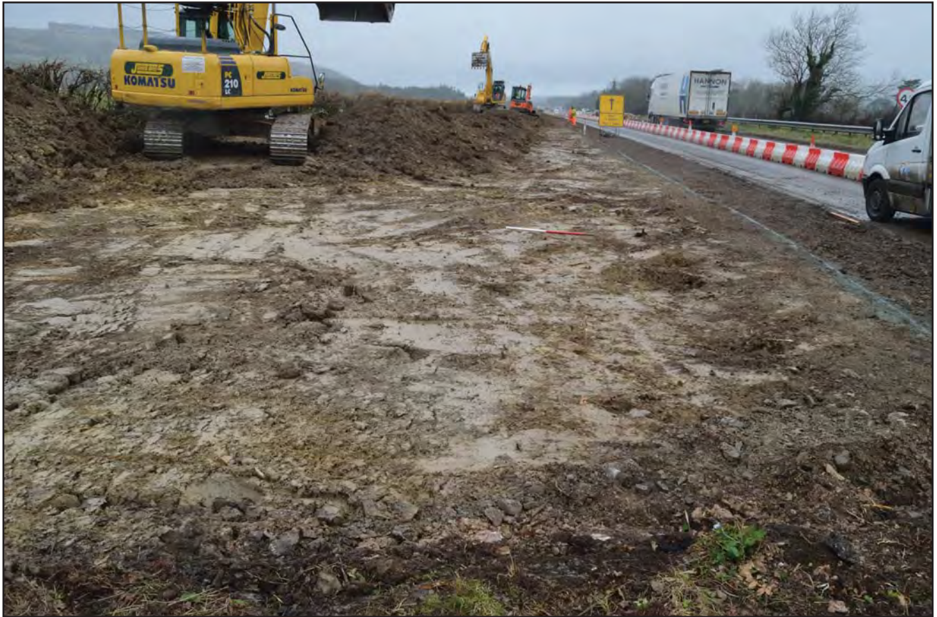
Plate 21: Strip to natural for merge taper. View from NE. Scale 1x1m. (G2424_WB_2017_019).
