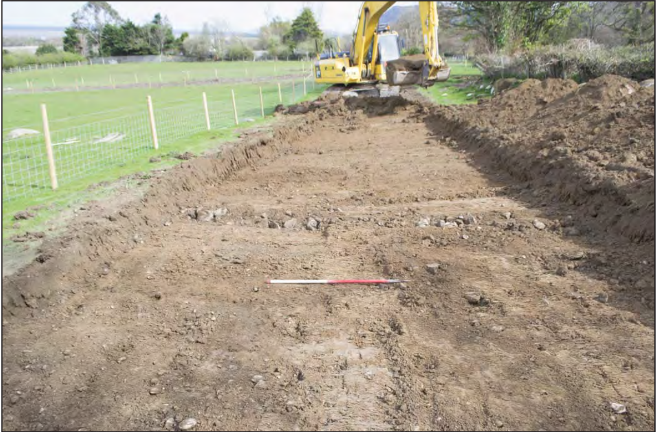
Plate 25: Topsoil strip for access road in Field 1. View from S. Scale 1x1m (G2424_WB_2017_035).
