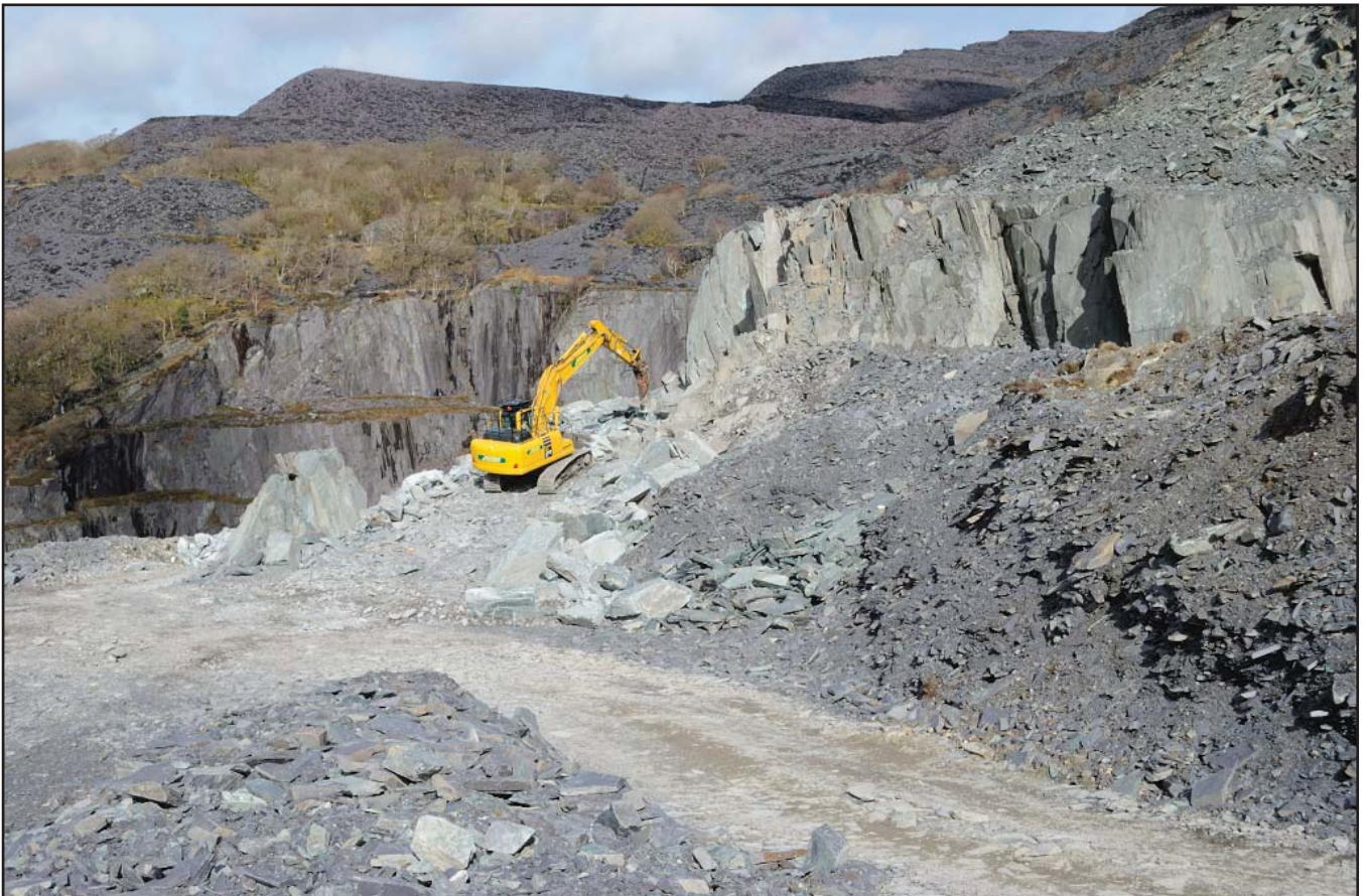
Plate 20: Breaking up boulders from unstable rock face of the 'Cockerel'. View from the south (Photographic archive ref. G2486_065).
