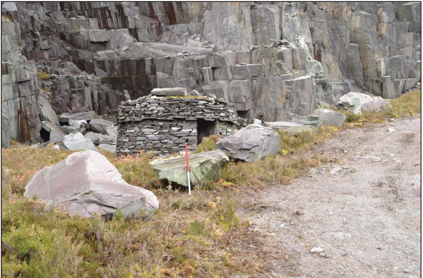
Plate 28: Slate boulders to protect the circular blast shelter. Scale 1.0m. View from the west (Photographic archive ref. G2486_057).
