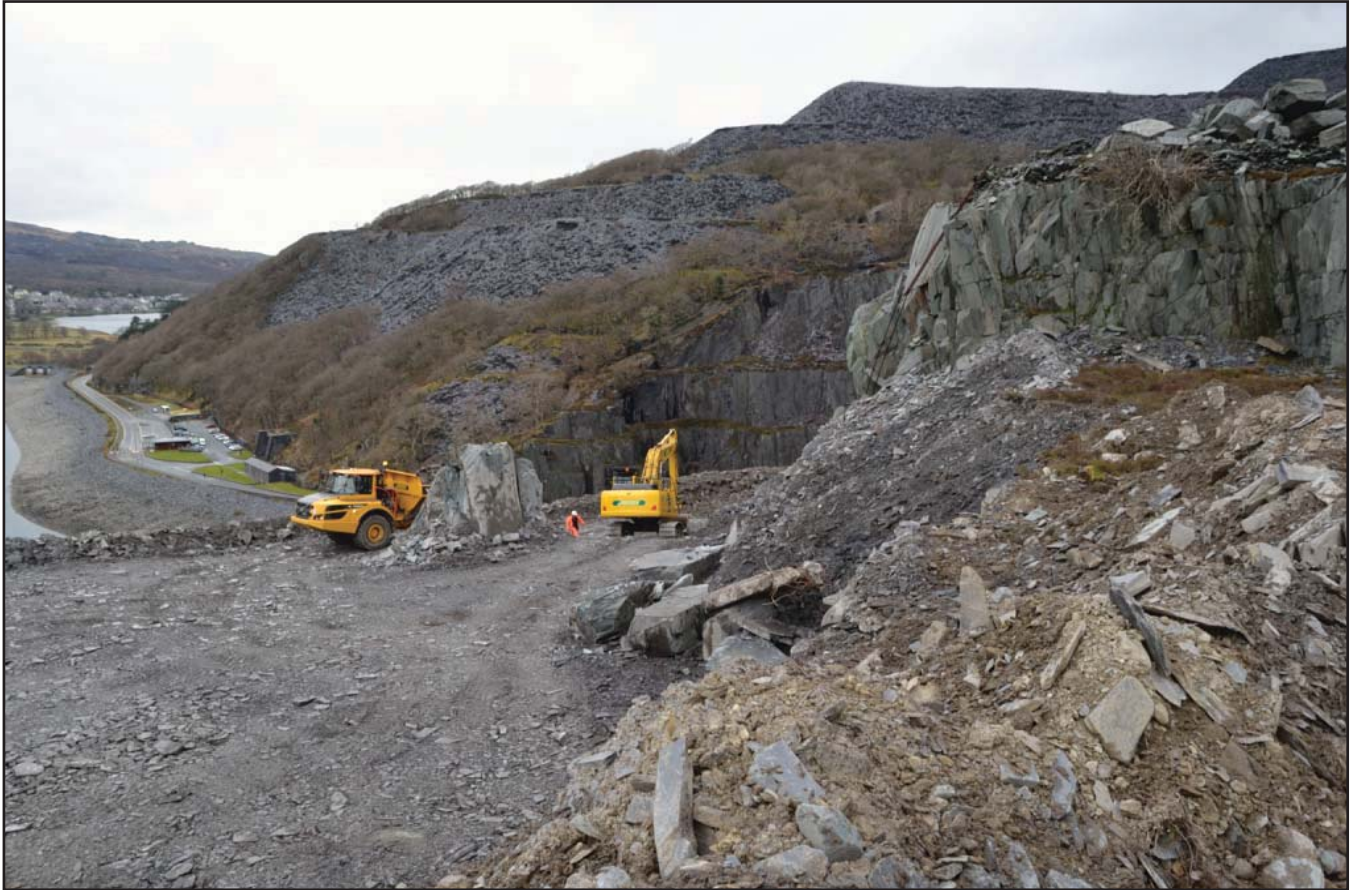
Plate 17: Catchment area and bunds below the 'Cockerel'. View from the southeast (Photographic archive ref. G2486_059).
