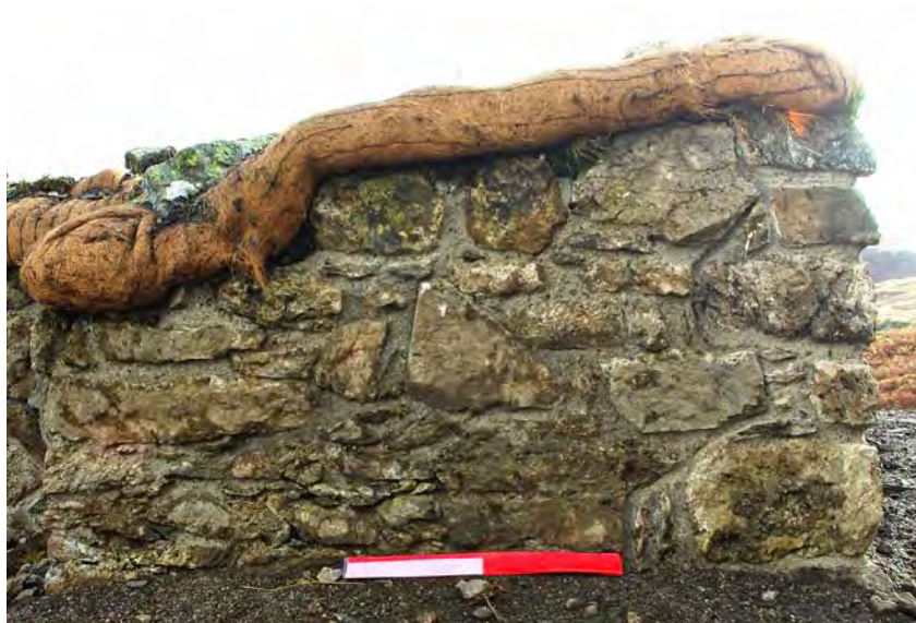
Fig. 42 Wall 517, E facing, after conservation. Curtain wall thickening
