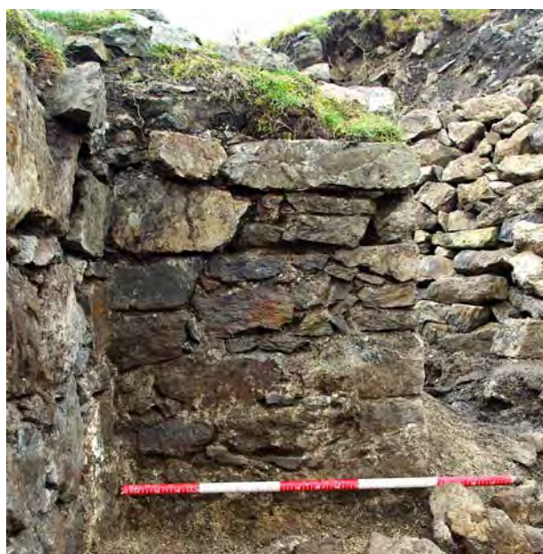
Fig. 39 Wall 517, E facing, before conservation. Curtain wall thickening
