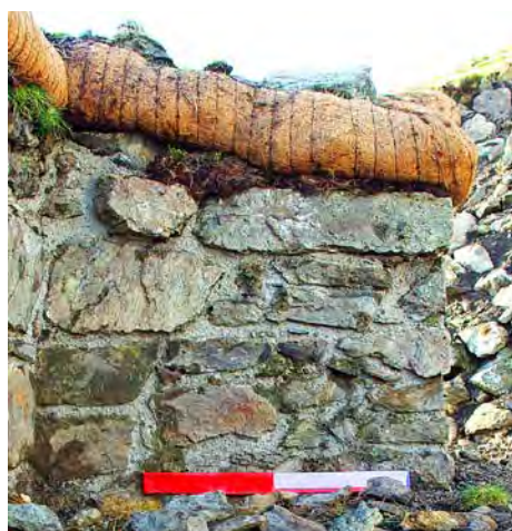
Fig. 40 Wall 517, E facing, after conservation. Curtain wall thickening
