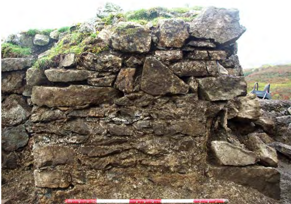
Fig. 41 Wall 517, E facing, before conservation. Curtain wall thickening
