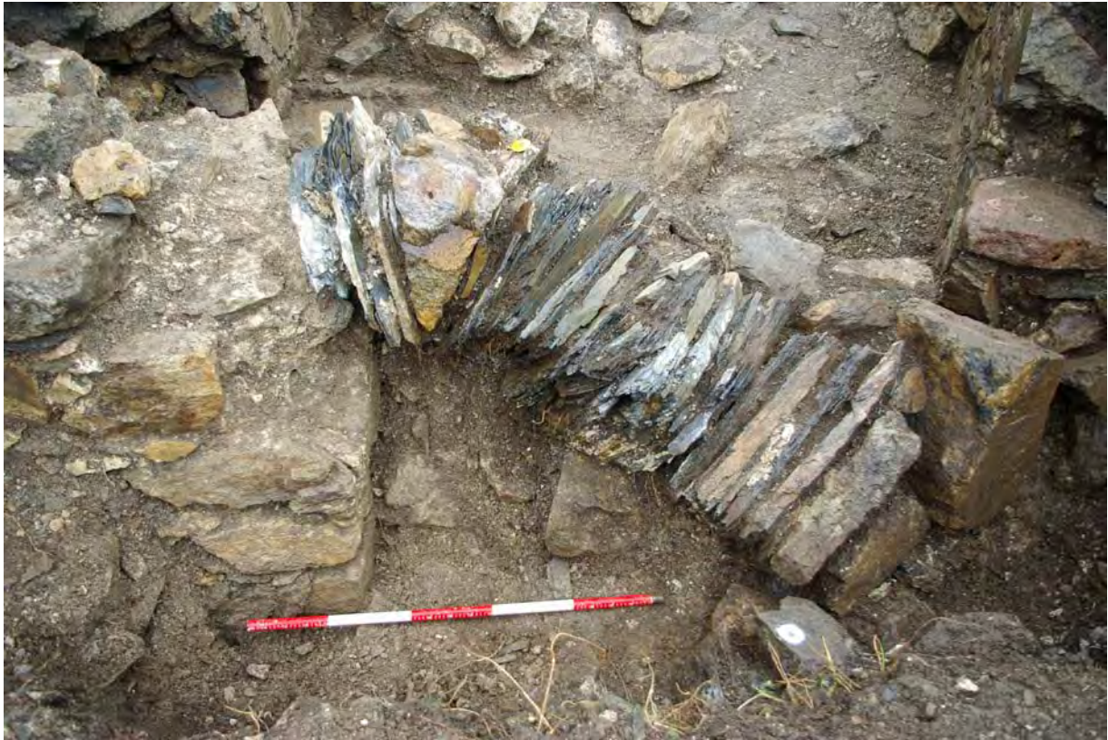
Fig. 17 Semi-collapsed arch (526)
