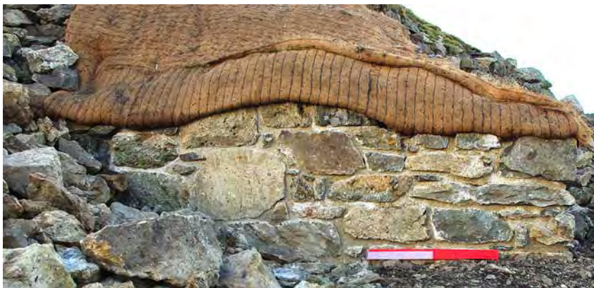
Fig. 48 Wall 529 after conservation. Outer face curtain wall. No original facing visible at this level
