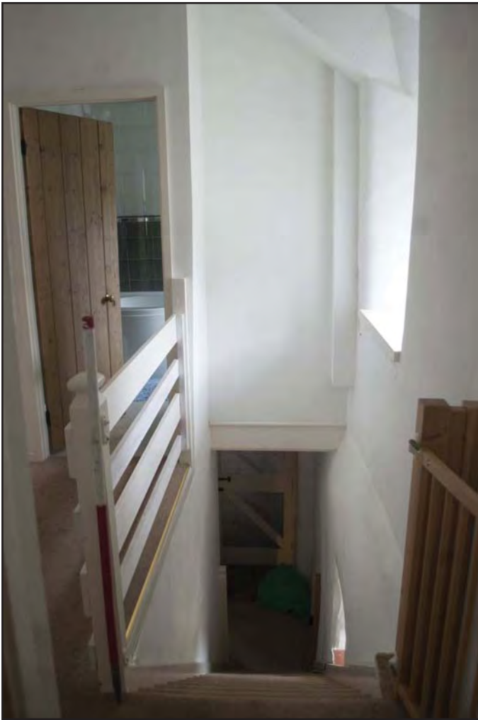
Plate 37: View of stairwell showing ground floor elevation against first floor expansion on north facing wall, with view of early 20th century staircase fittings (photographic archive ref. G2520_094)
