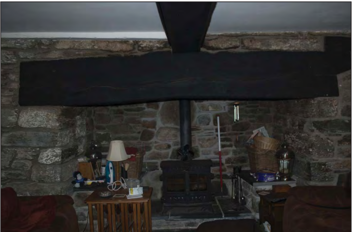
Plate 18: View of late 16th century fire range F02 within Lounge 1, with visible peg holes within the lintel (photographic archive ref. G2520_35)
