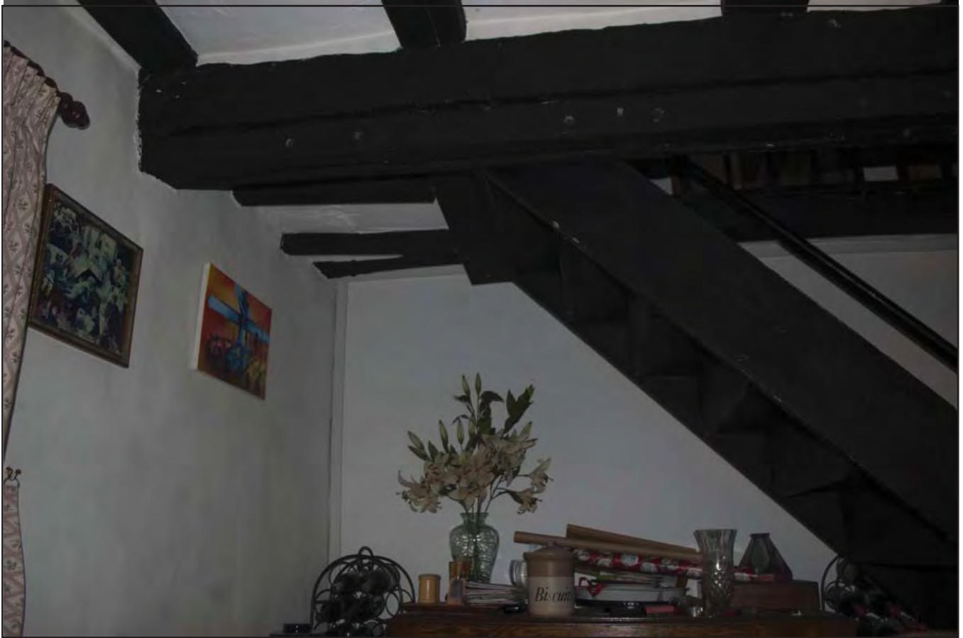
Plate 21: View of earlier narrow beams on a eastern-western beams, alongside visible peg holes within the central beam (photographic archive ref. G2520_044)
