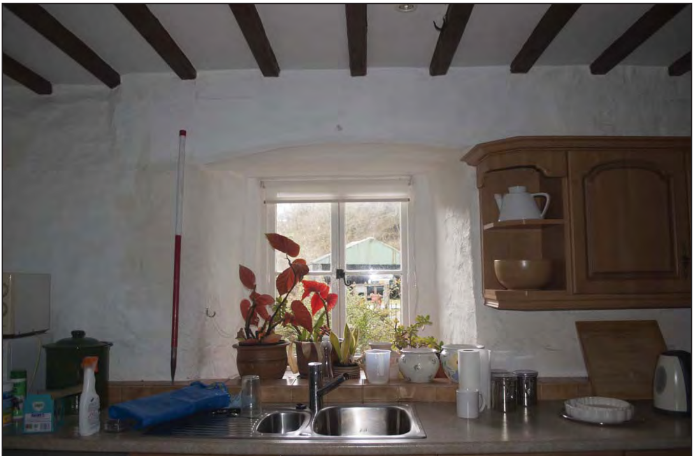
Plate 36: View of window W06 displaying arched lintel, previously belonging to the main entrance of the 17th century cross-passage (photographic archive ref G2520_080)
