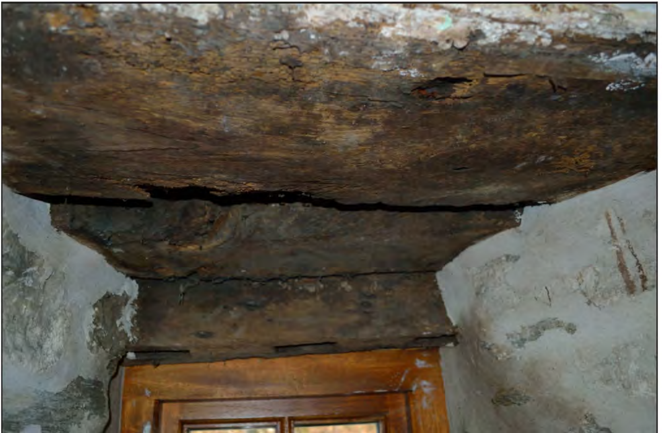
Plate 57: Detail of WB02, showing the three lintel beams, with outermost one with three mortice holes (10cm x 3cm) cut into it (archive reference: G2520_1126).
