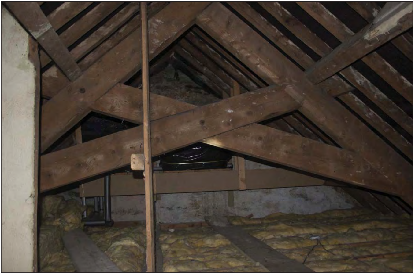
Plate 41: View of 20th century replacement timber roof truss in House 1 (photographic archive ref. G2520_052)
