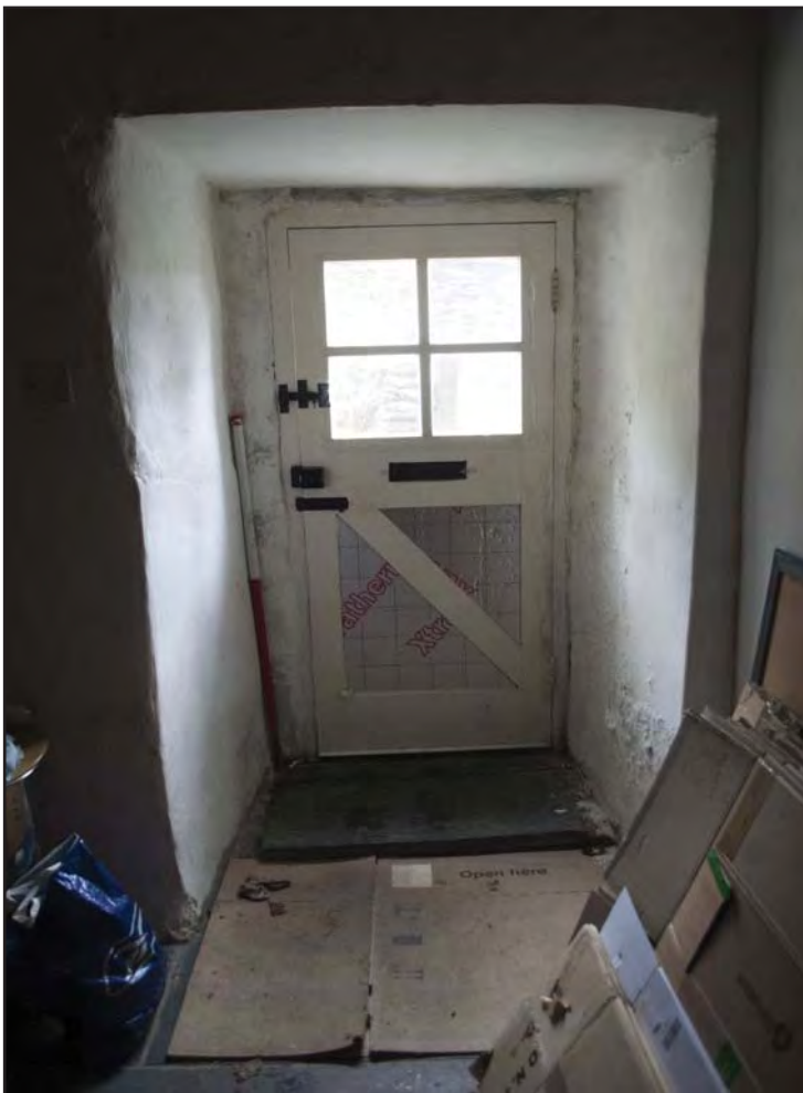
Plate 30: View of doorway D01, the northern end of the 17th century cross-passage, with 1930s half glass paneled door (photographic archive ref. G2520_068)
