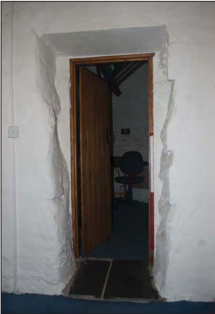
Plate 27: View of doorway D16 cut into the former northern gable end after further 18th century extension (photographic archive ref. G2520_066)
