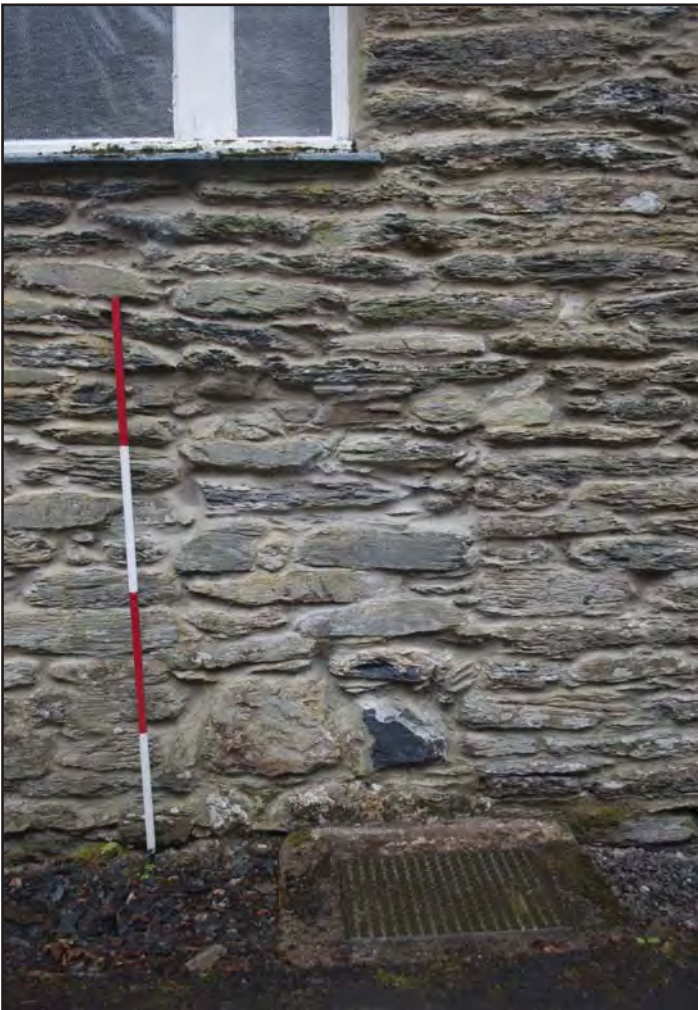
Plate 10: View of visible blocked doorway DB01 below window W13, may have possibly been part of the late 16th century cross-passage (photographic archive ref. G2520_018)
