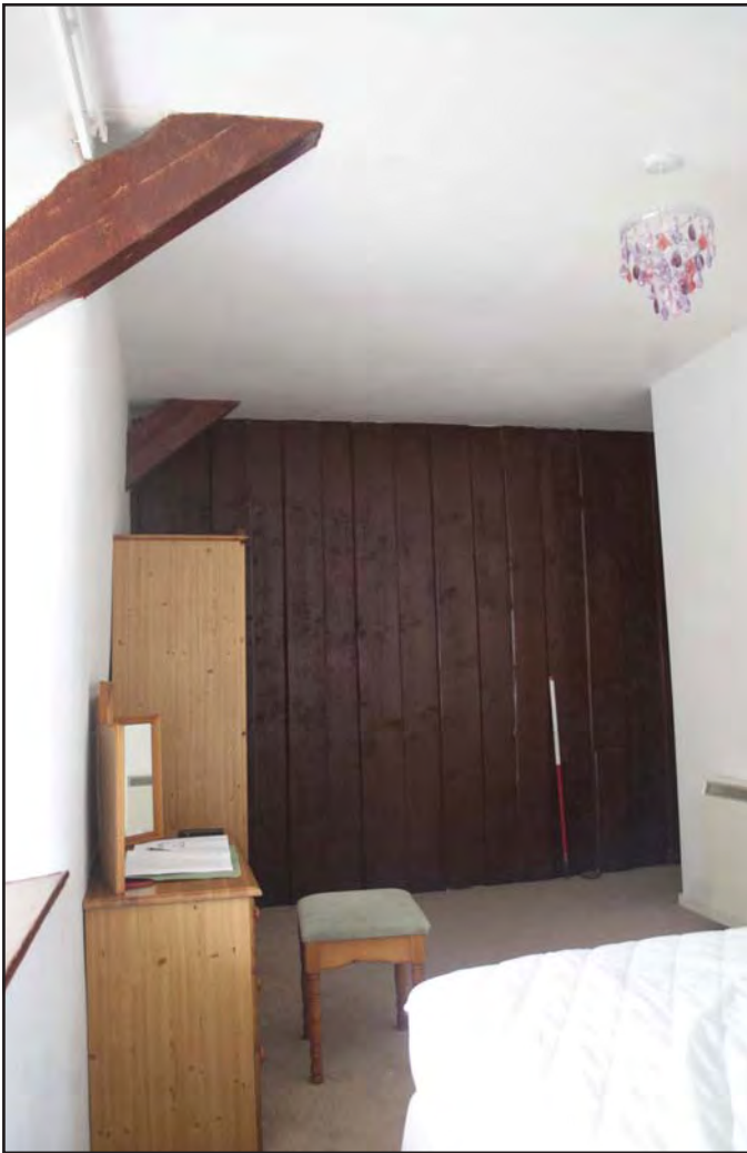
Plate 39: View of Bedroom 7 with exposed braces and early 20th century partitioning wall (photographic archive ref. G2520_092)
