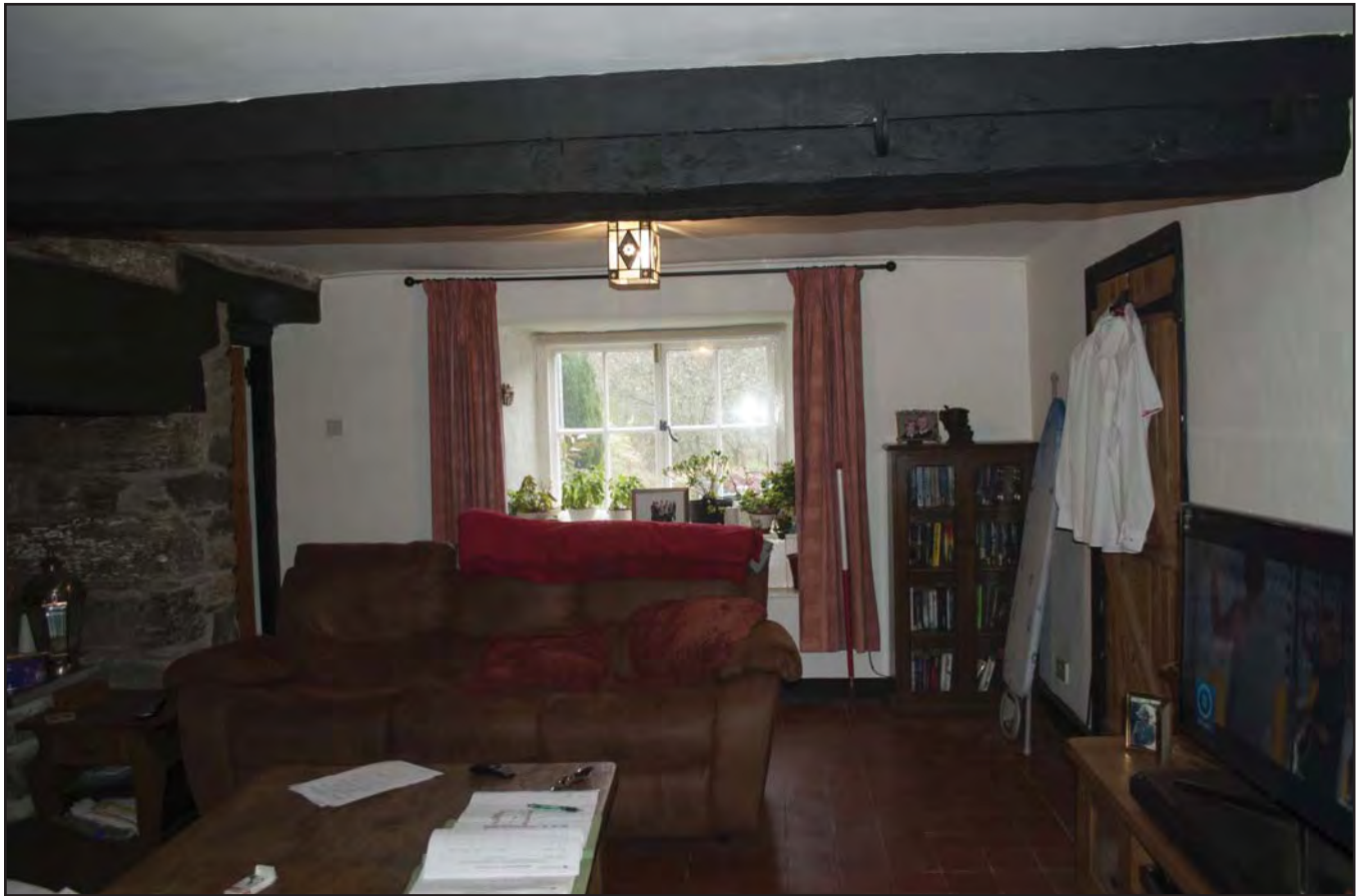
Plate 19: View of central beam running across a North - South axis in Lunge 1, with meat hooks visible the west face (photographic archive ref. G2520_036)
