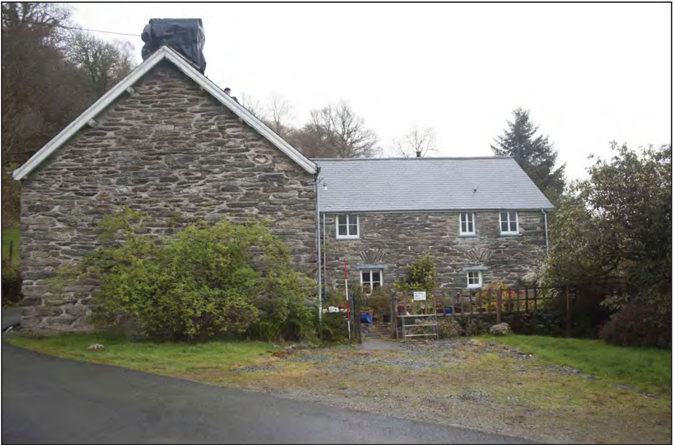
Plate 05: View of House 1 south gable end, with visible evidence of roof raising. Alongside with the view of House 2 the southern elevation (photographic archive ref. G2520_009)
