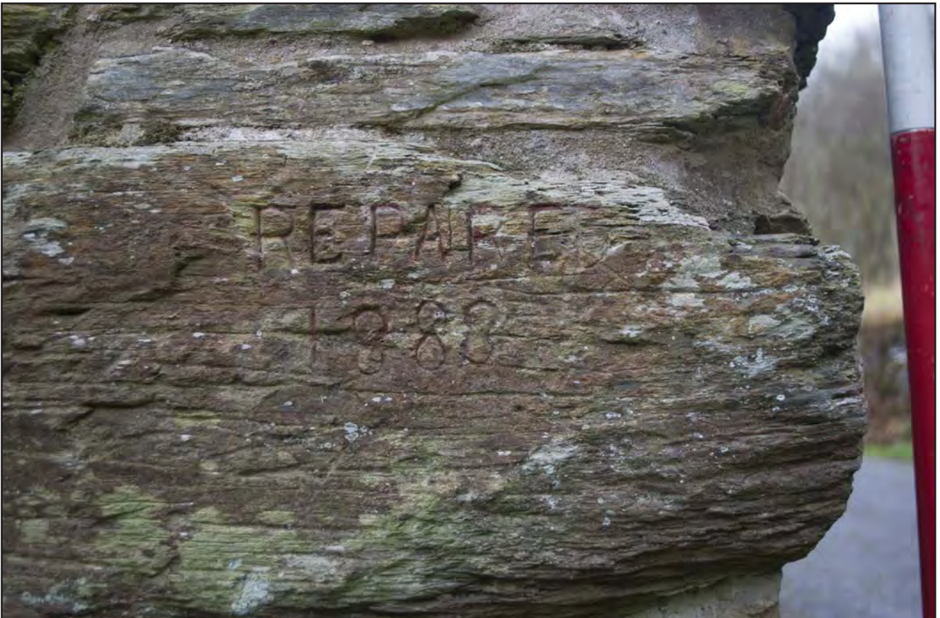
Plate 12: Close-up view of "REPAIRED 1883" engraved into the north facing quoin of House 1 north gable end (photographic archive ref. G2520_007)
