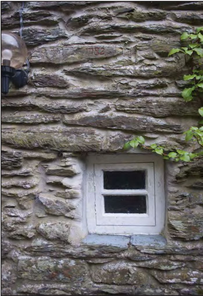
Plate 15: View of window W10 on western elevation demonstrating a later window size reduction, alongside with dates 1782 engraved into a stone above, with visible remnants of red Ox-blood paint (photographic archive ref. G2520_017)
