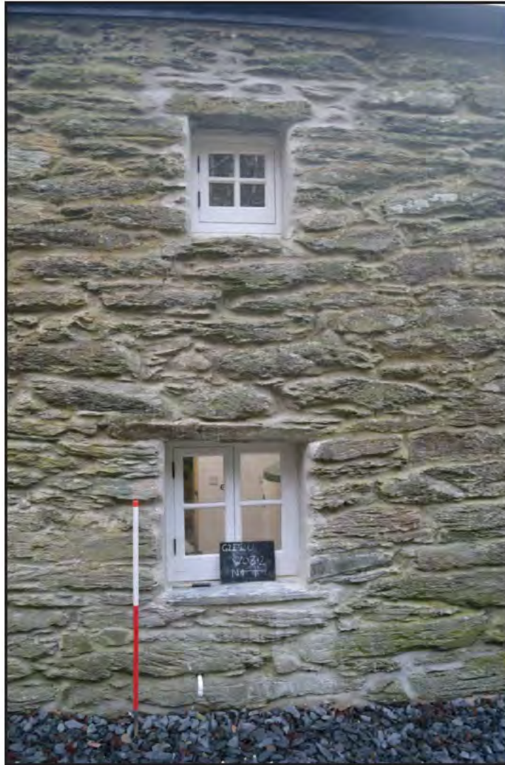
Plate 52: Detail of replacement windows WB02 and W03; scale: 1x1m (archive reference: G2520_1113).
