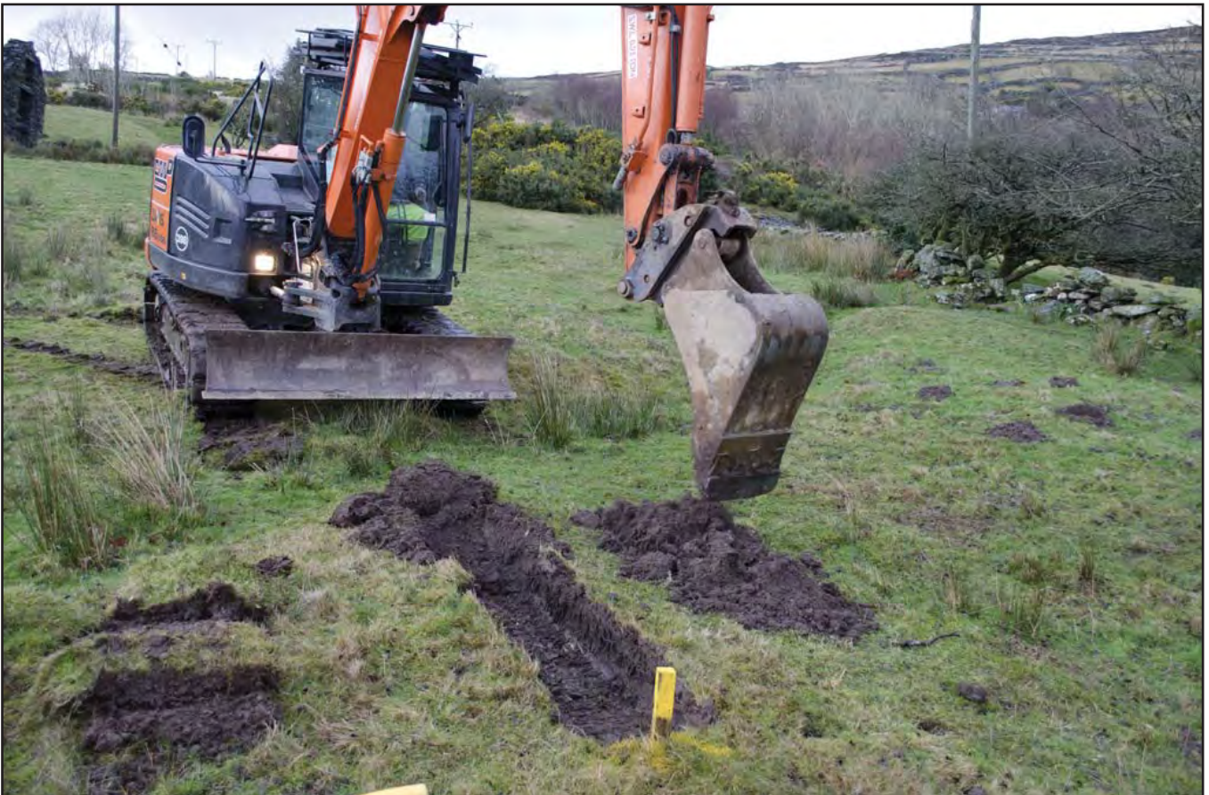
Plate 02: Trial Hole 1 - working shot of Trial hole 1 during excavation and removal of topsoil (archive image: G2492_016)
