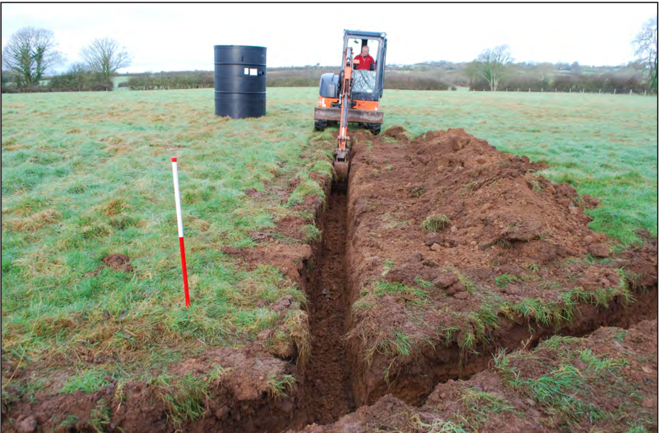
Plate 10: View from the northwest during the excavation of the soakaway trench. Note the septic tank positioned near the excavator prior to installation; scale: 1.0m (archive image: G2494_020)
