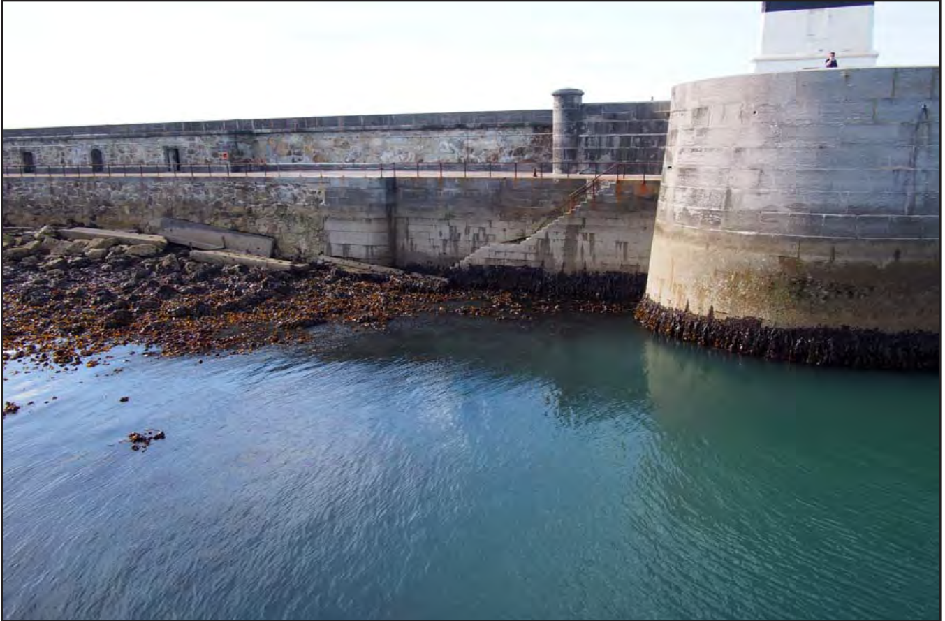
Plate 11: Portside view of the tail end of breakwater showing relationship with the ashlar masonry with view former storage and convenience area (sourced from Civil Engineering Solutions: 20150928 Holyhead Breakwater 151.jpg).
