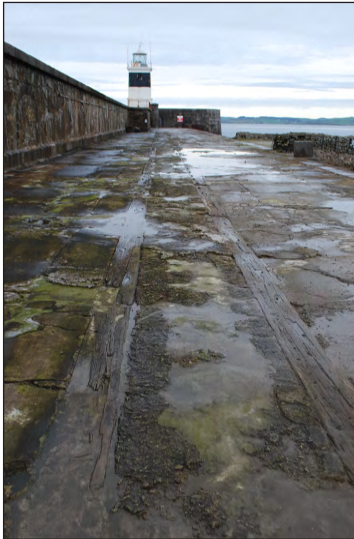
Plate 23: Holyhead Breakwater - view from west of wooden sleepers located along lower breakwater walkway near the lighthouse (archive image: G2498_022).
