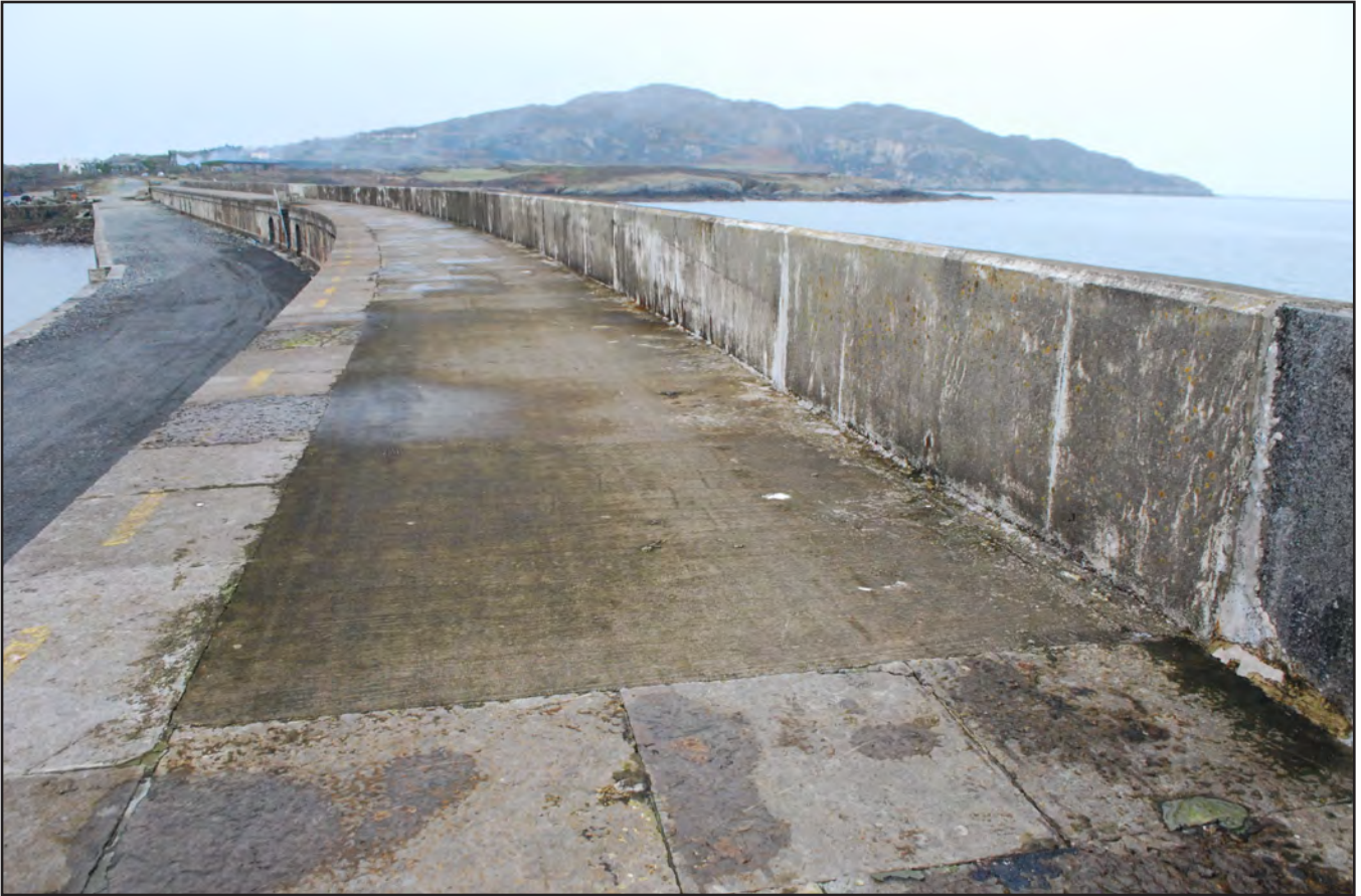
Plate 28: Holyhead Breakwater - view from east of storm damage repair to the parapet and carriageway (archive image: G2498_046).
