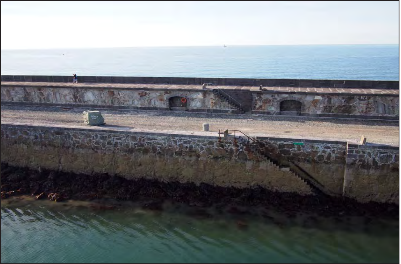
Plate 10: Portside view of mooring post, and staircases leading into the sea, and onto the parapet. Note two original alcoves with masoned seated areas possibly used for shelter during shipments (sourced from Civil Engineering Solutions: 20150928 Holyhead Breakwater 377.jpg).
