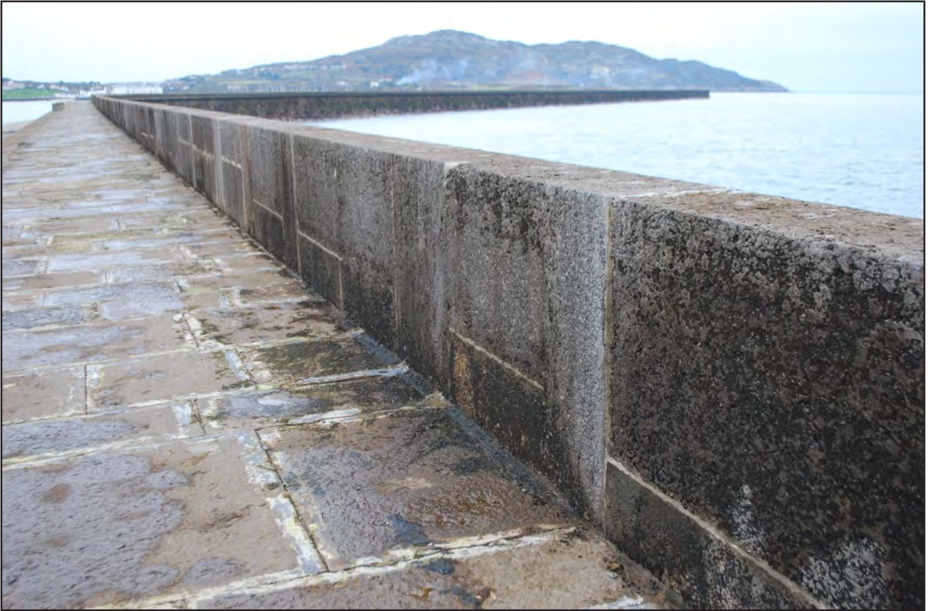
Plate 26: Holyhead Breakwater - view from southeast of parapet ashlar showing cyclopean blocks (archive image: G2498_037)
