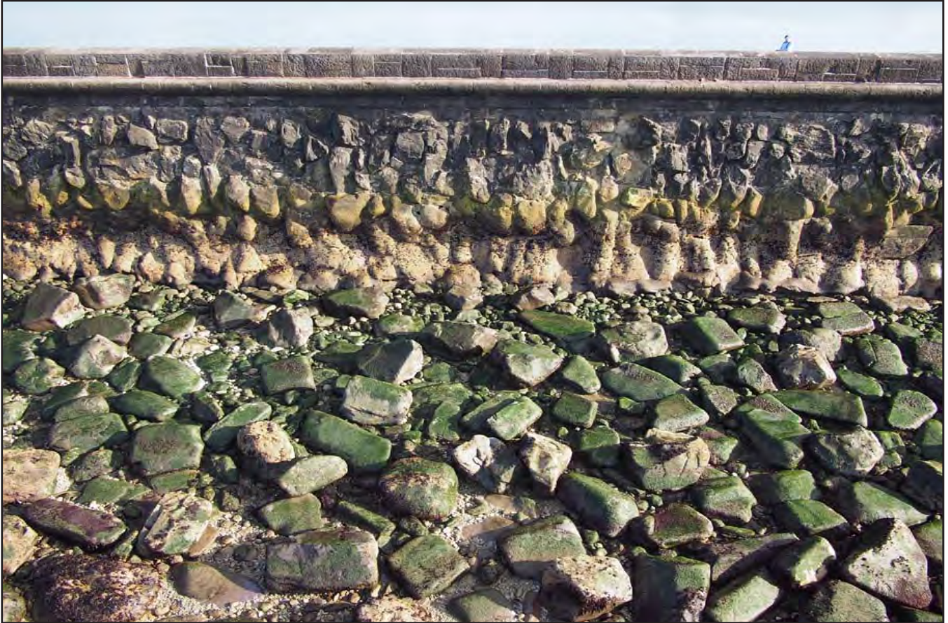
Plate 05: Seaward side view of rubble sourced from Holyhead Mountain used as supporting foundations of the parapet (sourced from Civil Engineering Solutions: 20150928 Holyhead Breakwater 186.jpg).
