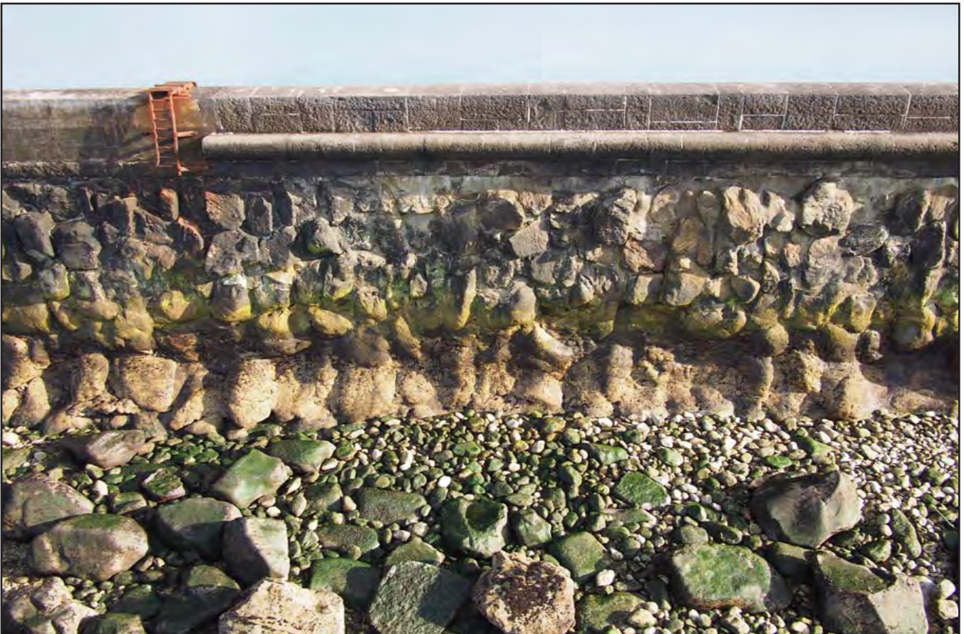
Plate 06: Seaward view of parapet with the remnants of a later addition of a ladder, possibly used in emergencies (sourced from Civil Engineering Solutions: 20150928 Holyhead Breakwater 206.jpg).
