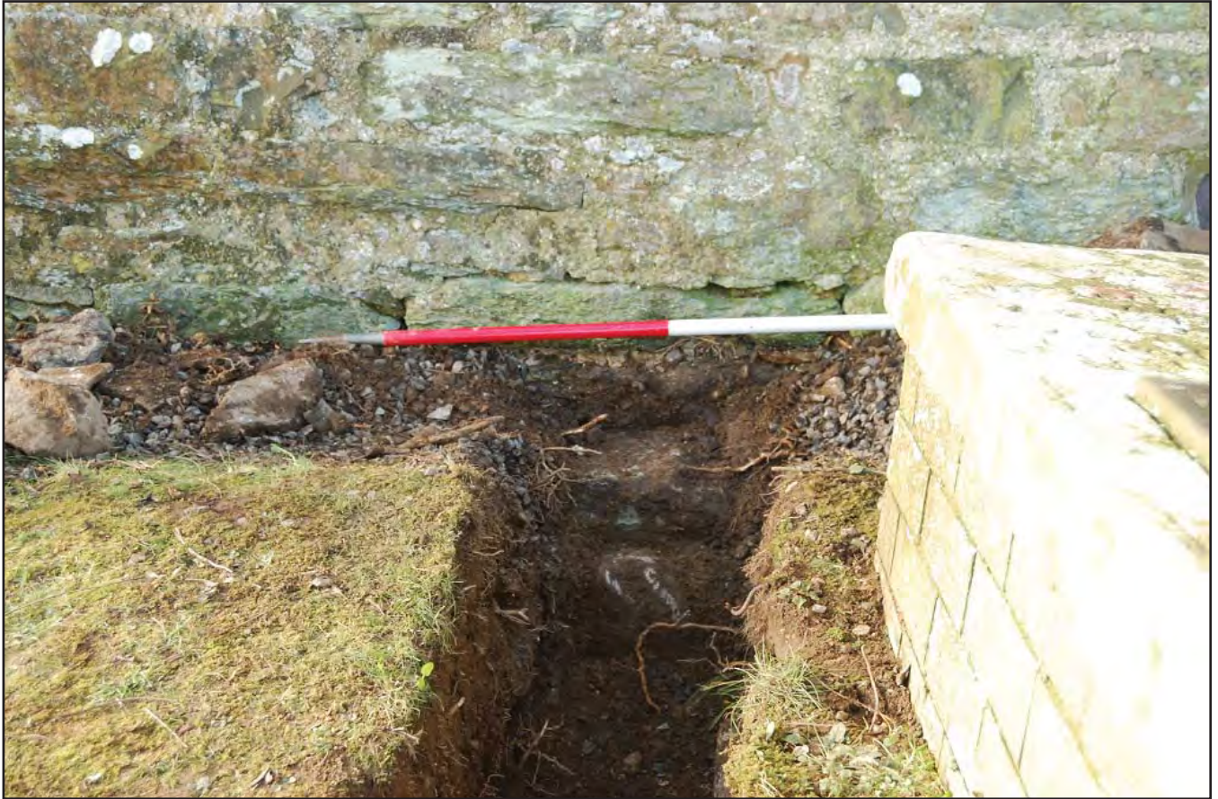
Plate 05: Footing of church wall exposed in the pipe trench. Scale 1m. (photographic archive ref. G2488_009).
