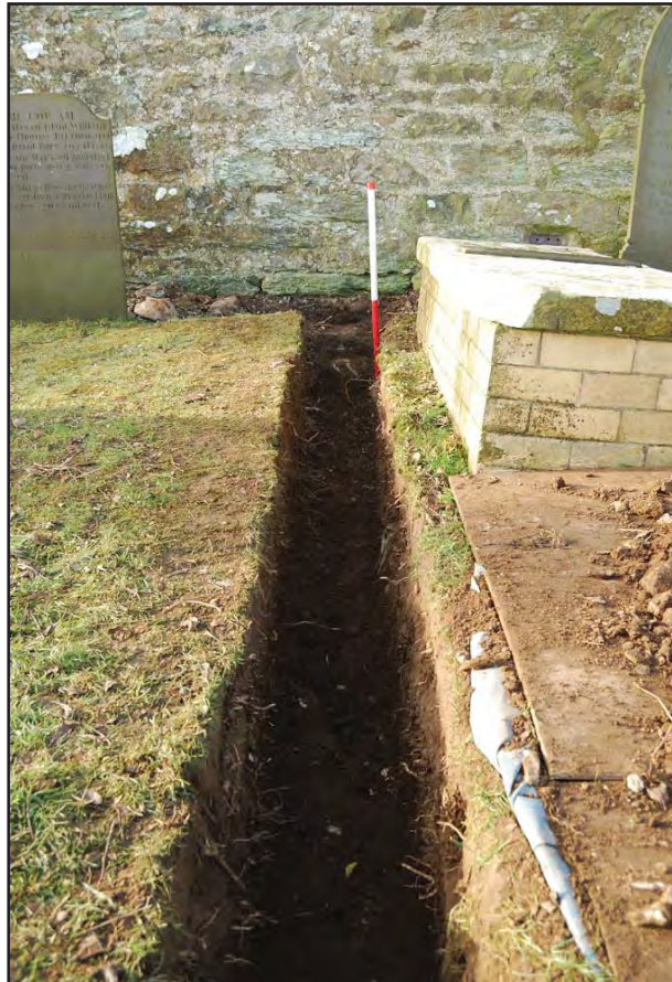
Plate 03: The pipe trench excavated through the churchyard. Scale 1m. (photographic archive ref. G2488_013)
