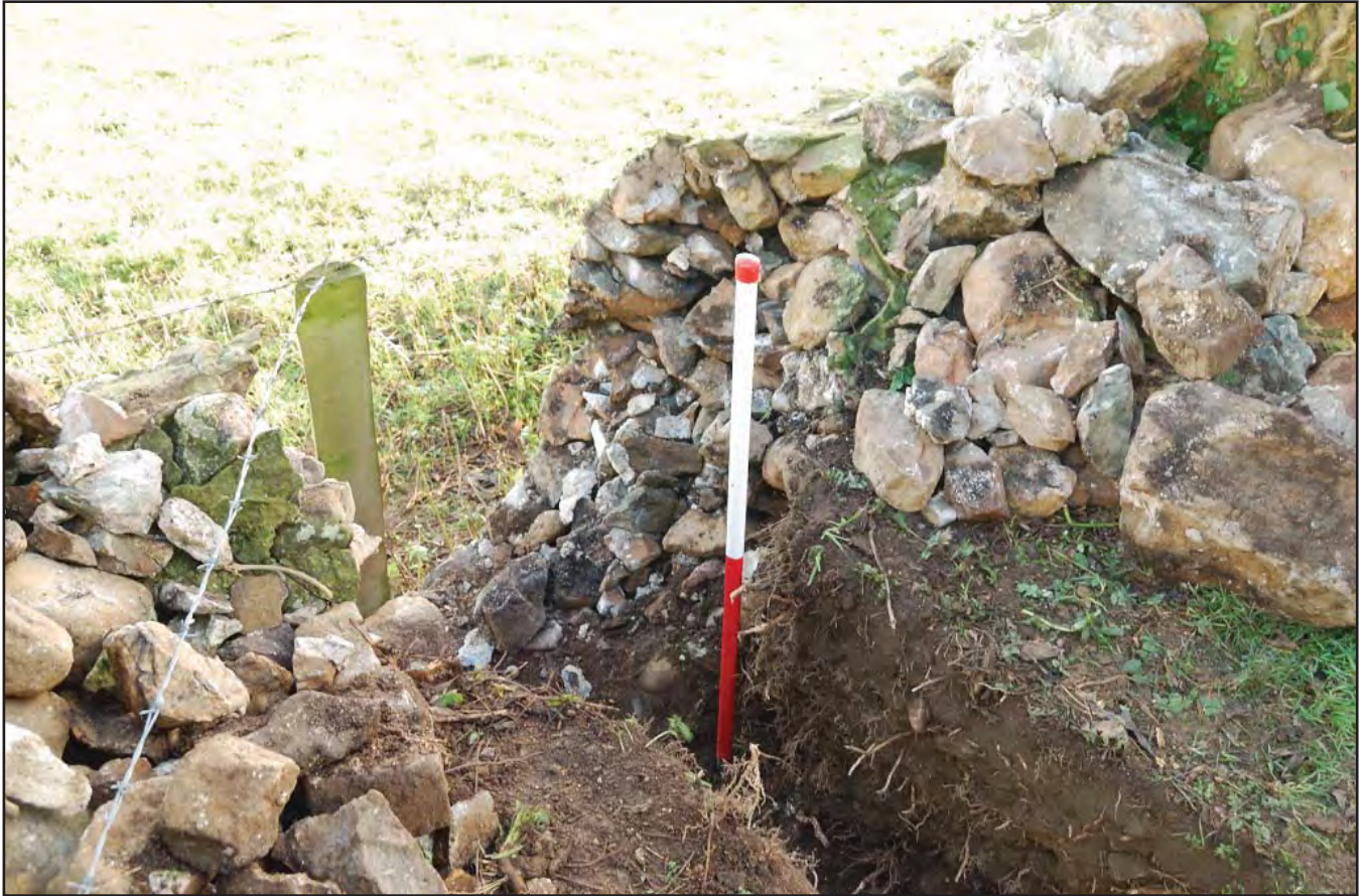
Plate 09: Section through retaining wall. Scale 1m. (photographic archive ref. G2488_014)
