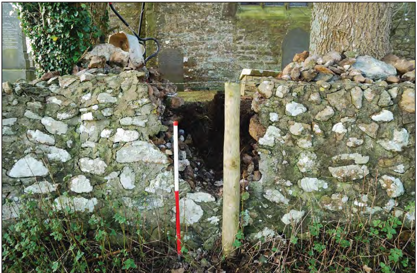
Plate 04: Pipe trench breach through the retaining wall. Scale 1m. (photographic archive ref. G2488_015)
