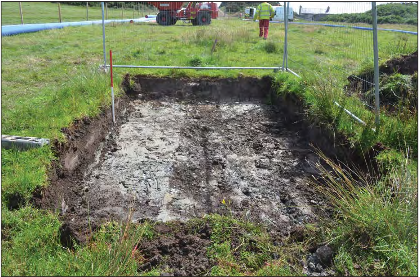
Plate 13: A to B - Field 18, pipe bursting pit showing trench of 12" AC 1966 water main. Scale = 1m.
