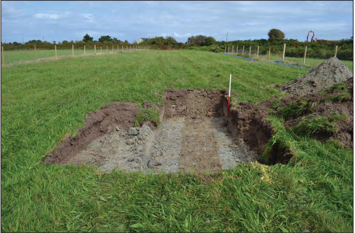
Plate 09: A to B - Field 09 pipe bursting pit showing trench of 12" AC 1966 water main. View from the south west. Scale = 1m.
