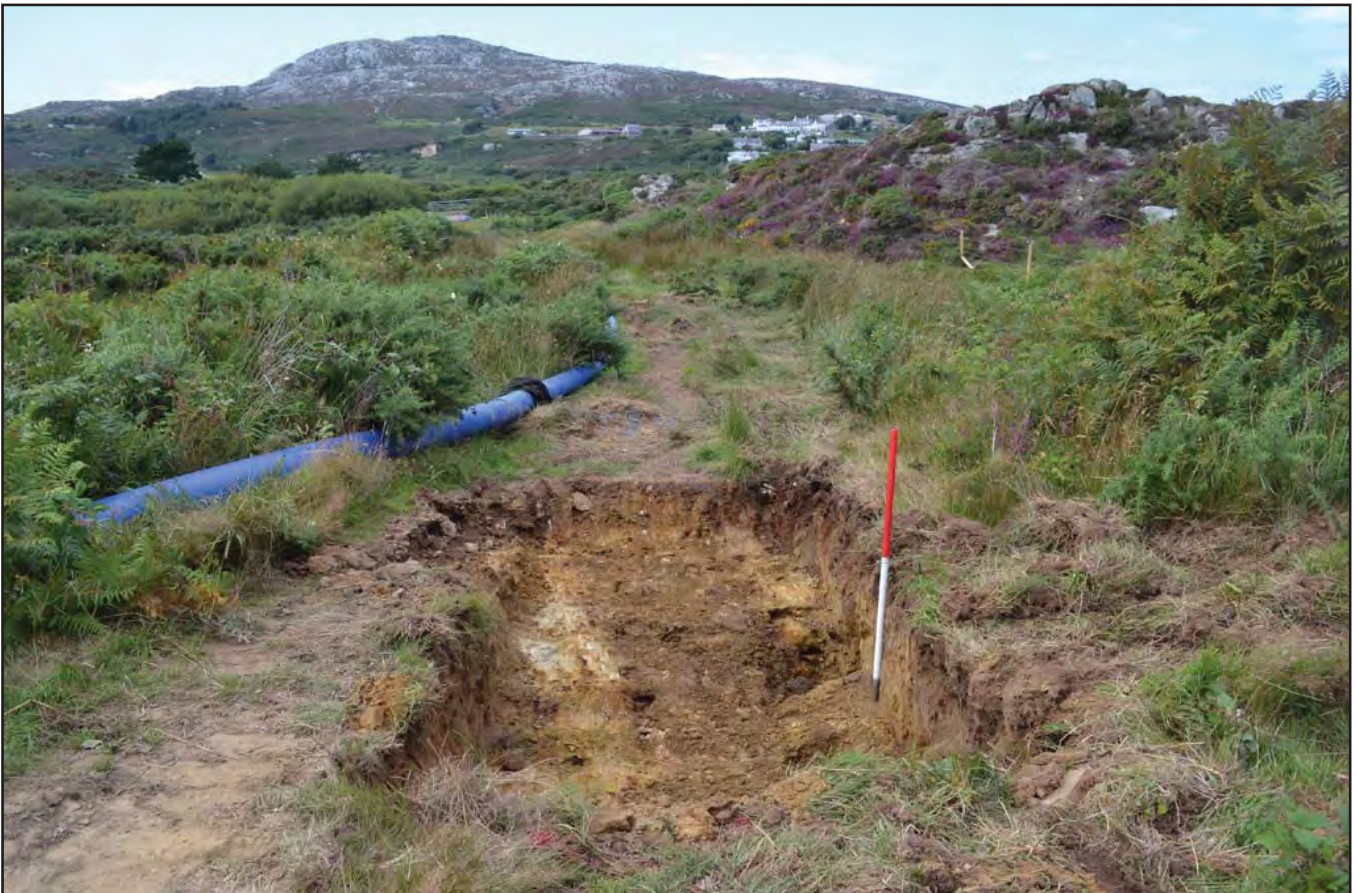
Plate 12: A to B - Field 17, pipe bursting pit showing 12" AC 1966 water main trench in the pit. View from the south east. Scale = 1m.
