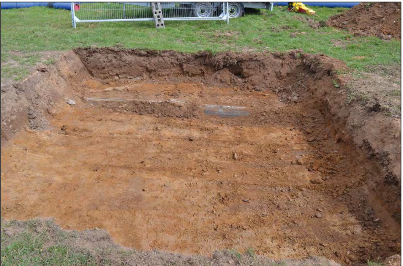
Plate14: A to B - Field 19, pit excavated to locate 12" AC 1966 water main for pipe bursting.
