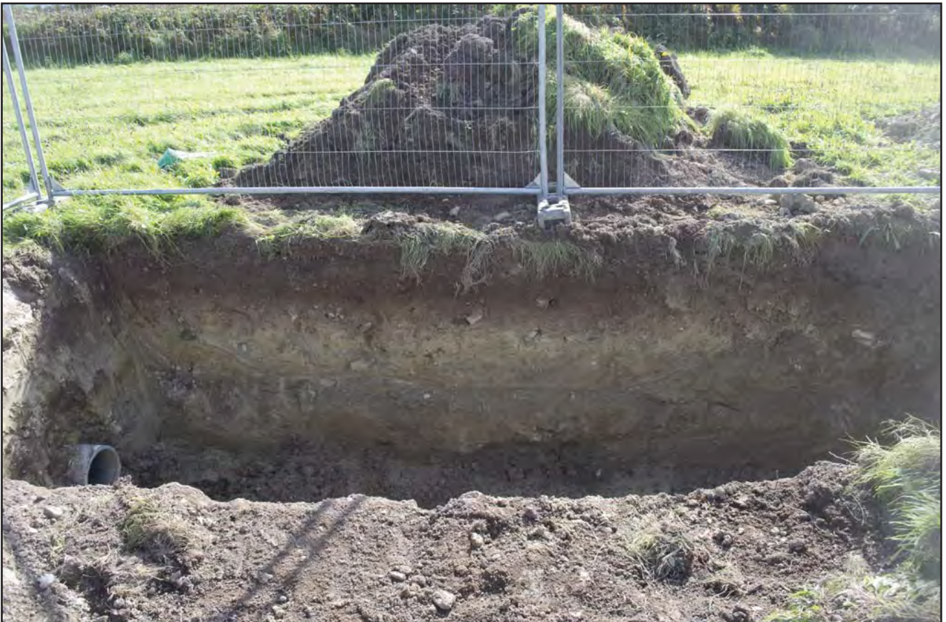
Plate 06: A to B - Field 05, north west facing section of pipe bursting pit. 12" AC 1966 water main visible in pit.
