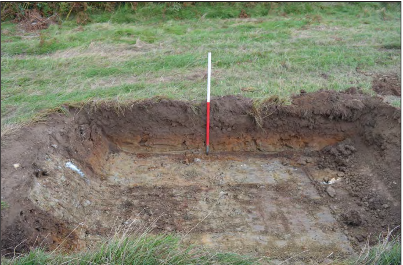
Plate 10: A to B - Field 10, north west facing section of pipe bursting pit excavated over 12" AC 1966 water main. Scale = 1m.
