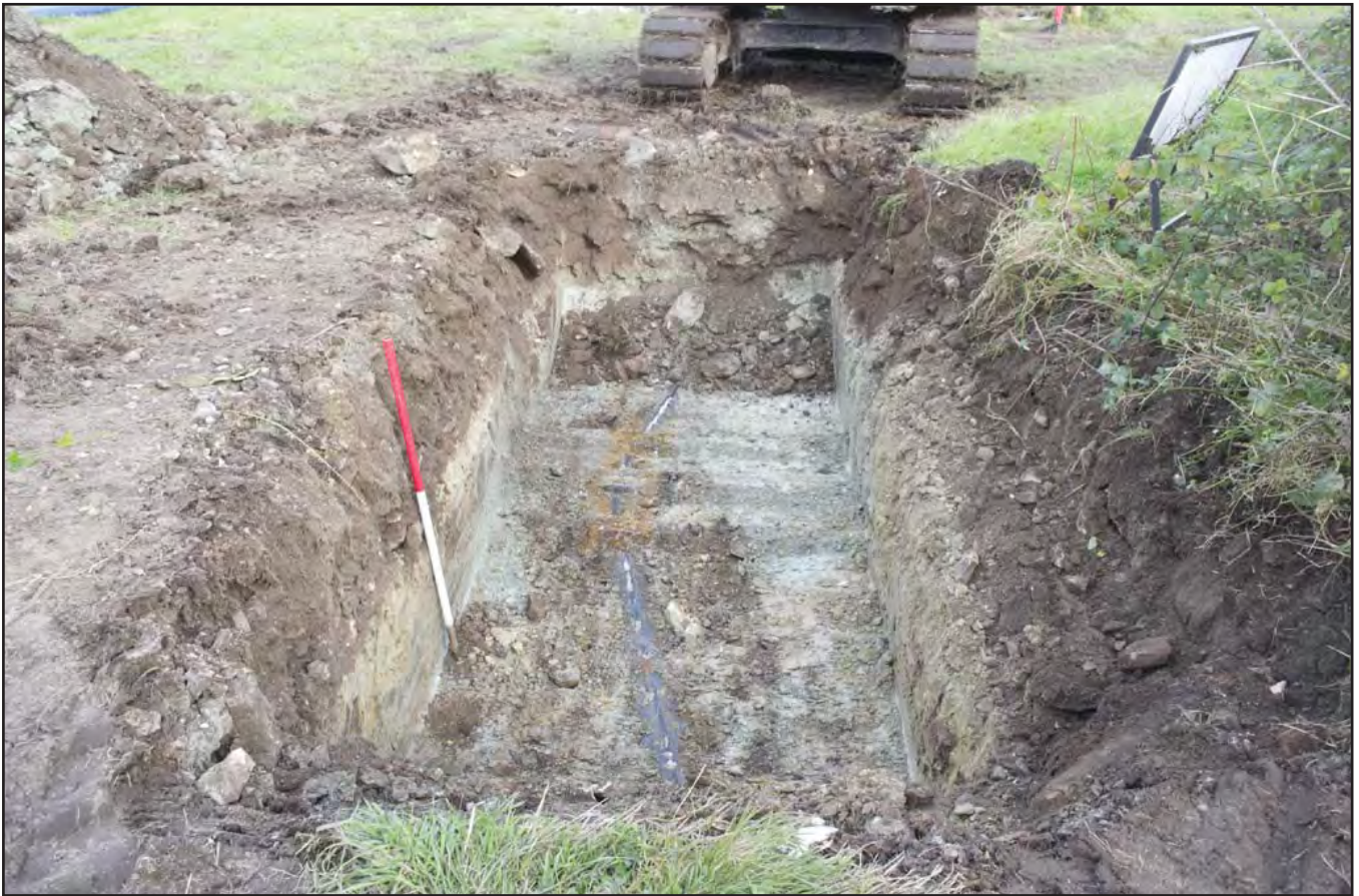
Plate 07 : A to B - Field 06, pit excavated over bend in 12" AC 1966 main . Scale = 1m.
