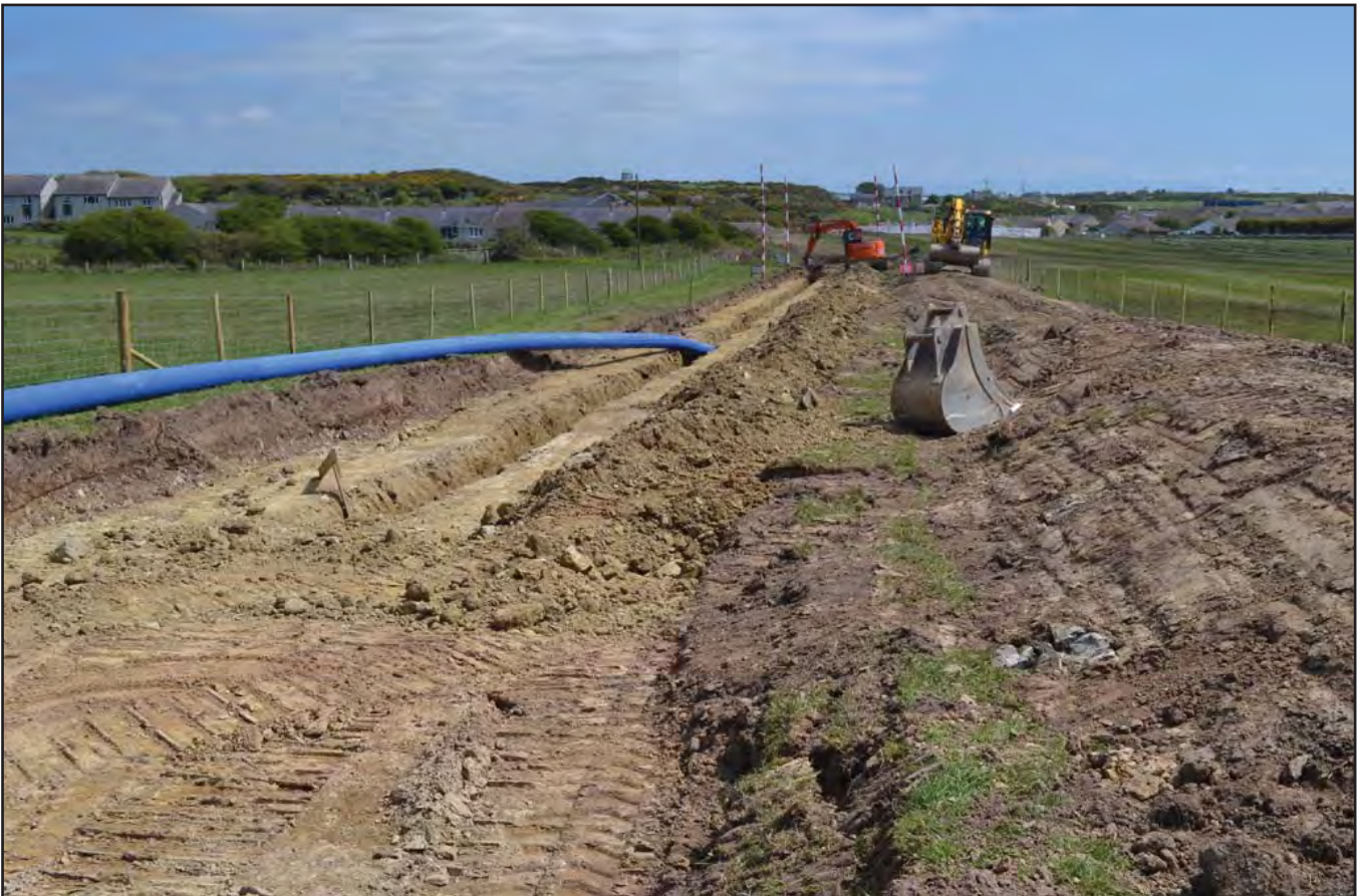
Plate 28: B to E - Field 4, working shot showing pipe trench in open cut area.
