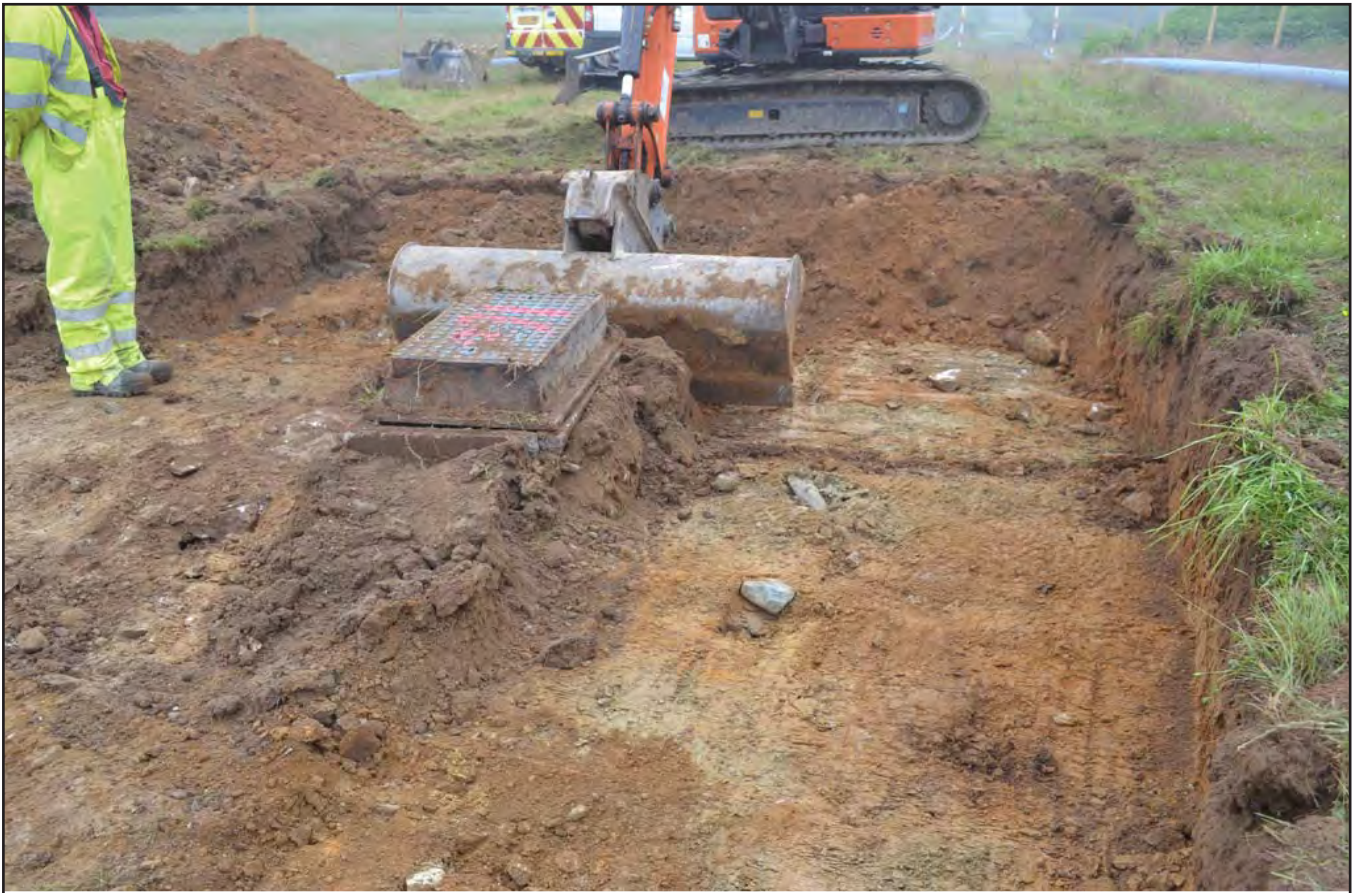
Plate 17: A to B - Field 21, working shot of controlled strip around the air valve at the start of the open cut through Fields 21 and 20.
