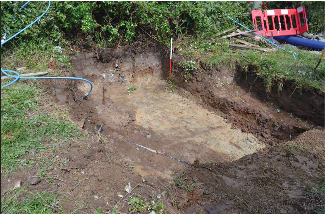
Plate 22: B-E Field 1, pit excavated at field boundary with Plas Road showing 12" AC water main trench. Scale =1m.
