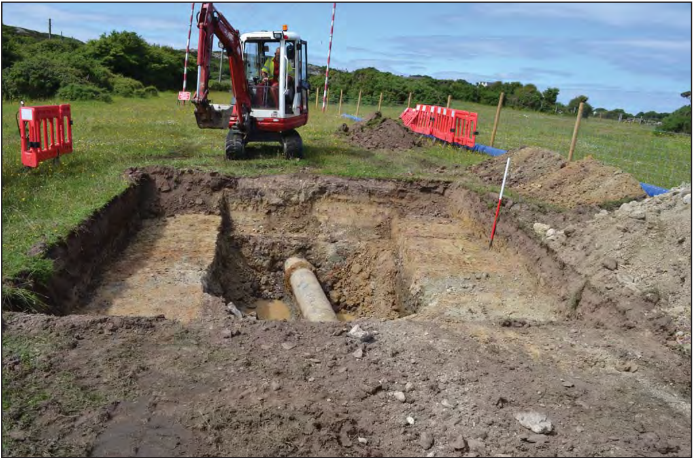
Plate 19: A to B - Field 22, pit excavated over 12" AC 1966 water main. View from the south east. Scale = 1m.
