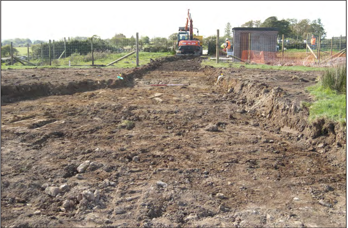
Plate 07: Topsoil strip for access road and sub-station area. Scale = 1m.
