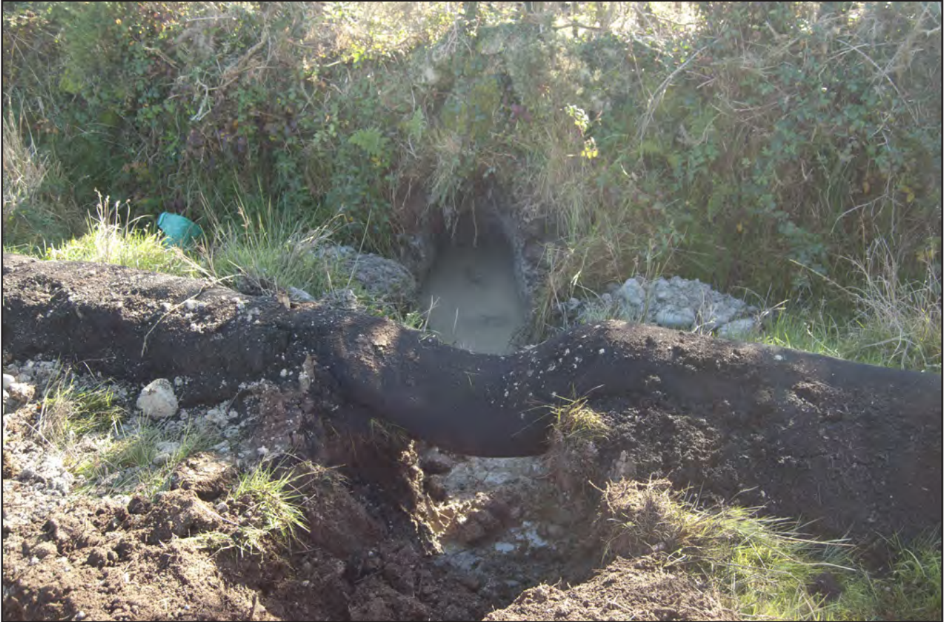
Plate 03: Cable trench excavated under boundary wall between fields A and B.
