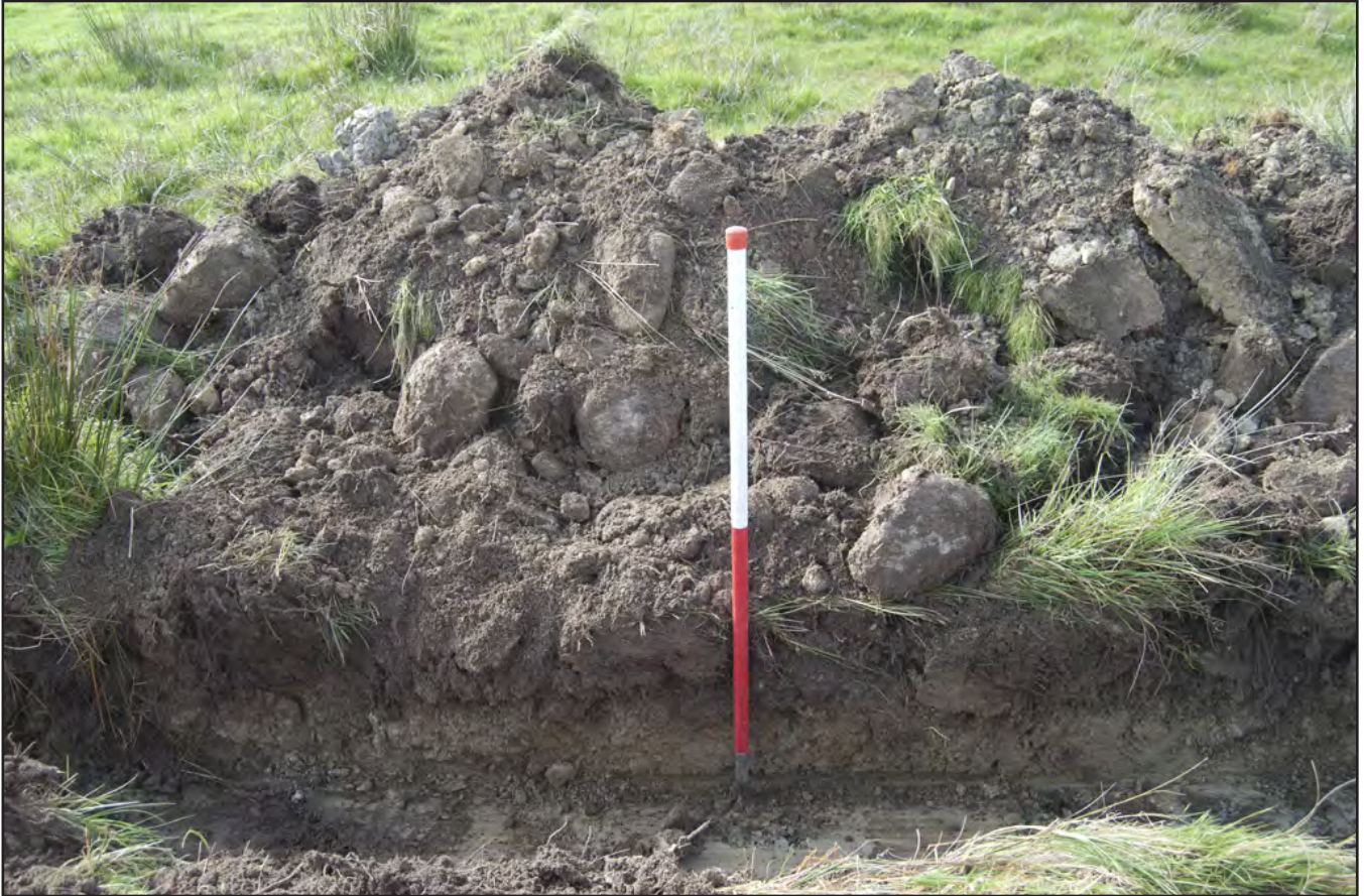
Plate 05: North east facing section of the cable trench in Field B. Scale = 1m.
