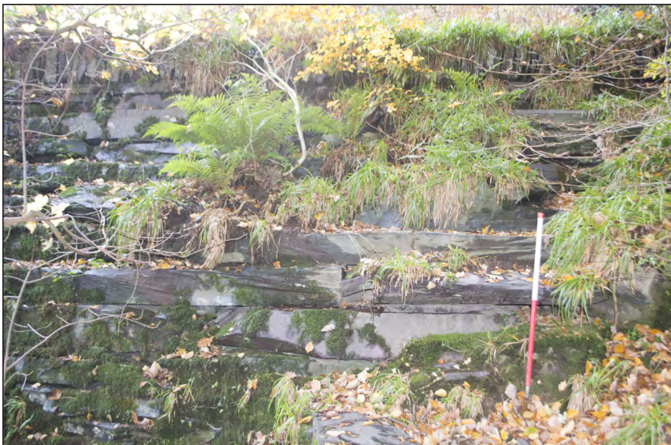
Plate 14: Feature 10 (PRN 56243) view from south of large slate slabs used for dam's construction. Scale 1m. (photographic archive ref. G2487_029)
