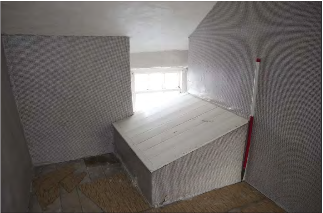
Plate 71: Attic 2: Room C - interior view detailing wooden construction likely used as draft excluder. Scale: 1.0m (archive image: G2483_145).
