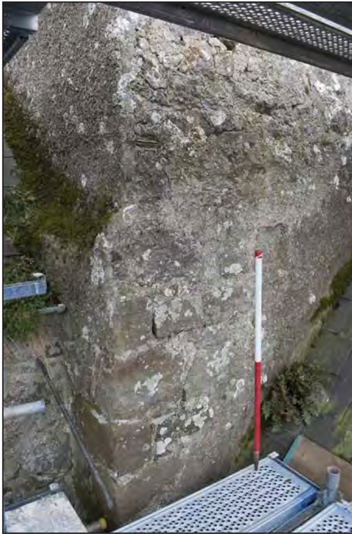
Plate 79: Detail of medieval quoins in northeast corner of former chapel at first floor level; scale: 1.0m (archive image: G2483_192).
