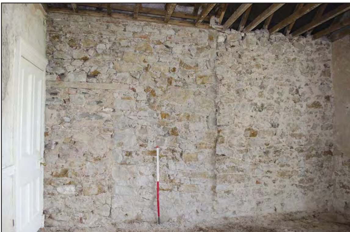
Plate 26: Dining Room - interior view of west wall with detail of blocked door way and later extension walls. Scale: 1.0m (archive image: G2483_181).
