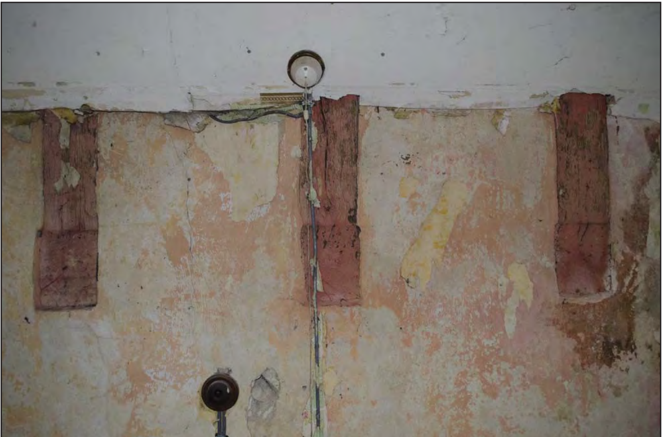
Plate 64: Disused Chapel - interior view detailing truncated beams. Scale: 1.0m (archive image: G2483_157).
