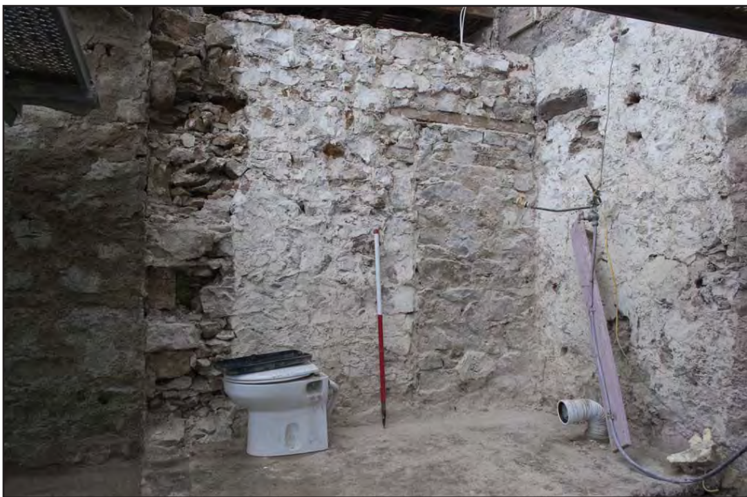
Plate 80: Blocked doorway in northwest rear gable wall; scale: 1.0m (archive image: G2483_195).
