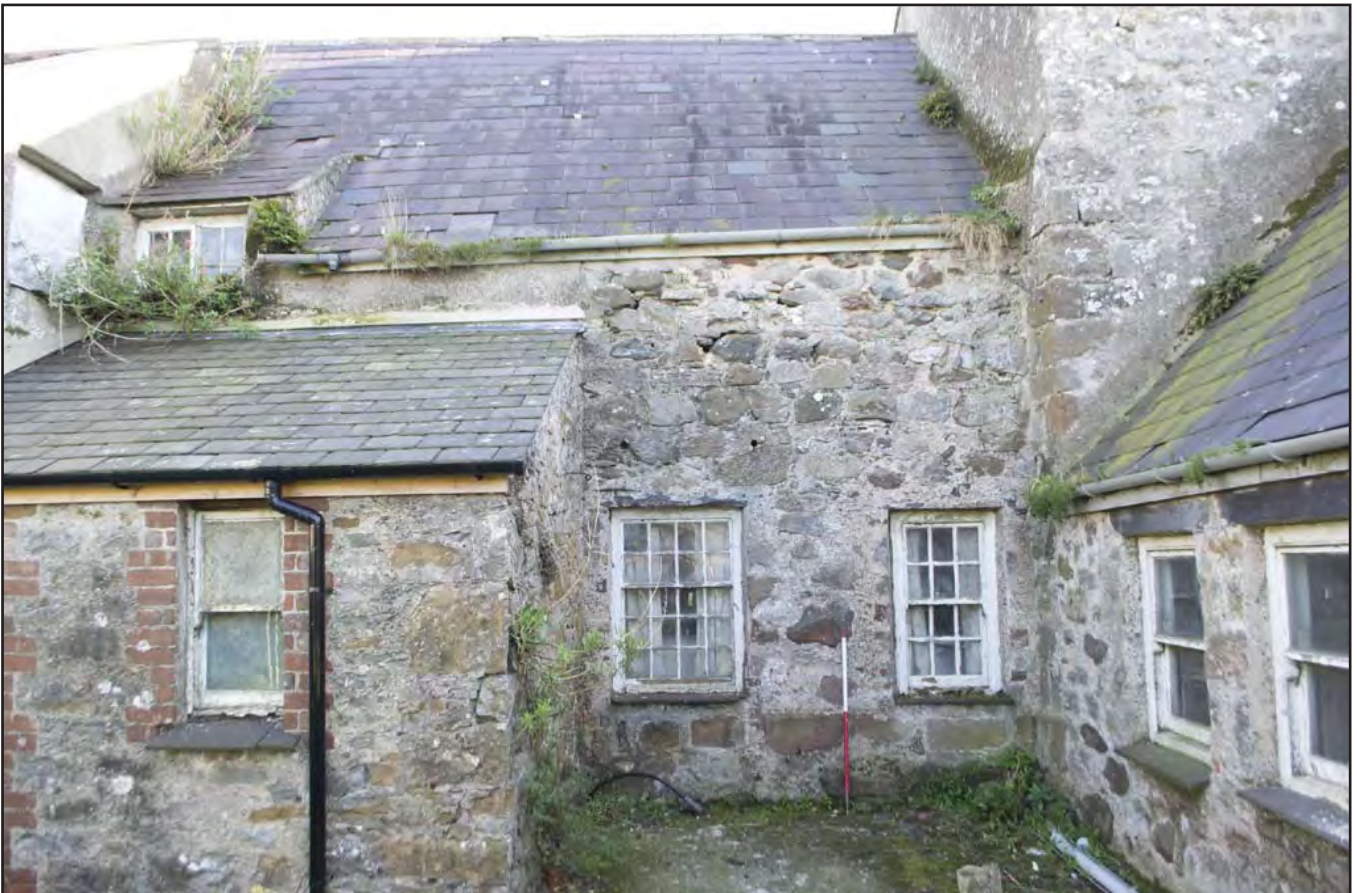
Plate 08: Rear Elevation - view from the northeast detailing disused chapel wall and junction with the nave showing quoins. Scale: 1.0m (archive image: G2483_188).
