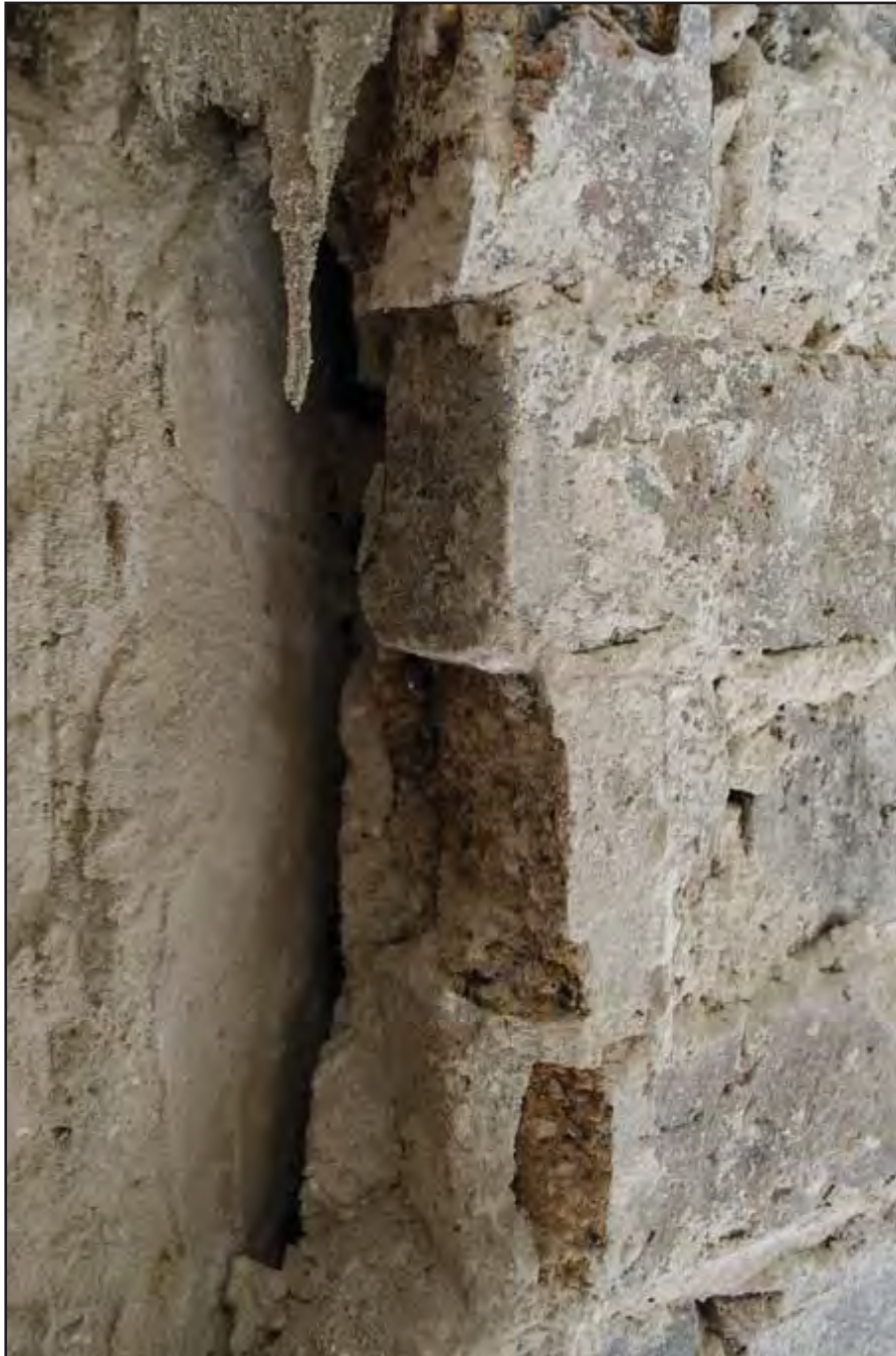
Plate 39: Living Room 1 - interior view with detail of structural phasing associated with bay window W11 (archive image: G2483_061).
