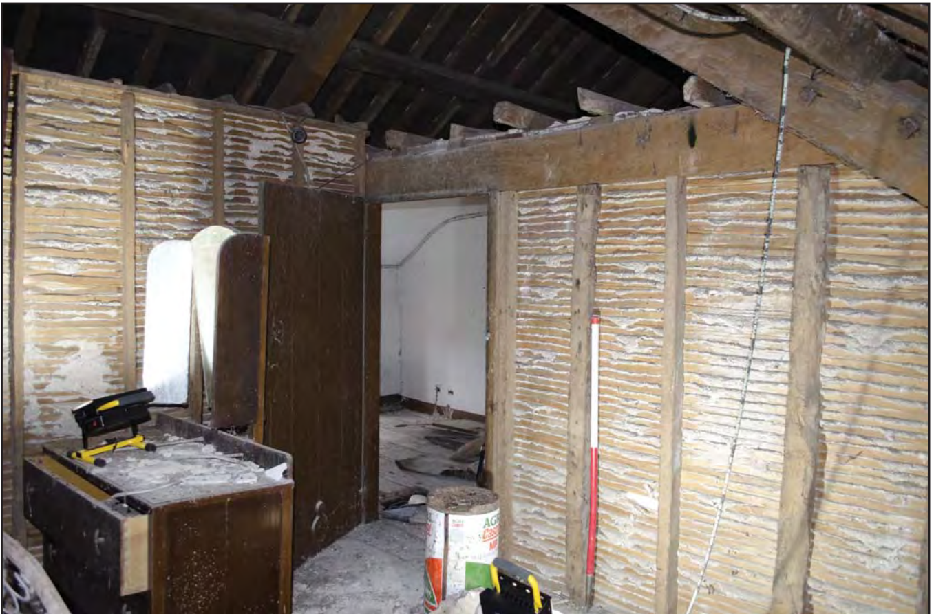
Plate 68: Attic 1: Room A - interior view detailing plaster laths, roof space storage and door D28. Scale: 1.0m (archive image: G2483_136).
