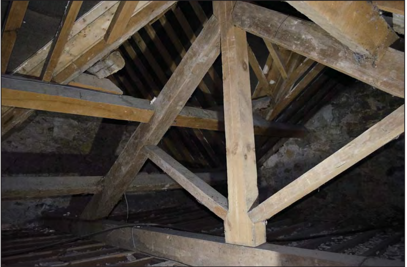
Plate 73: Attic 3 - interior view detailing roof space area with modern beams (archive image: G2483_153).
