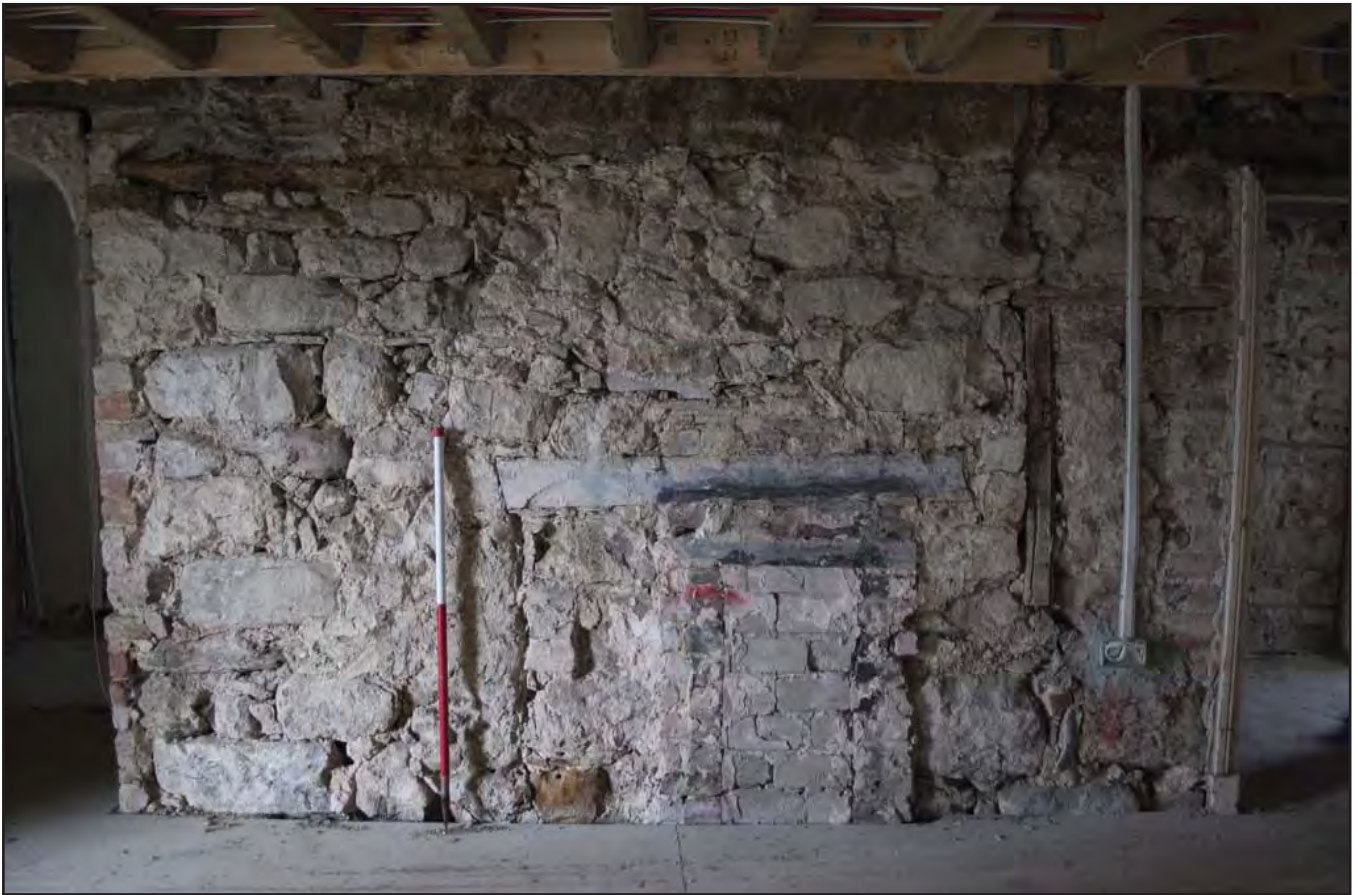
Plate 87: Internal view of east-facing elevation in Hall 1, showing two blocked former fireplaces; scale: 1.0m (archive image: G2483_214).
