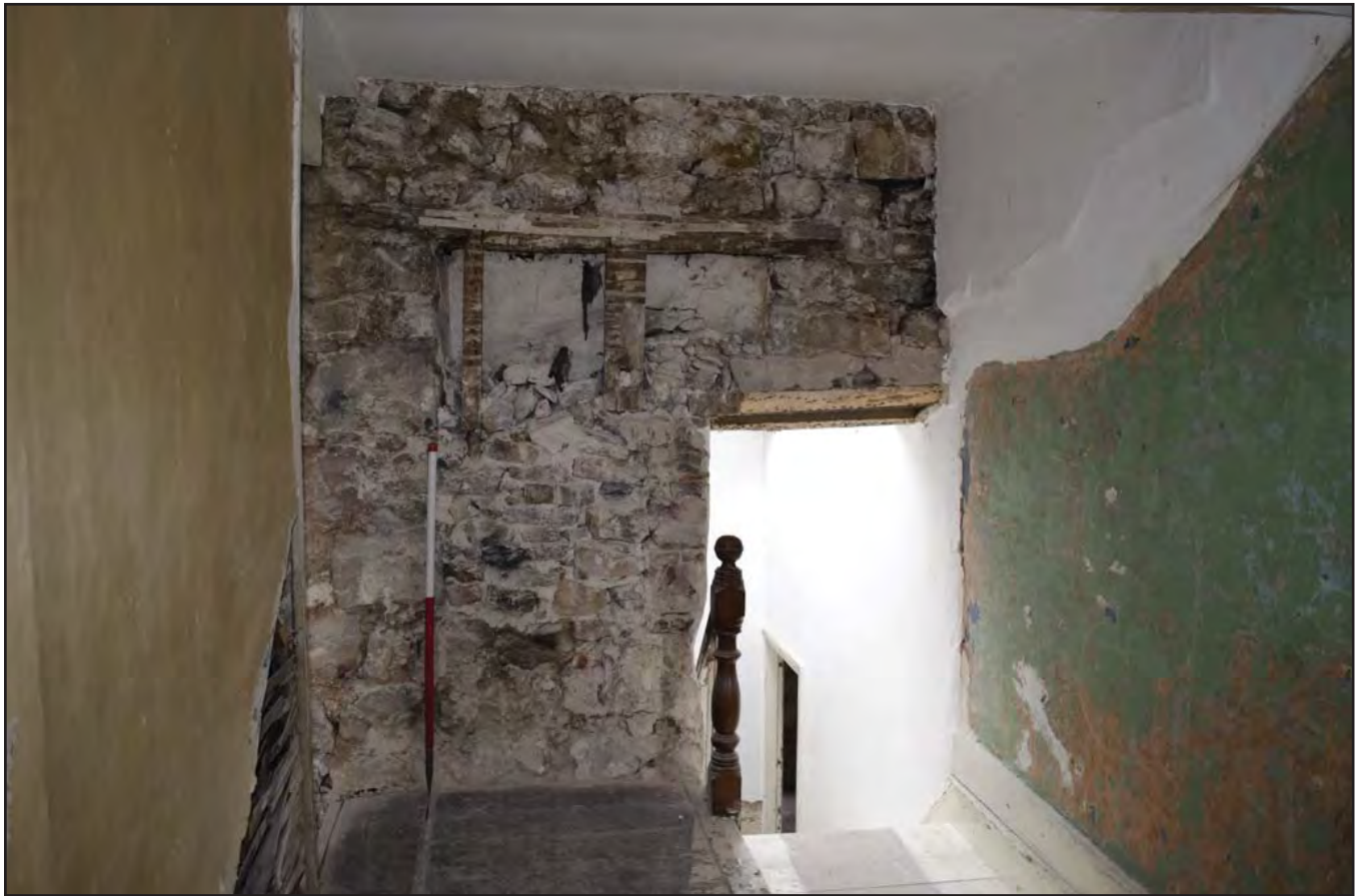
Plate 55: Corridor - interior view detailing stone wall and what appears to have once been a window. Scale: 1.0m (archive image: G2483_108).
