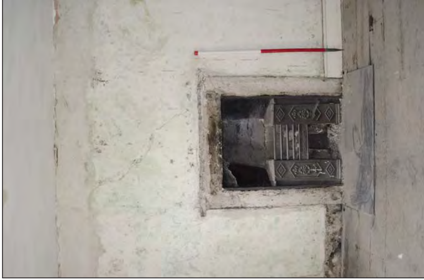
Plate 57: Bedroom 2 - interior view detailing Victorian fireplace F07, surrounded by 18th century plaster. Scale: 1.0m (archive image: G2483_114).
