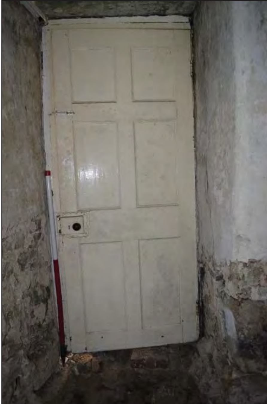
Plate 19: Store - interior view detailing door D06 and showing late Victorian/Edwardian door knob. Scale: 1.0m (archive image: G2483_036).
