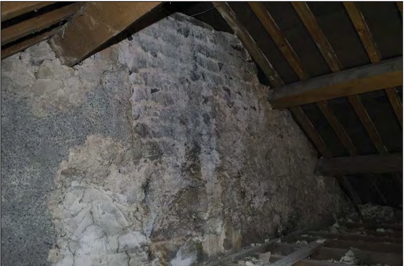
Plate 74: Attic 3 - interior view detailing terminus wall at E-end with 18th century plaster (archive image: G2483_155).
