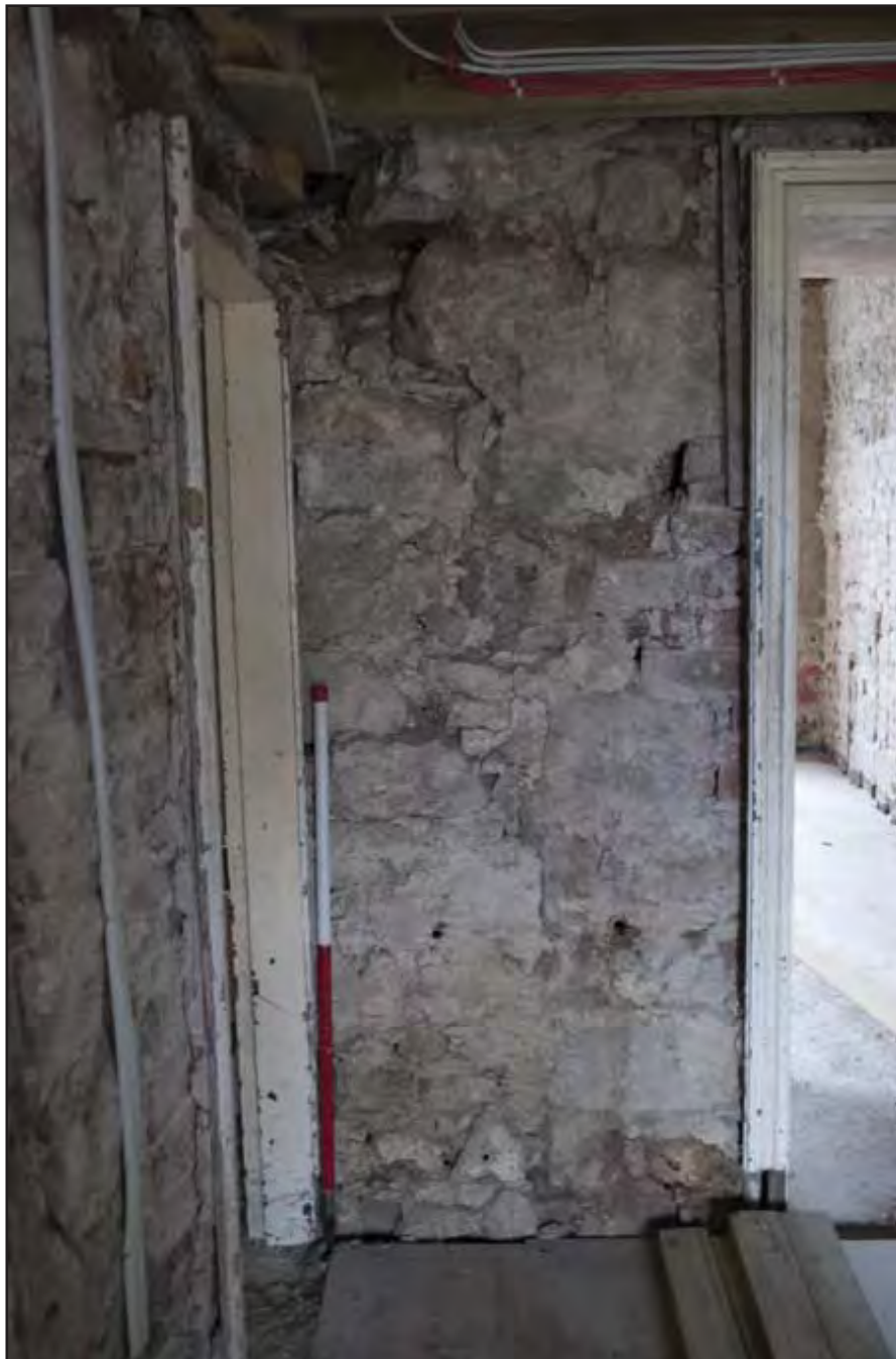
Plate 89: Detail of chamfered stone edge in south-facing internal elevation in Hall 1; scale: 1.0m (archive image: G2483_217).
