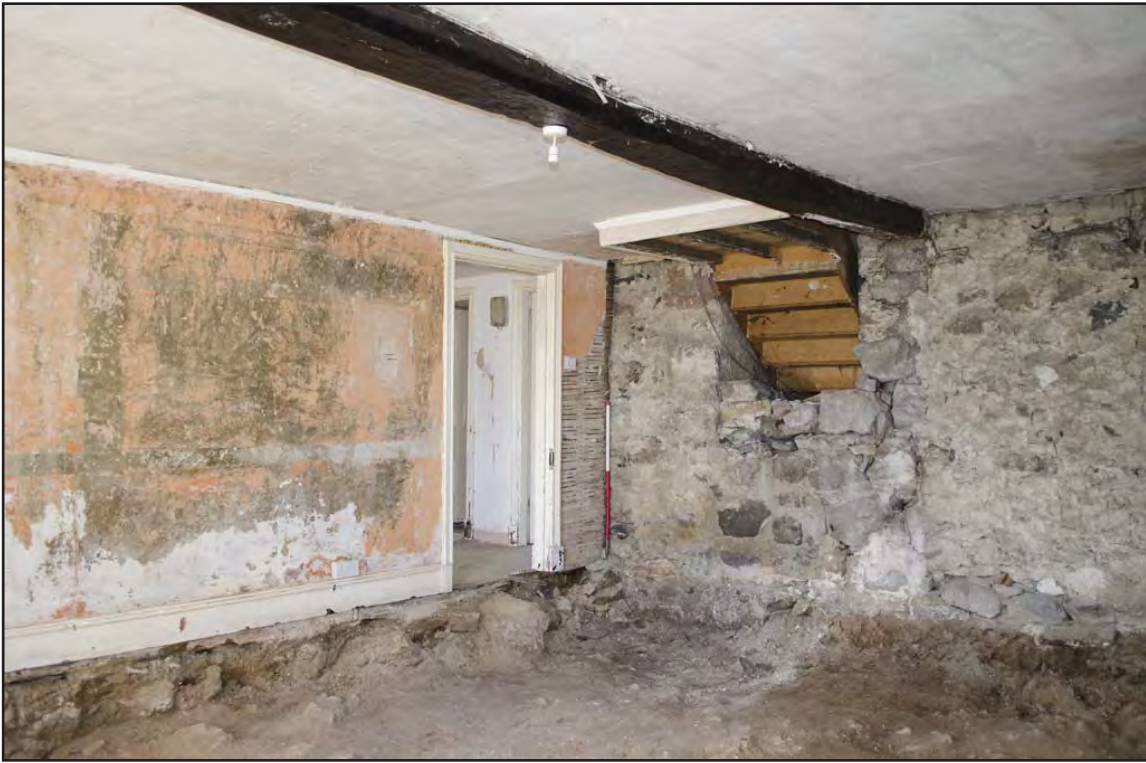
Plate 43: Living Room 2 - interior view showing rear of back stair case, earlier foundations and door D16. Scale: 1.0m (archive image: G2483_066).
