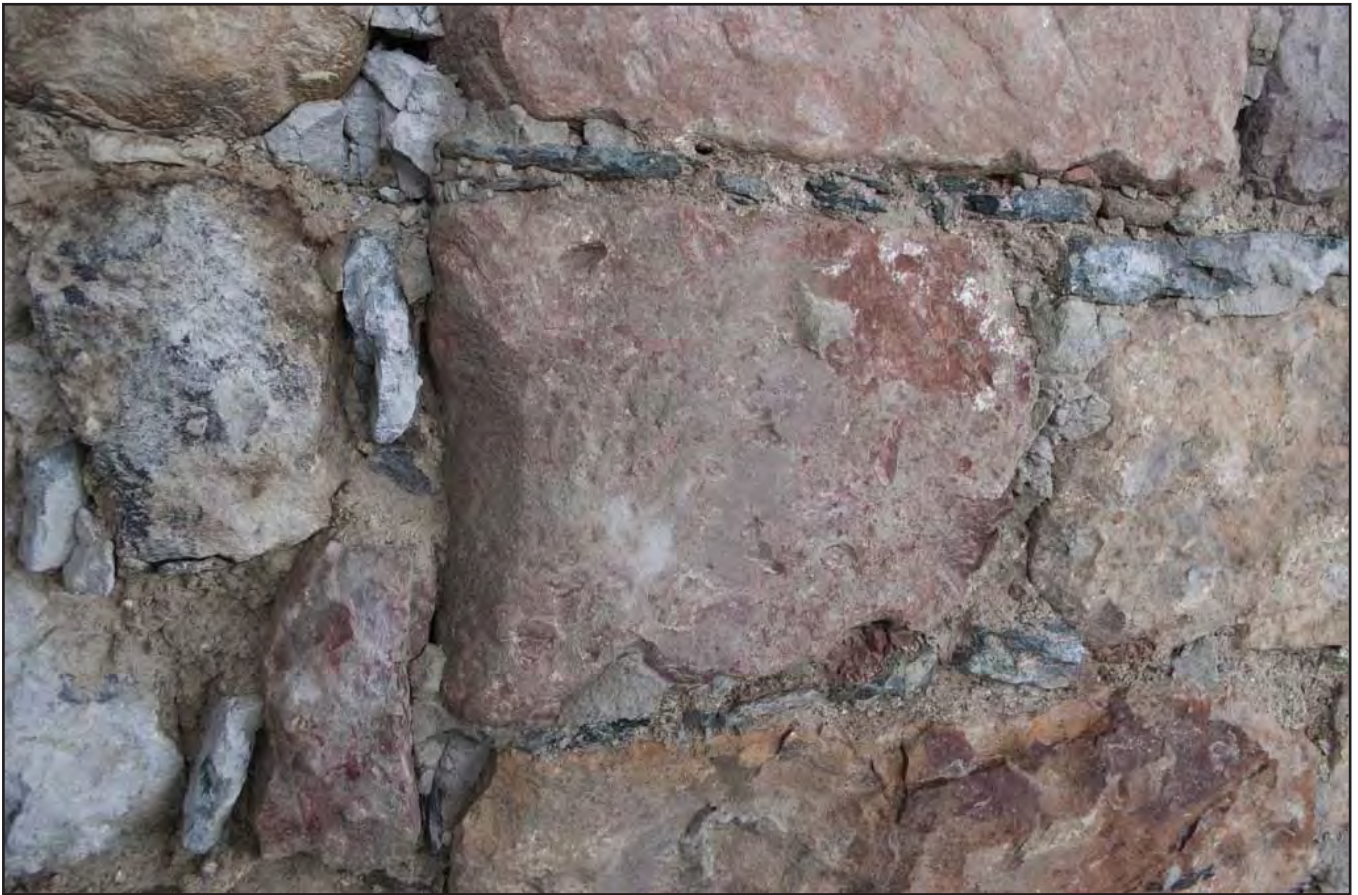
Plate 83: Detail of medieval quoin showing wear created by probable tool sharpening (archive image: G2483_204).
