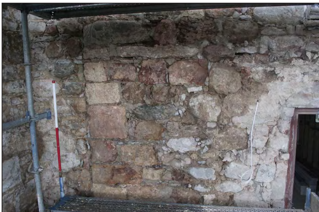
Plate 82: Large quoins and butt joint at the former west end of the grange chapel, with medieval masonry; scale: 1.0m (archive image: G2483_203).
