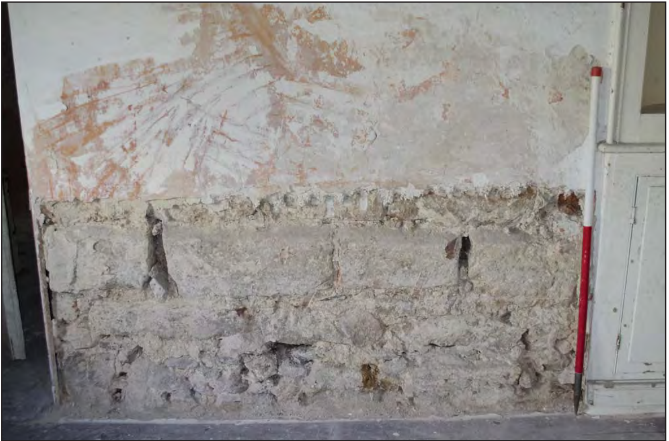
Plate 47: Office - interior view detailing chamfer masonry course, belonging to medieval grange. Scale: 1.0m (archive image: G2483_080).
