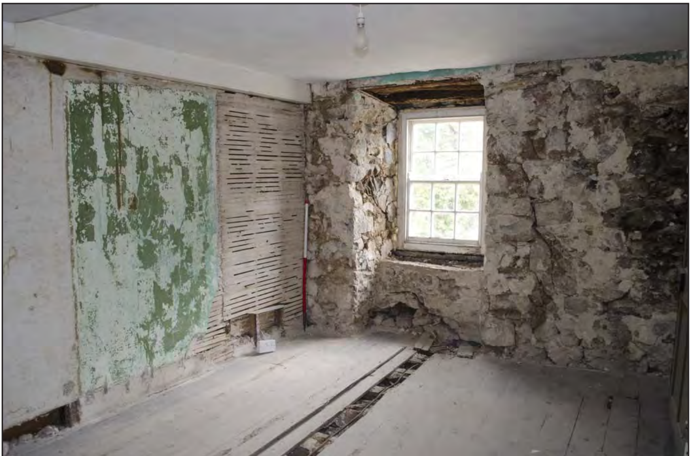
Plate 56: Bedroom 2 - interior view detailing 18th century plaster and original stone wall. Scale: 1.0m (archive image: G2483_111).
