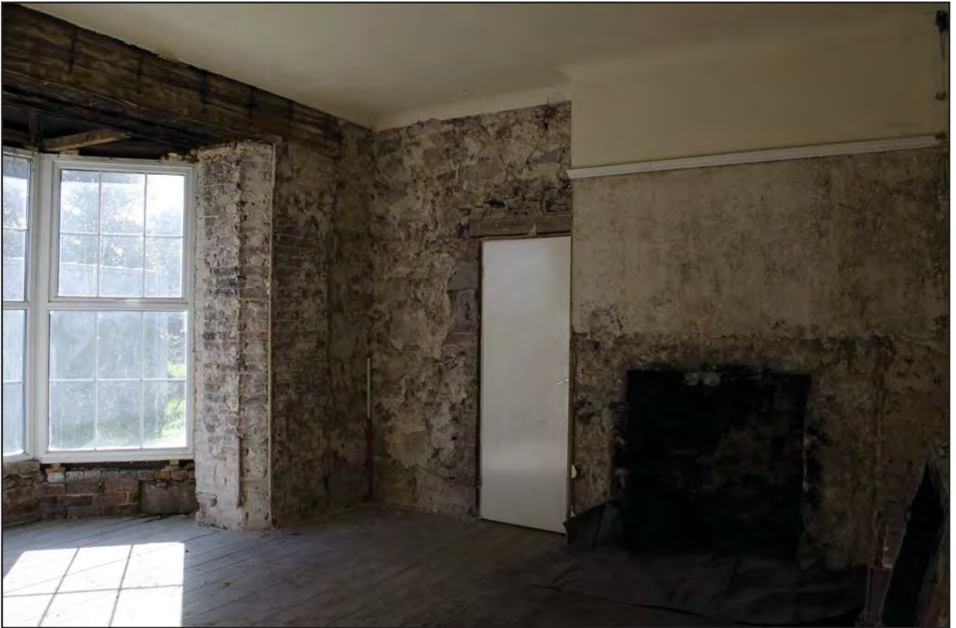
Plate 37: Living Room 1 - interior view with detail of structural phasing including 17th century wall and bay window and door D19 inserted at a later date. Scale: 1.0m (archive image: G2483_055).
