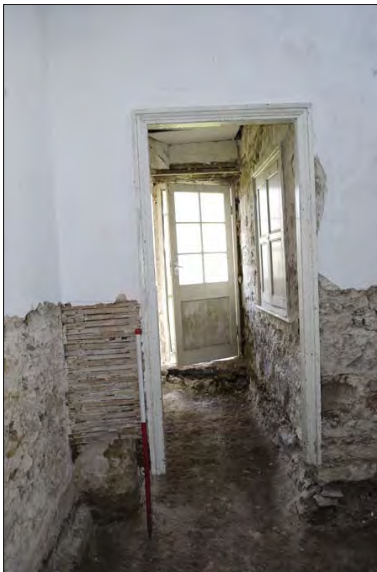
Plate 44: Lobby/Hall - interior view with detail of door D10 and plaster laths . Scale: 1.0m (archive image: G2483_071).
