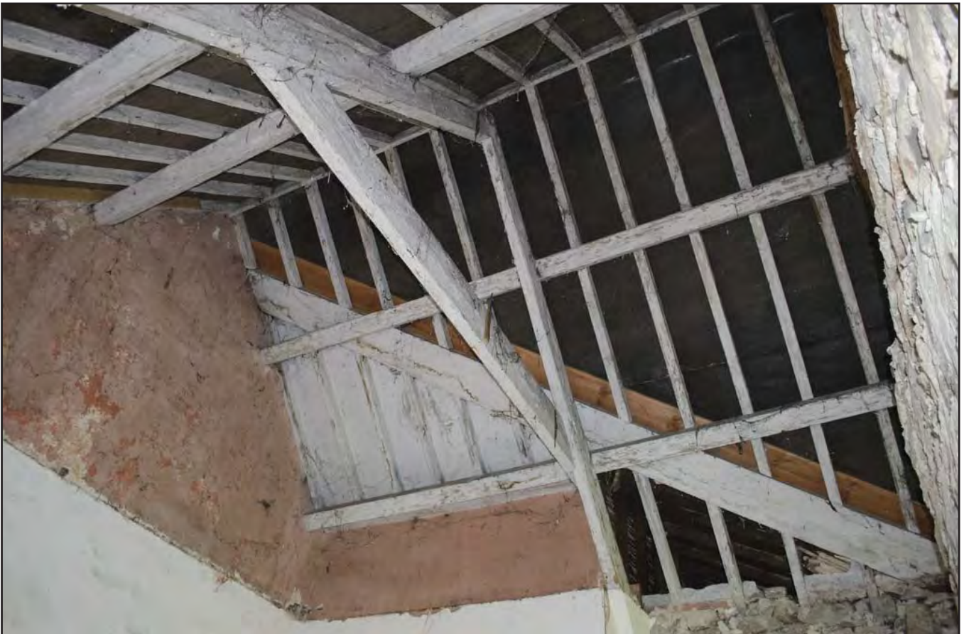
Plate 48: Office - interior view detailing roof beams and A-shaped truss (archive image: G2483_082).
