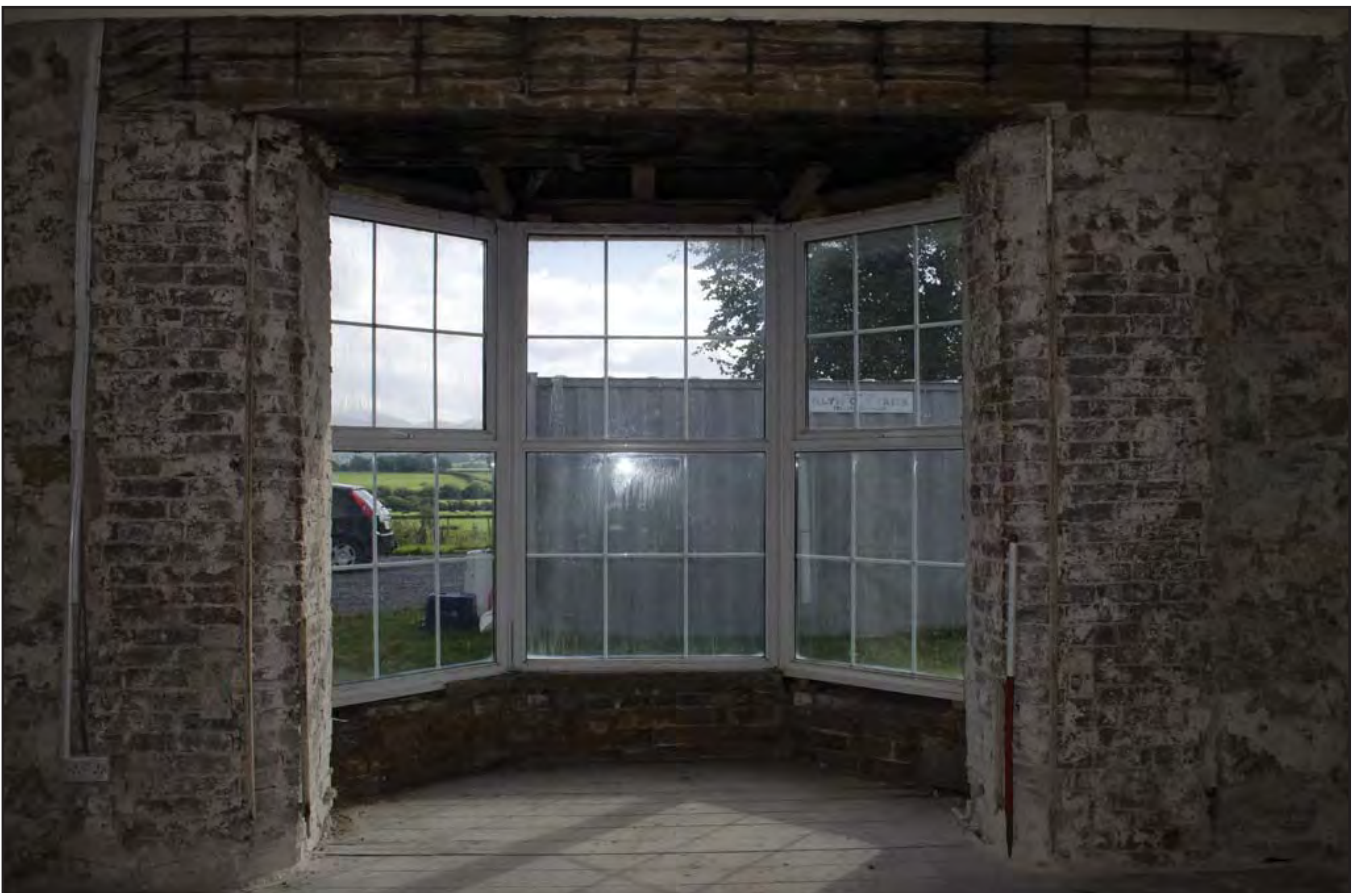
Plate 38: Living Room 1 - interior view with detail of bay window W11 with Victorian brickwork and truss supporting walls above. Scale: 1.0m (archive image: G2483_055).
