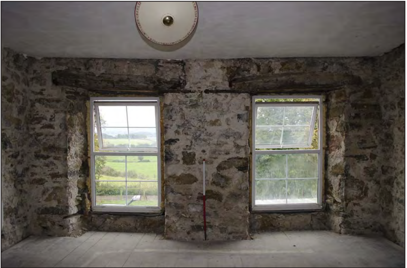
Plate 51: Bedroom 1 - interior view detailing windows W12 and W13, original timber frame above both windows and central iron supports. Scale: 1.0m (archive image: G2483_091).
