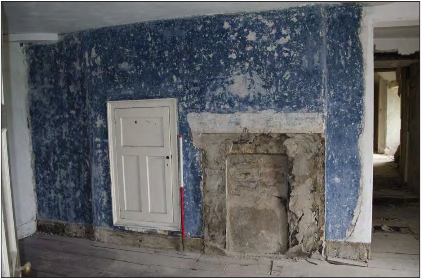
Plate 61: Bedroom 4 - interior view of blocked-up fireplace F09, built in cupboards C03 and chimney breast. Scale: 1.0m (archive image: G2483_124).
