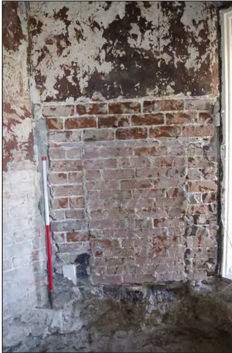
Plate 17: Utility - interior view detailing blocked-up fireplace F02. Scale: 1.0m (archive image: G2483_034).
