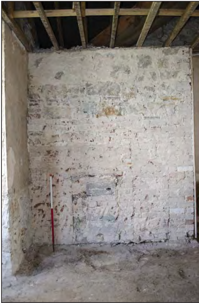
Plate 25: Dining Room - interior view with detail of of blocked-up fireplace F03. Scale: 1.0m (archive image: G2483_046).
