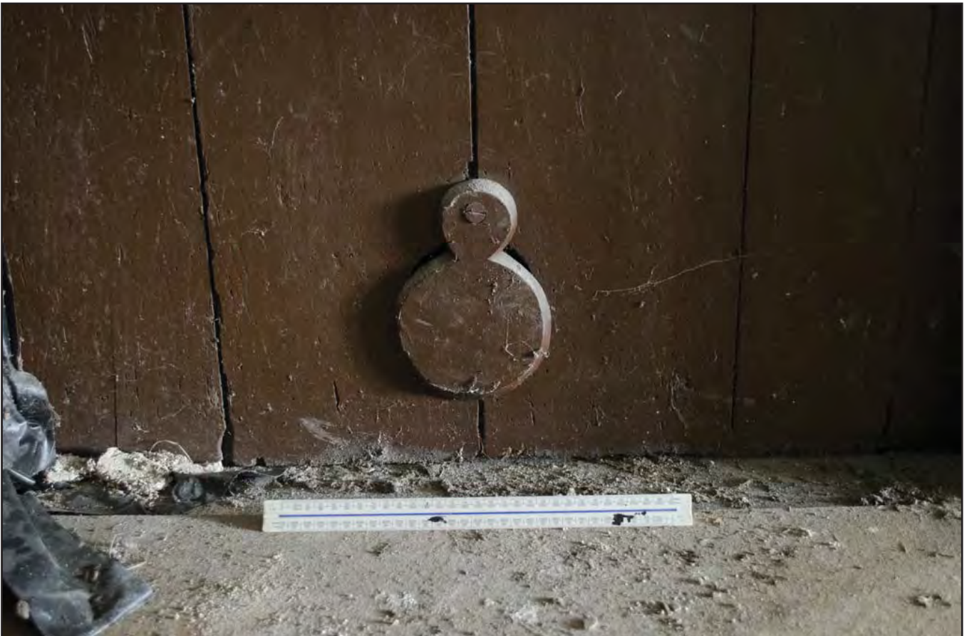
Plate 72: Attic 1: Lobby - interior view detailing circular flap (c.0.24m) at the base of door D28 - closed. Scale: 0.30m (archive image: G2483_151).
