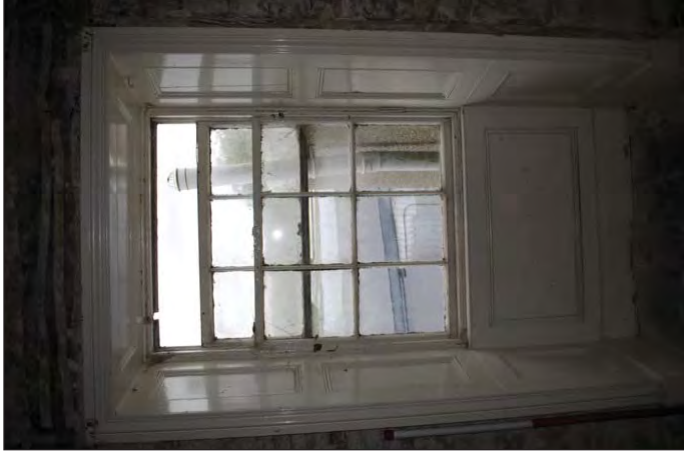
Plate 53: Bedroom 1 - interior view detailing window W20 with Georgian wood panelling. Scale: 1.0m (archive image: G2483_097).
