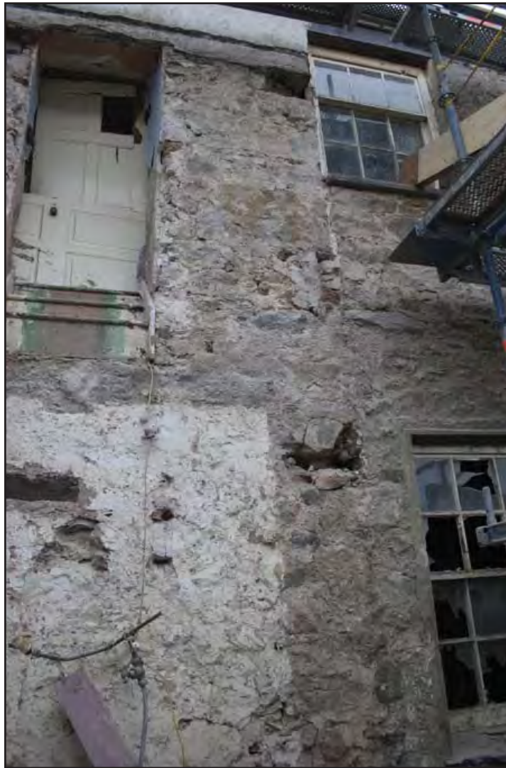
Plate 81: Rear elevation - general view after removal of bathroom extension detailing modifications to the building (archive image: G2483_199).
