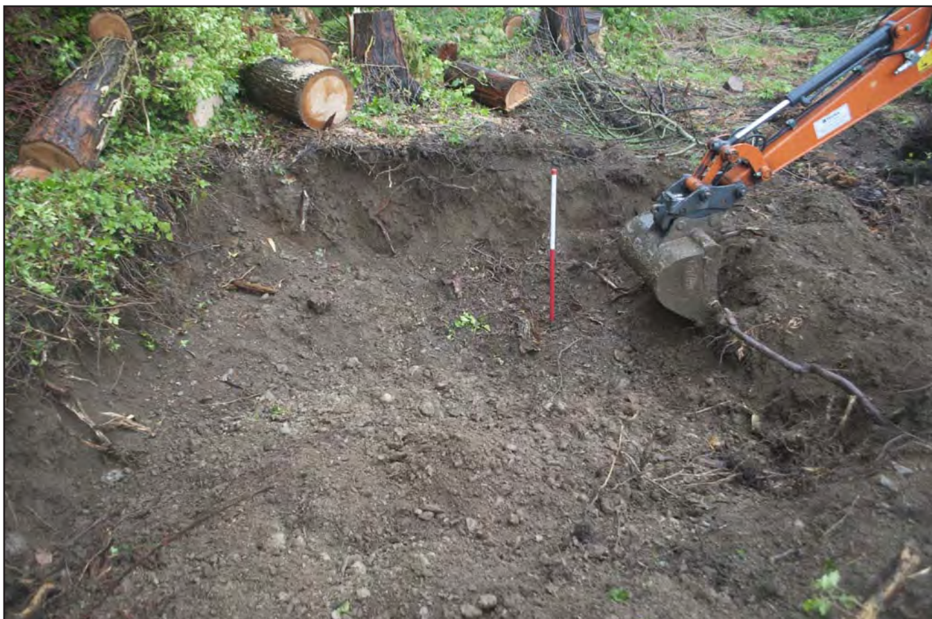
Plate 02: Energy Centre Building: Topsoil stripping at Energy Centre site, viewed from the east; scale 1m (archive image: G2447_066)
