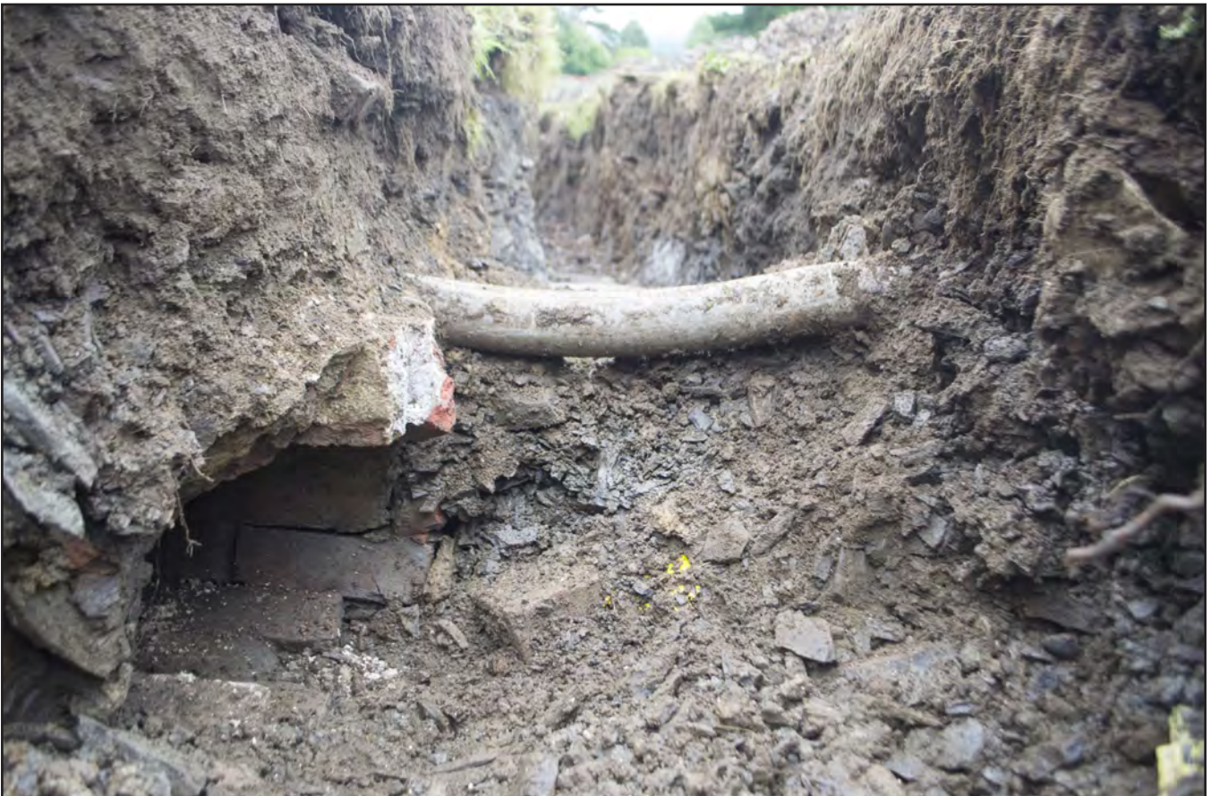
Plate 12: Pipeline 1: Lead pipe and brick tunnel [18^] from within Pipe line 1 as it first appeared at SH 60238 71203 (archive image: G2447_133)
