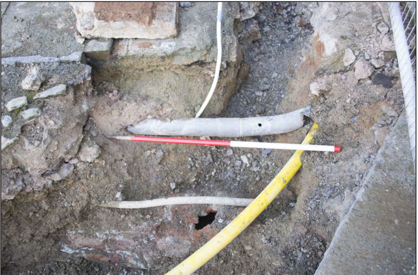
Plate 22: Pipeline 10: Brick service pipe [23^] with lead pipe modern service pipes; 1m scale (archive image: G2447_153)
