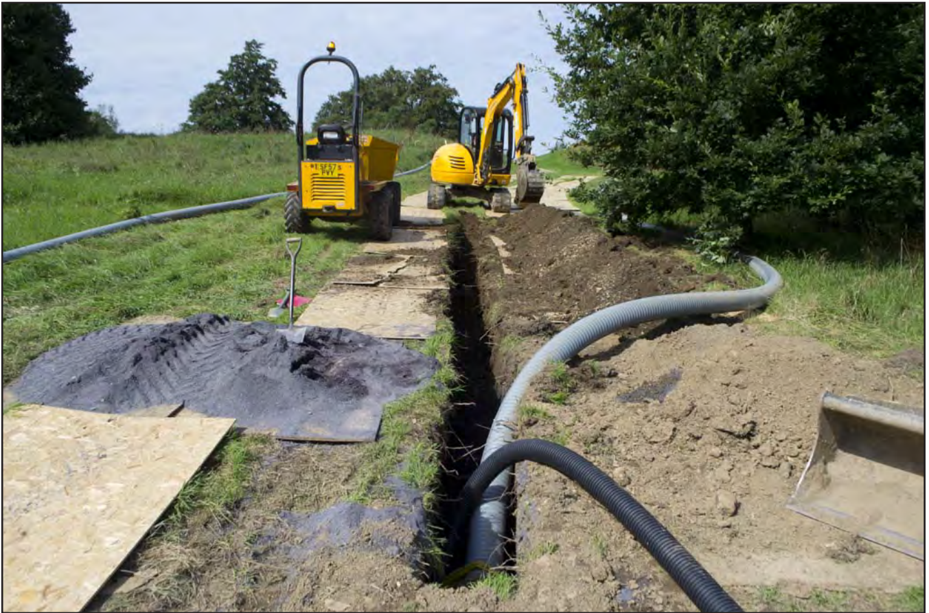
Plate 09: Pipeline 1: Shot along trench during excavation of pipe trench showing previously backfilled area near woodlands (archive image: G2447_123)
