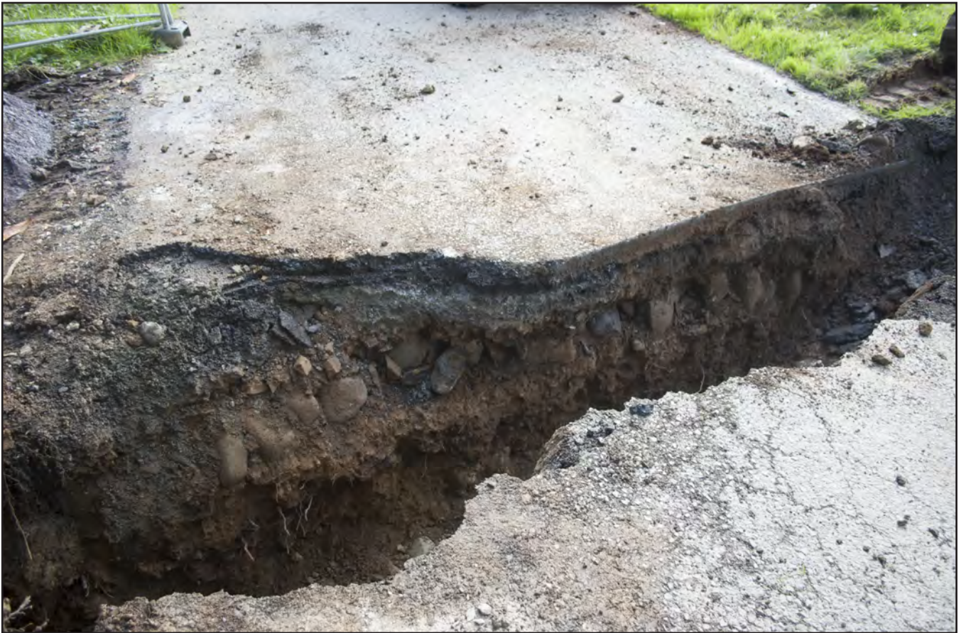
Plate 07: Pipeline 1: Shot of tarmac road showing cobbles in N facing trench section (archive image: G2447_110)
