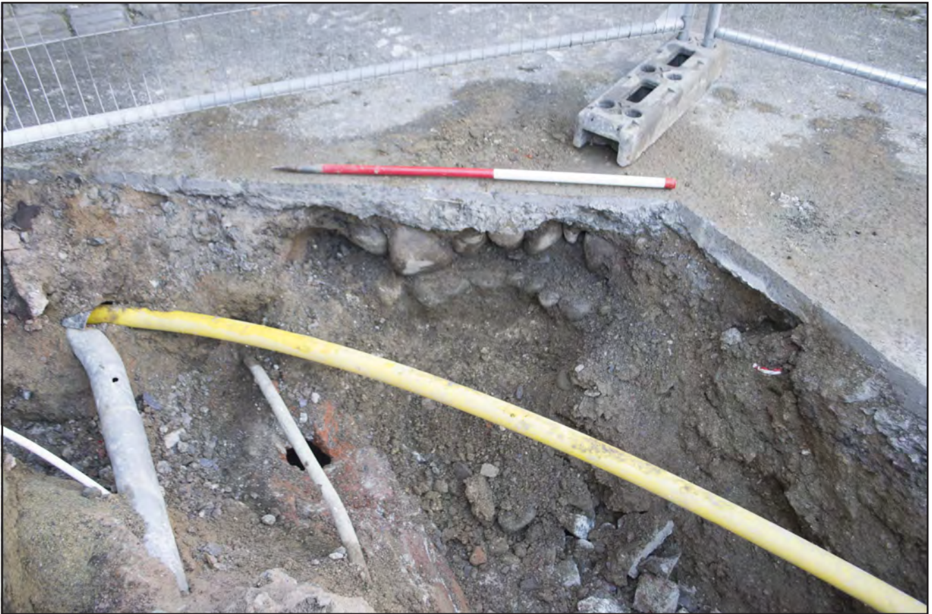
Plate 21: Pipeline 10: Brick service tunnel [23^] with cobbled surface in shot within S end corner of trench; scale 1m (archive image: G2447_155)
