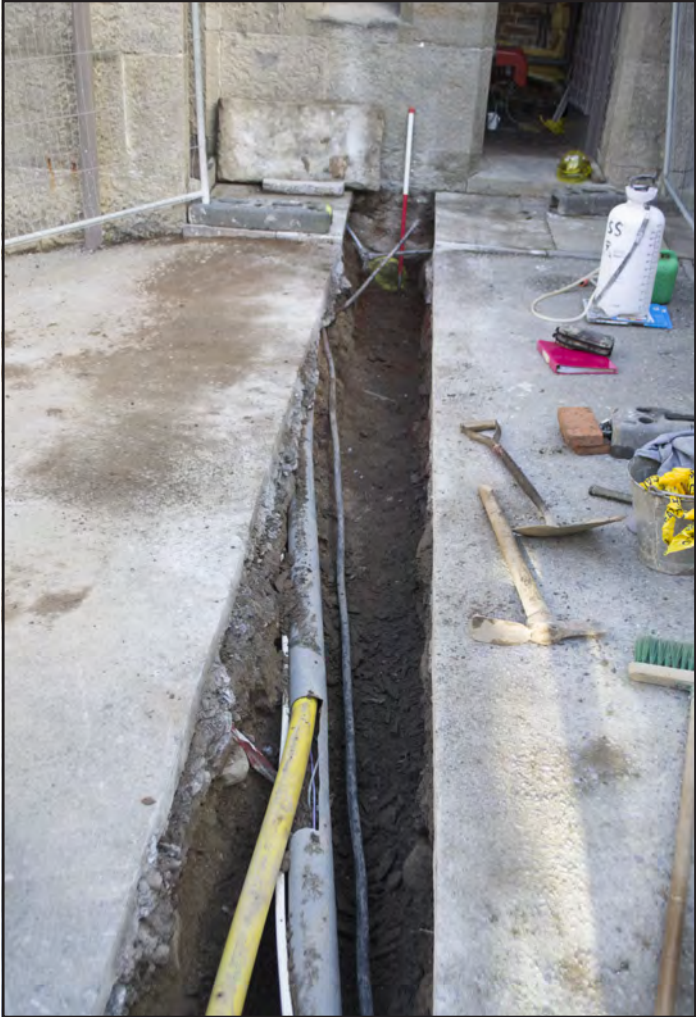
Plate 19: Pipeline 10: Shot of trench leading to N end of castle with damaged bricks and modern services; scale 1m (archive image: G2447_160)
