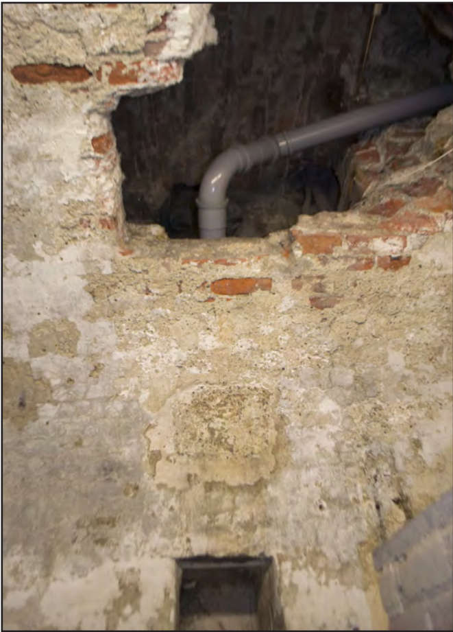
Plate 15: Pipeline 1: Portrait shot of c.30cm x 30cm mortared area - likely to have been [18^] tunnel terminal, along with appearance of lead pipes (archive image: G2447_144)
