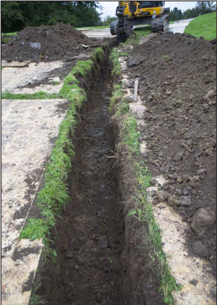
Plate 09: Pipeline 1: Shot along trench during excavation of pipe trench showing previously backfilled area near woodlands (archive image: G2447_123)
