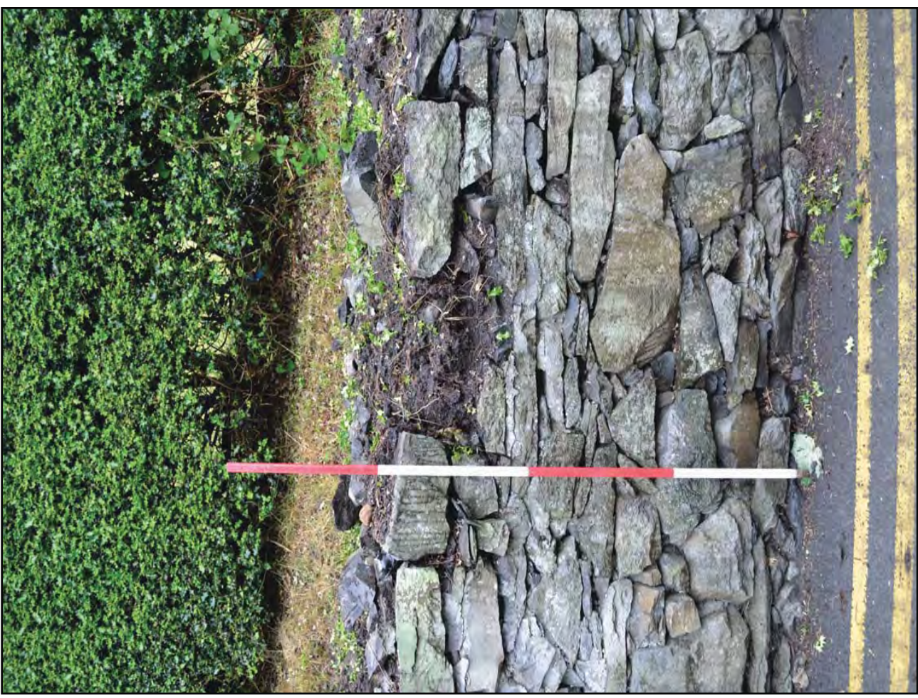
Plate 16: Wall E with large stone removed to aid root removal
