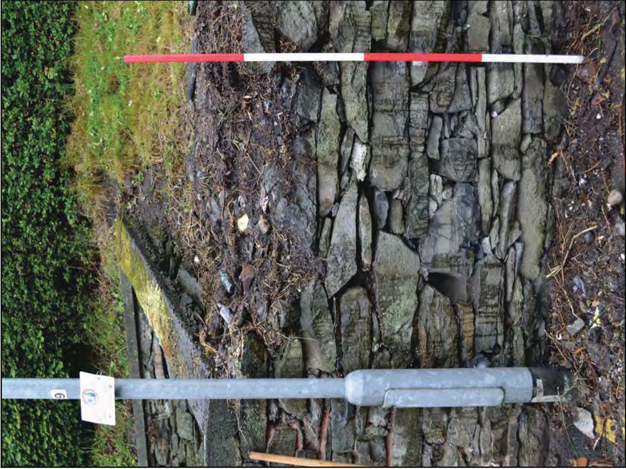
Plate 15: Wall E with top stones removed to aid root removal
