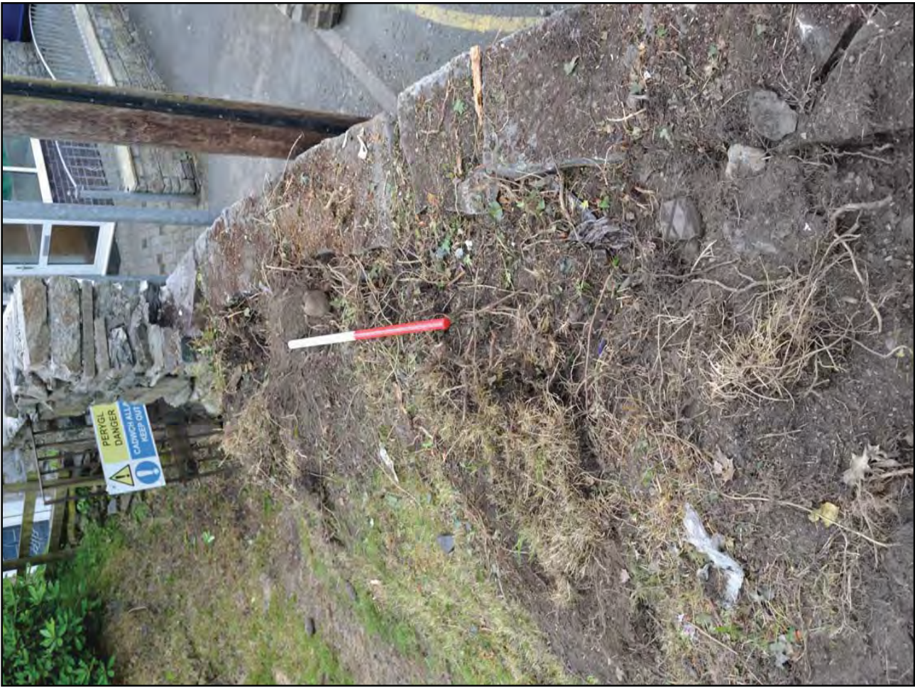
Plate 18: Wall E after root removal
