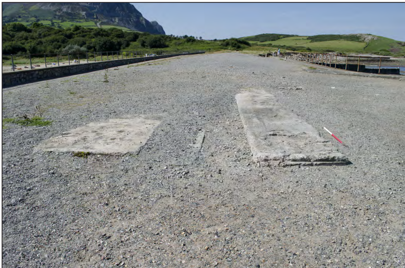
Plate 07 Detail of concrete pads in stone pier surface (Scale: 1 x1m; archive image: G2475_Trefor_Pier_010)
