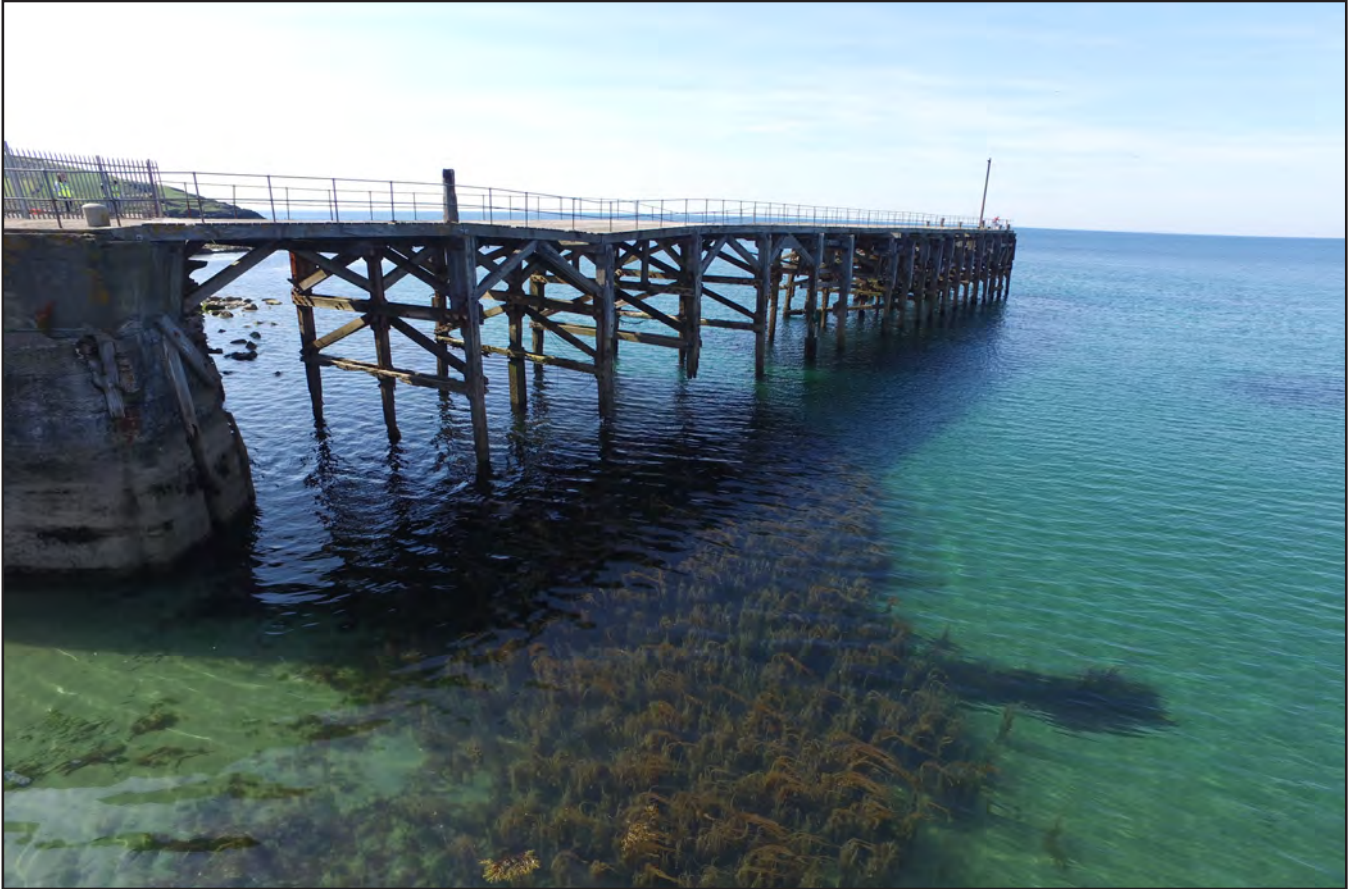
Plate 19: View of north-northwest side of Trefor pier showing rotted timber in the intertidal zone, most notably on Truss 17 (UAV image: DJI_0233)
