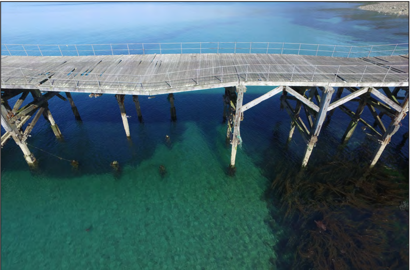
Plate 12: Aerial view of Trefor Pier from the east-southeast showing the condition of timber decking over collapsed trusses (Trusses 12 to 18) (UAV image: DJI_0108)
