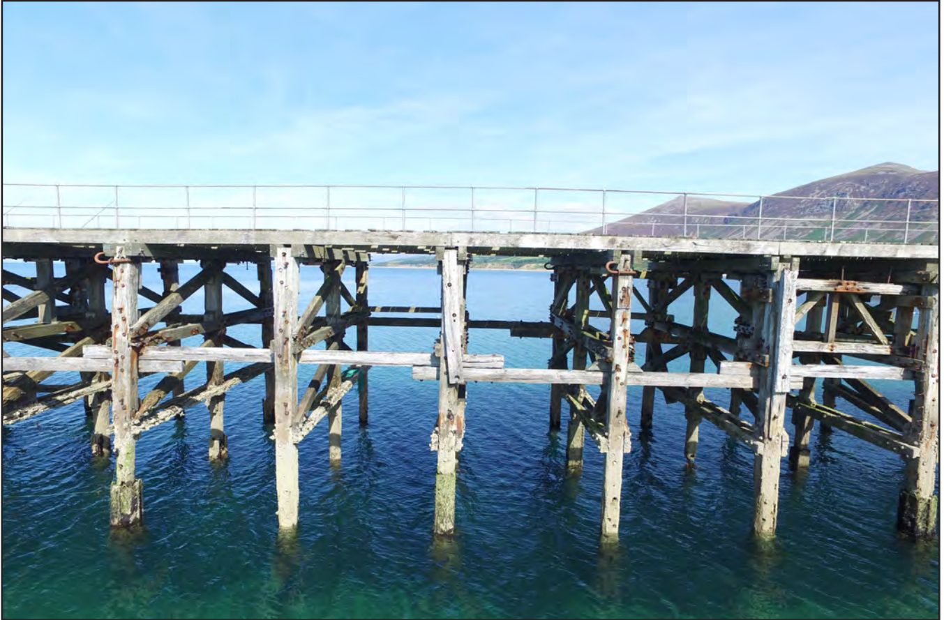
Plate 13: View of Trefor pier from the east-southeast showing the detail of the truss construction (Trusses 5 to 10) (UAV image: DJI_0146)
