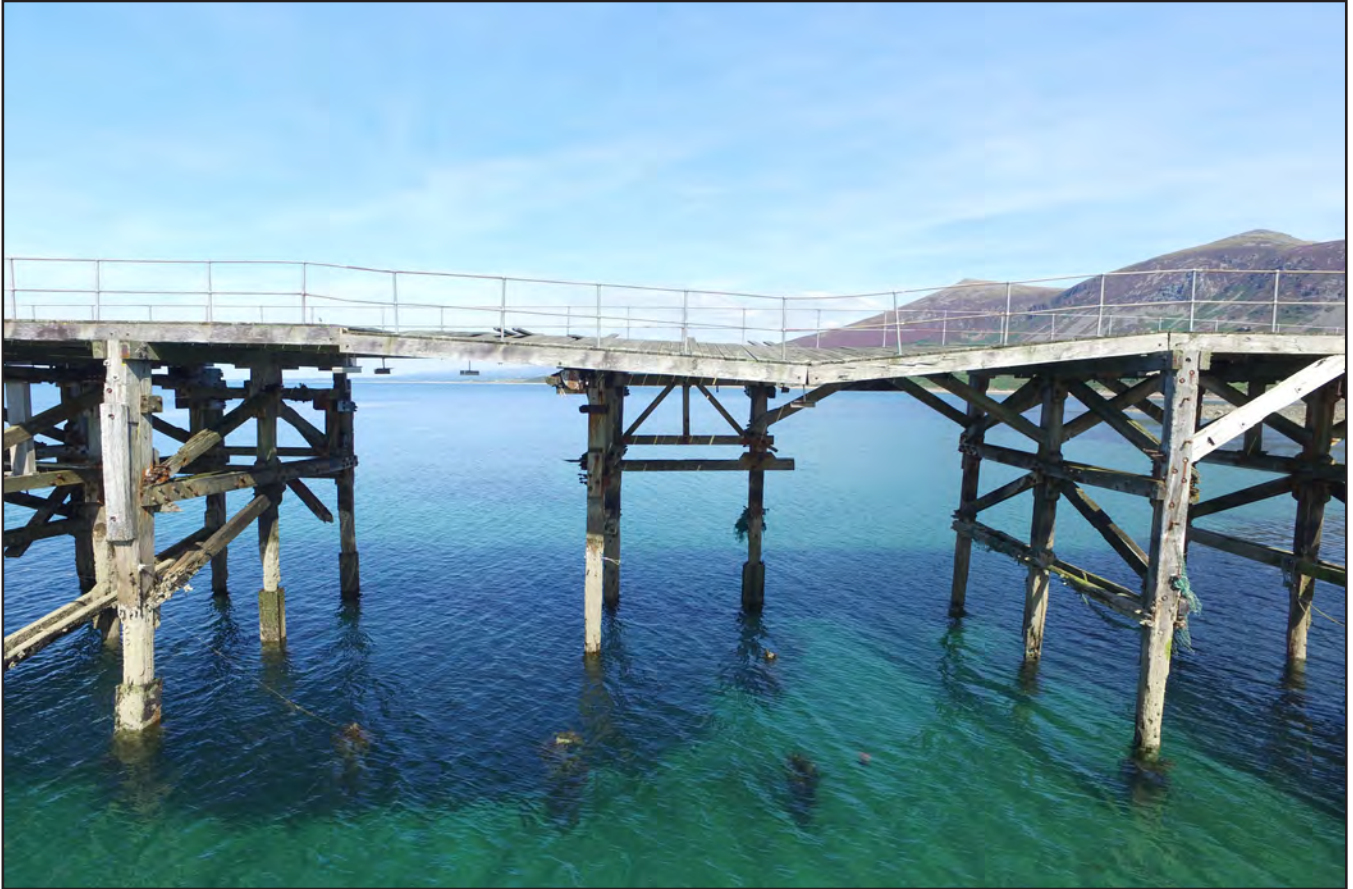
Plate 17: View of Trefor pier from the east southeast showing the damaged section of the pier from trusses 13 to 15 (UAV image: DJI_0143)
