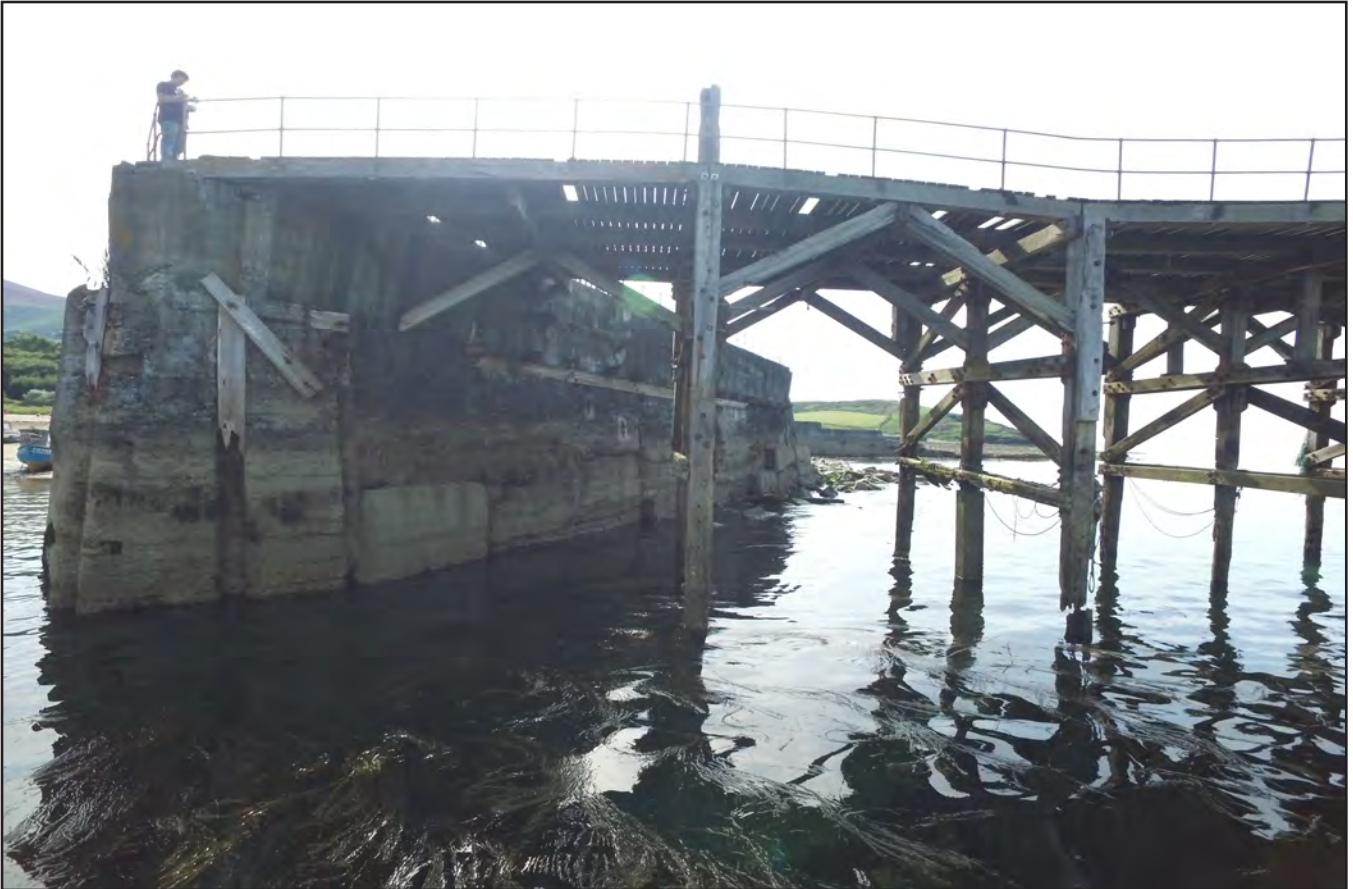
Plate 22: Detail of truss construction and stone pier (Trusses 18 and 19) (UAV image: DJI_0698)
