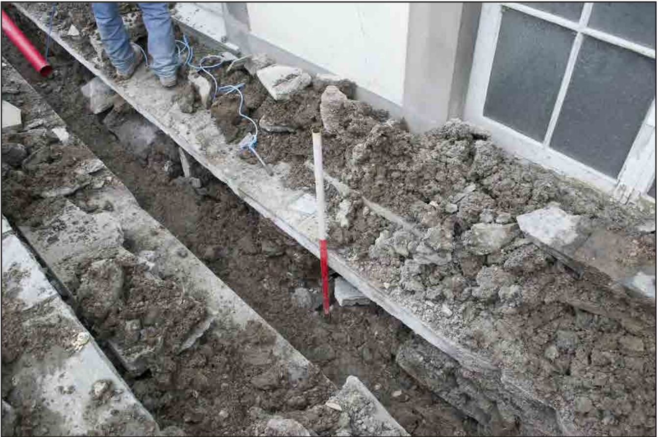
Plate 01: Excavation of electrical cable trench to north of Bishop's Palace Room GF03 monitored by GAT on the 29th May 2014. Scale 1x1m.
