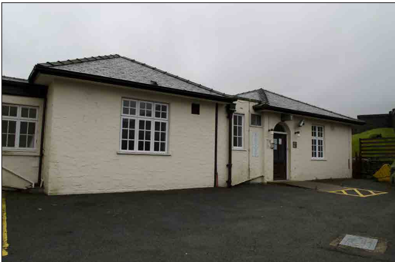
Plate 06: Side Elevation (west wing) - detail of west wing showing hip gable slate roofing. This part of the west wing is a post-1925 extension (archive image: G2459_010).
