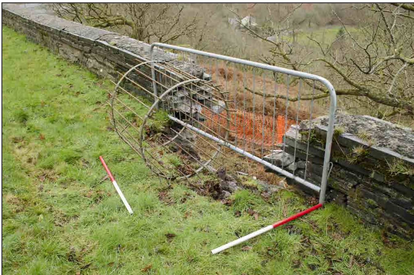
Plate 16: Detail of an existing breach in the boundary wall of the memorial garden; note the slate core of the wall. Scale: 2 x 1.0m (archive image: G2459_032).
