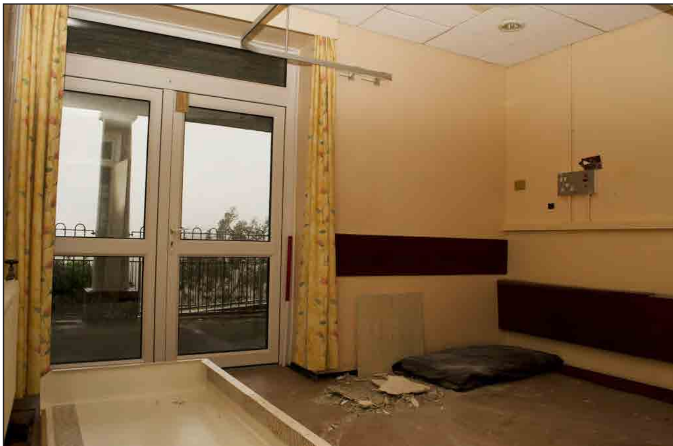
Plate 40: West Wing - Room G20 (2 Bed Ward): view south looking to the rear of the building. This room is within the original part of the west wing and has always functioned as a 2 Bed Ward. The double doors open onto the veranda; this is an original feature but the fittings have been replaced with modern uPVC. Scale: 1.0m (archive image: G2459_122).
