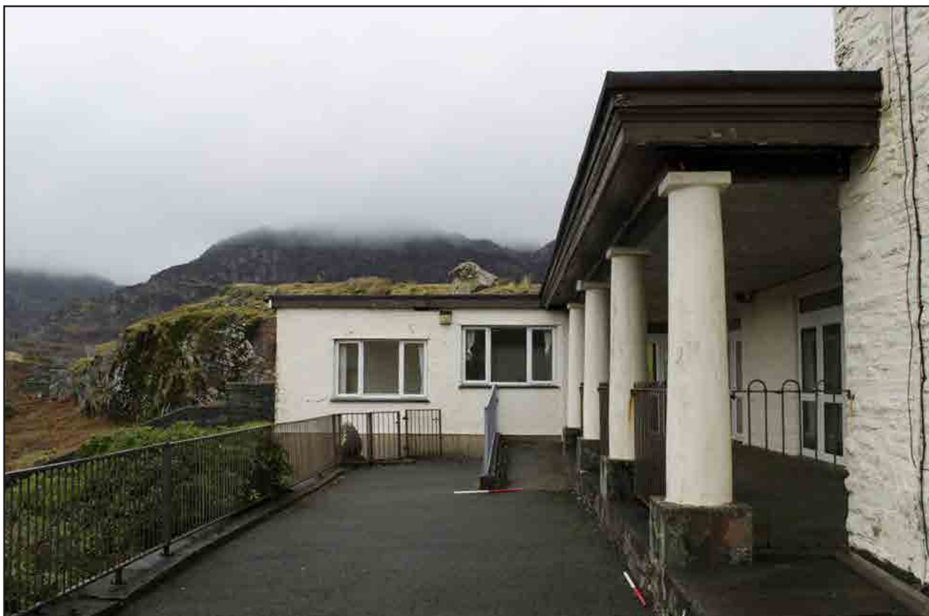
Plate 08: Side and Rear Elevations - view west of west wing. The flat roofed part of the wing is a post-1972 extension which included a dayroom. The veranda in the foreground is part of the original 1925 building although the veranda roofline was subsequently modified when the wing was extended. Scale: 2 x 1.0m (archive image: G2459_017).
