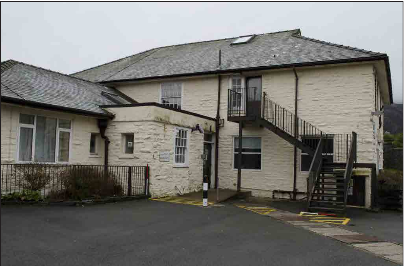
Plate 10: Side Elevation (east wing) - view southwest of wing as seen from the front of the hospital. The wing projects from the main building core. The flat roof portion of the wing is the original staff entrance, whilst the hip gable portion includes the patient wards. The windows are all in their original positions. The fire escape on the main building core is a modern addition, with the fire escape door utilising an earlier window that has been enlarged. Scale: 2 x 1.0m (archive image: G2459_025).
