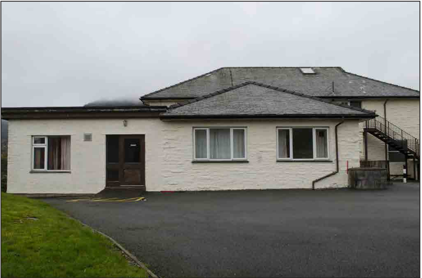
Plate 09: Side Elevation (east wing) - view west; the east wing comprised a hip gable slate roof wing that projected at a right angle to the main building and originally housed the male ward and staff entrance. The hip gable part of the wing is from the original building; the flat roof belongs to a post-1972 extension for a dayroom that removed the veranda. The windows in the original part of the wing were added during the construction of the dayroom extension. Scales: 2 x 1.0m (archive image: G2459_024).
