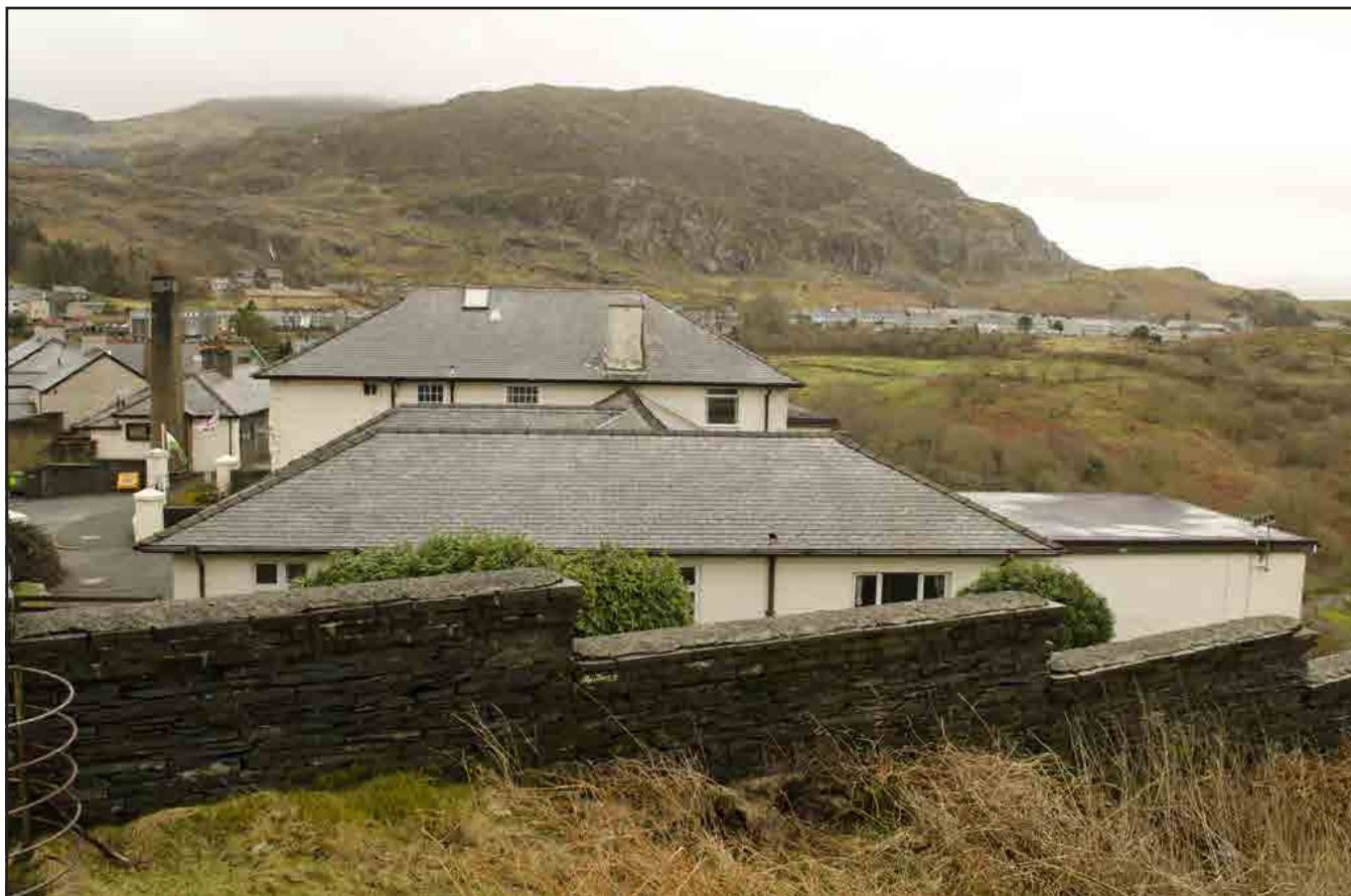
Plate 07: Side Elevation - view east of the west wing and main building core, detailing the hip gable slate roofs used for the main building and parts of the west wing, as well as the flat roofing used at the rear of the west wing. The main building core is part of the Original building, along with part of the west wing visible beneath a chimney at the centre of the image. The remaining parts of the building are extensions (archive image: G2459_011).
