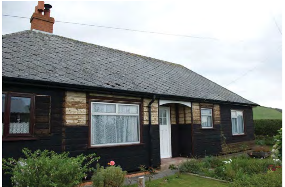
Plate 19. No. 7, Marconi Bungalows, Tywyn (PRN 60173) with render removed for repairs, showing original weather boards and part of a blocked window
