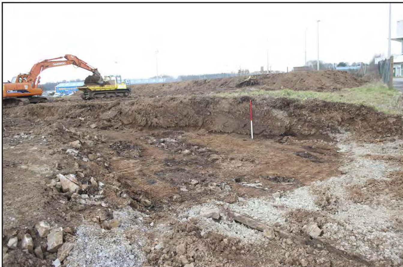
Plate 09: View northwest during groundworks detailing degraded stone and the glacial horizon in the foreground. Excavation depth was 1.0m (Scale: 1 x 1.0m; archive image: G2461_034)
