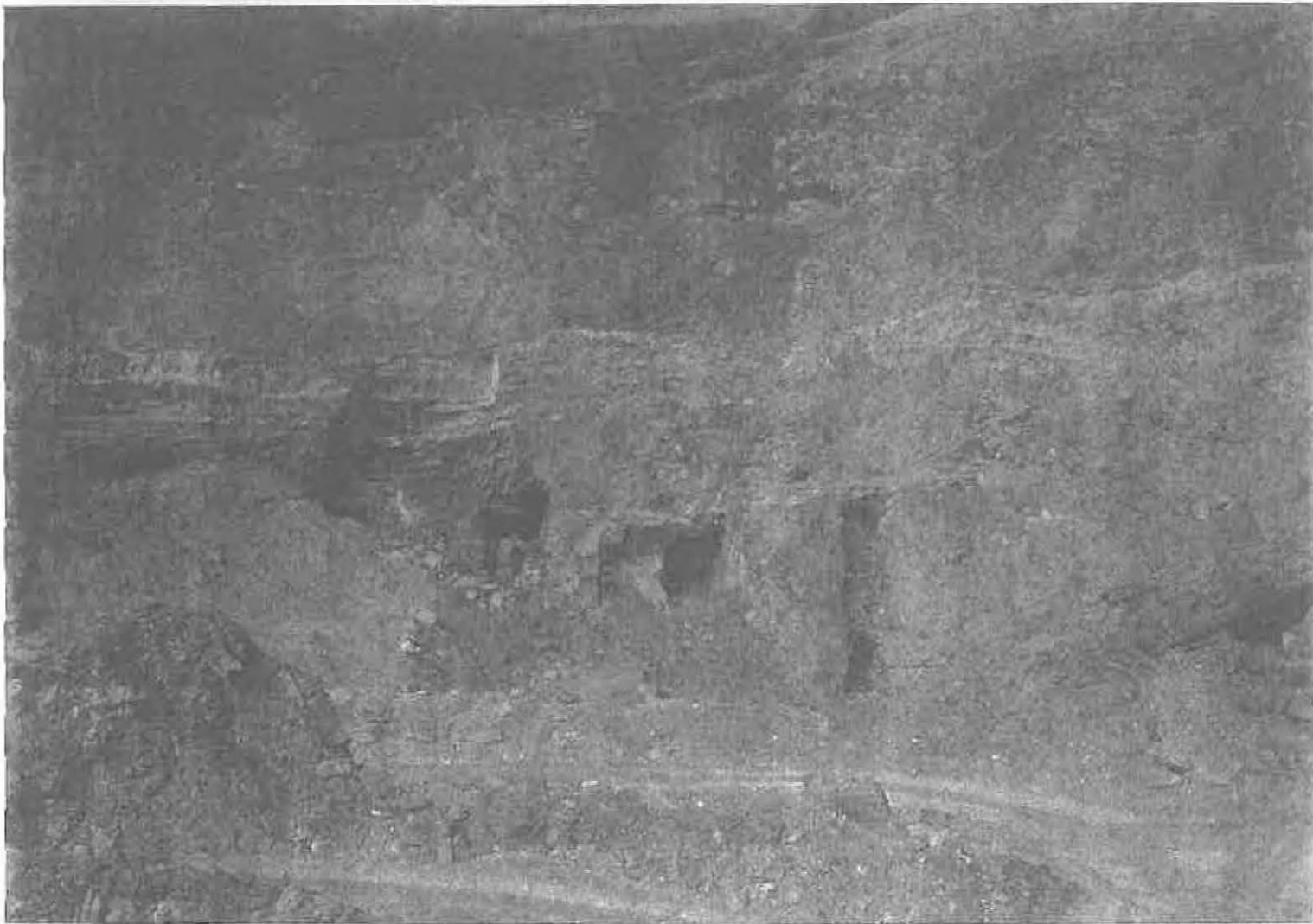
The process of untopping what had been an underground quarry in order to work it as an open-cast, showing the dip of the strata and the system of chambers from which the slate was extracted.
