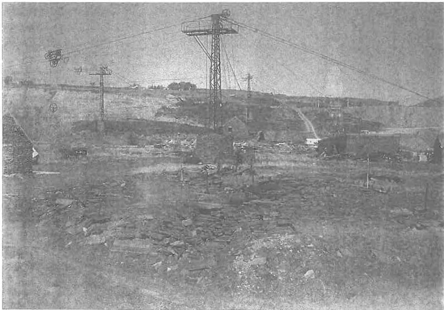
A view of the bank on a pit quarry, showing the blondins, a transshipment shed and an electricity sub-station.
