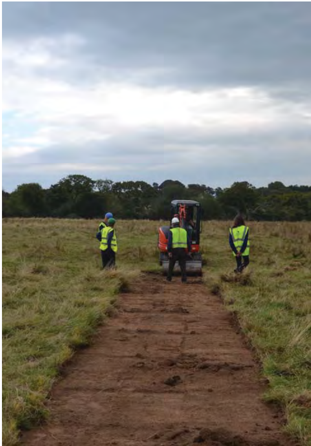
Plate 3. Mini-digger stripping topsoil and ploughsoil from trench 1 under archaeological supervision
