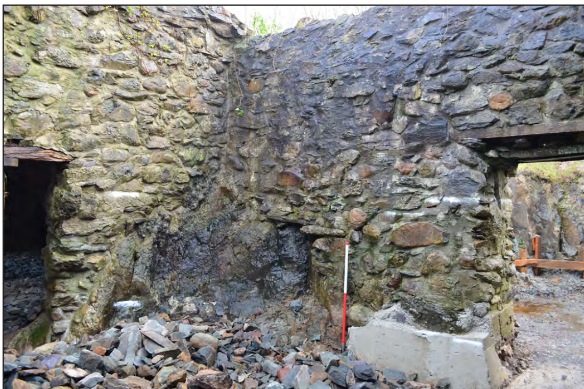
Plate 16: Southwest room - internal elevation: bedrock built into the east corner (Scale: 1 x 1.0m)
