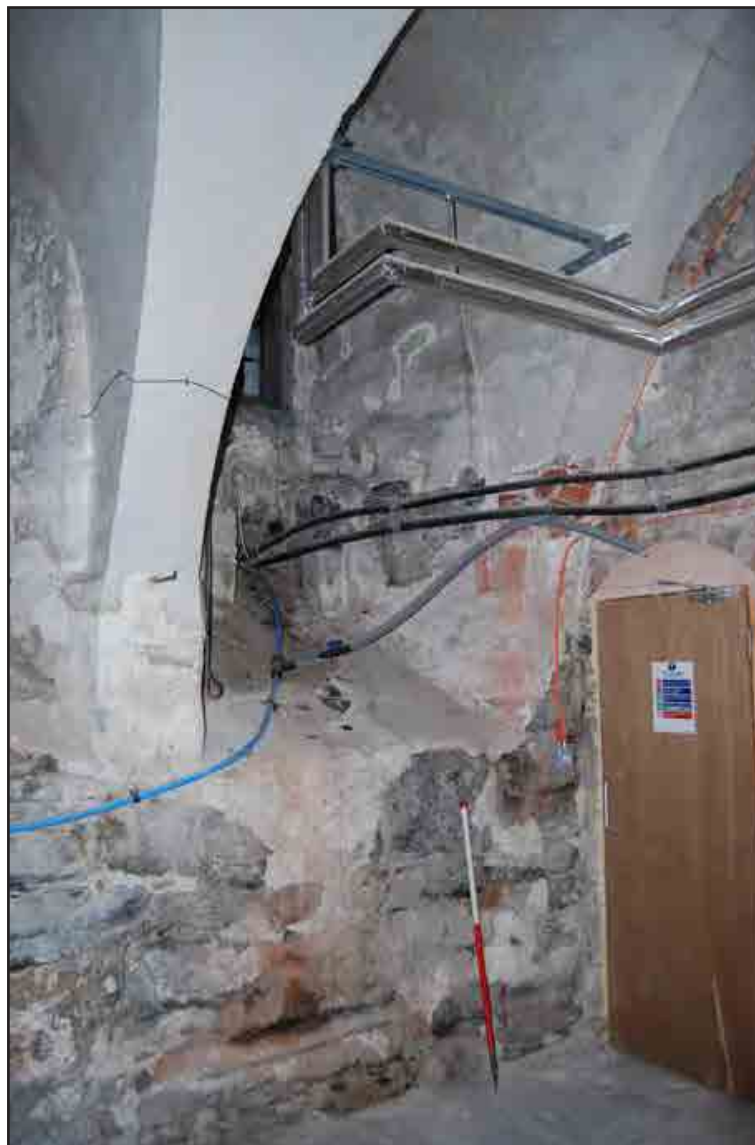
Plate 11: Cellar - view from within cellar of access point for the heat main from the courtyard. The heat main will use the same access point and route as the existing pipes. Scale: 1 x1m.
