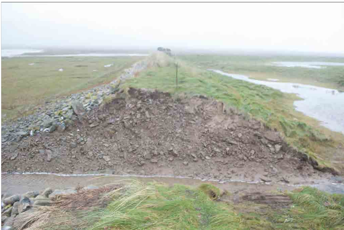
Plate 04: West facing section through the bank after machining.
