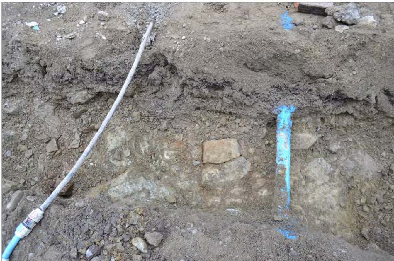
Plate 01: Possible metal surface in open cut trench, with services crossing the trench. Section between G9-G10. No scale. Viewed from the North-West.
