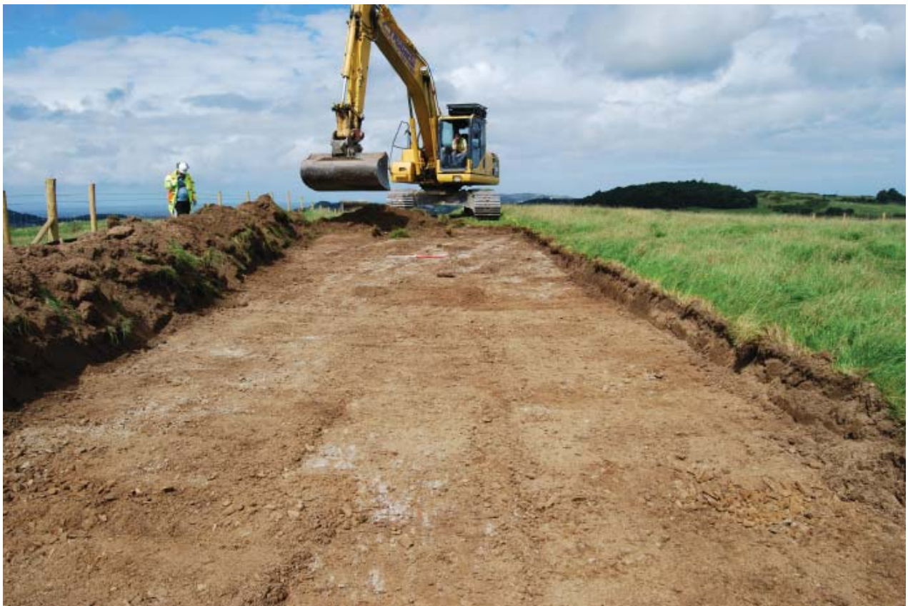
Plate 8: Working shot taken during the topsoil strip of the overflow pipeline route. View from the northeast.
