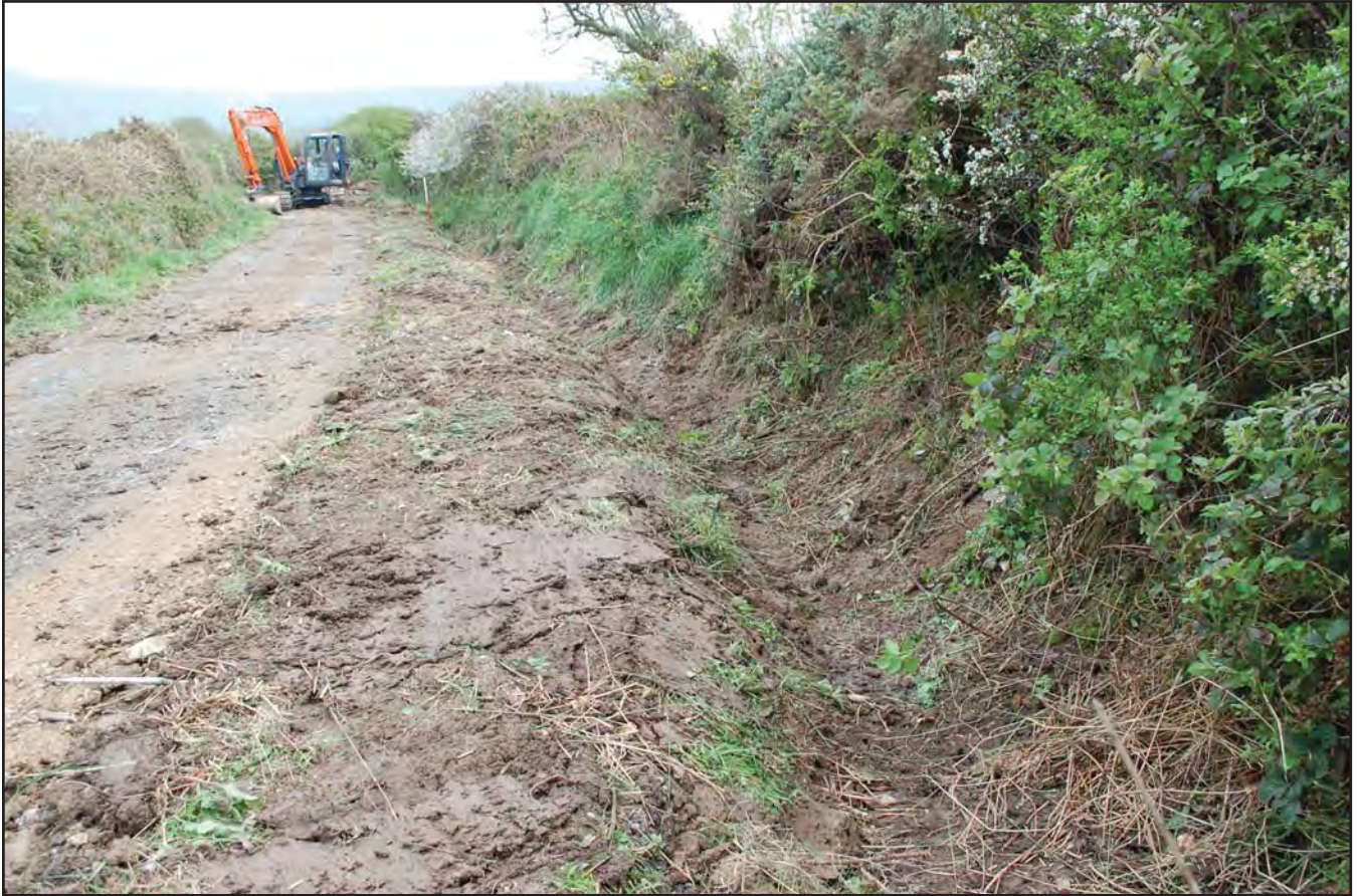
Plate 03: Section C of the opencut trenching, showing the verge cleared along the track ready for the new pipe. View from the NW
