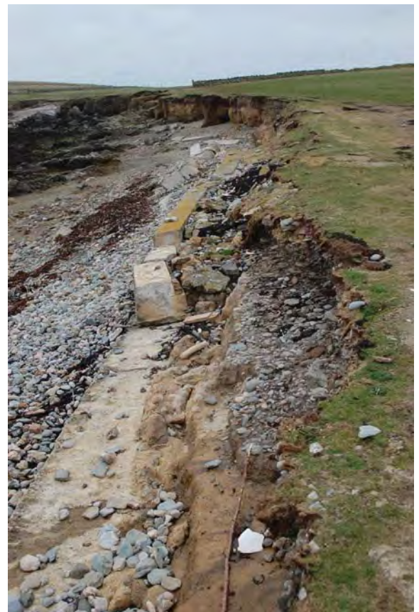
Plate 2. Collapsed sea defences at Henllwyn, view from E
