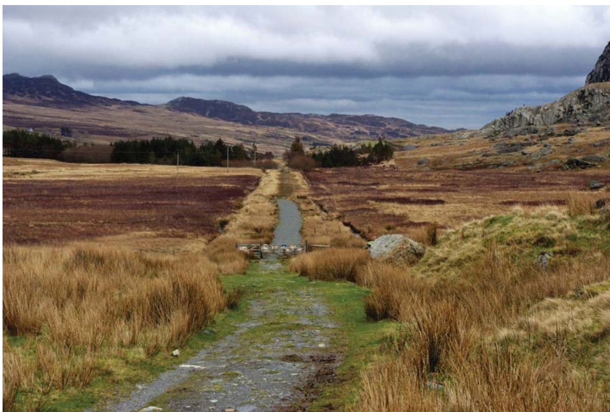
Plate 8 Partly resurfaced turnpike embankment crossing bogs (PRN 58542)
