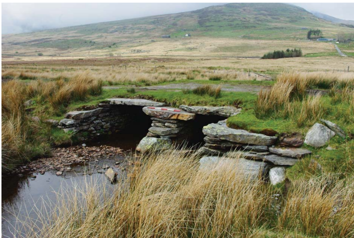
Plate 11 A well preserved stone culvert beneath Nant y Benglog turnpike (PRNs 3278 and 37327)
