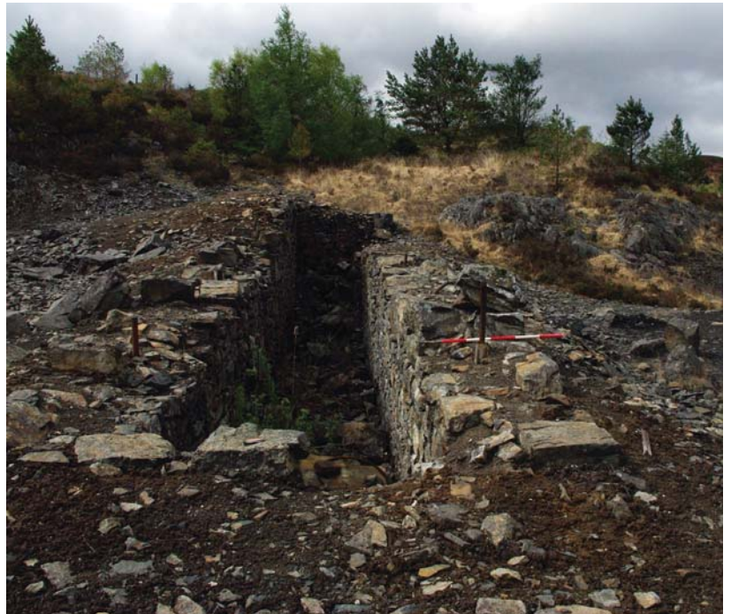
Plate 35. Wheelpit associated with the Willoughby Mine dressing floor (NPRN 533510)
