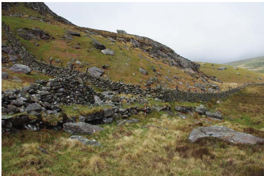
Plate 37. Revetment supporting northern side of Lord Penrhyn's Road, Nant y Benglog (NPRN 534077)
