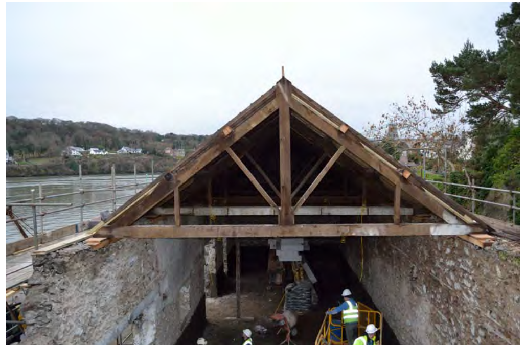
Plate 08: Exposed roof timber trusses. View from the north.
