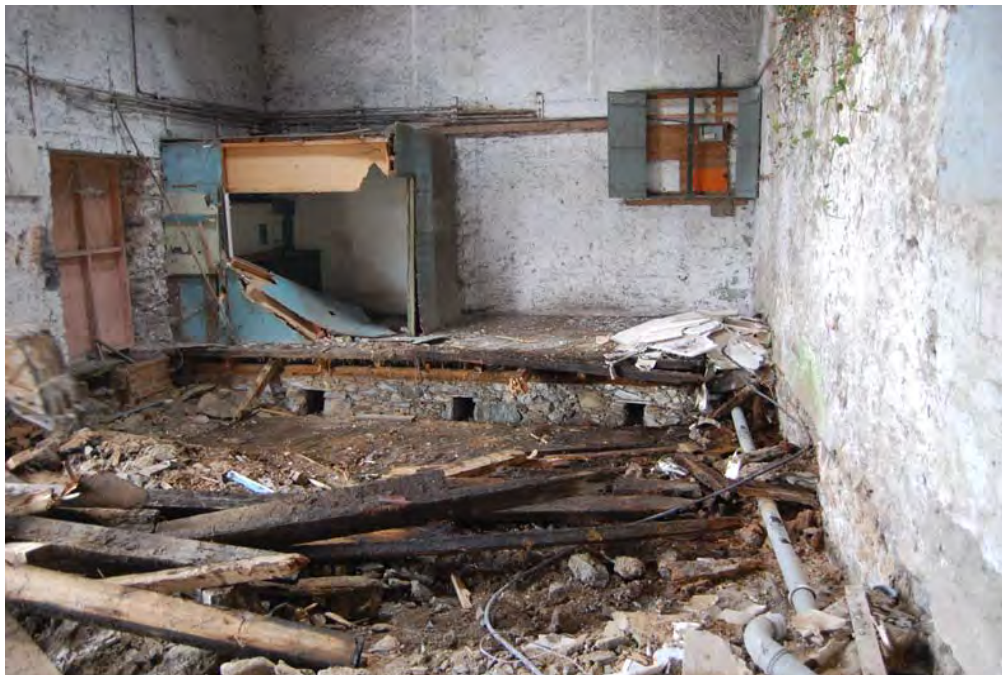
Plate 06: Dwarf Walls exposed during works. View from the NNW.
