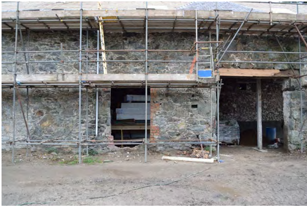
Plate 05: External eastern elevation showing partially bricked up doorway. View from the east.
