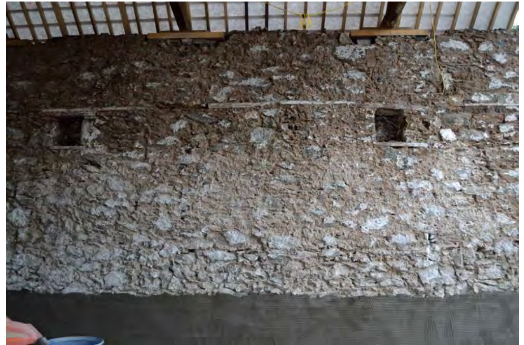
Plate 03: Internal western elevation wall with render removed showing recesses for first floor beams. View from the east.
