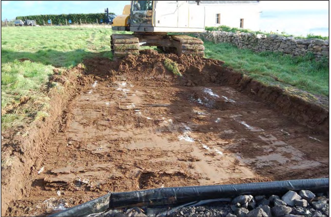
Plate 01: Stripping of Access Road. View from the southwest.
