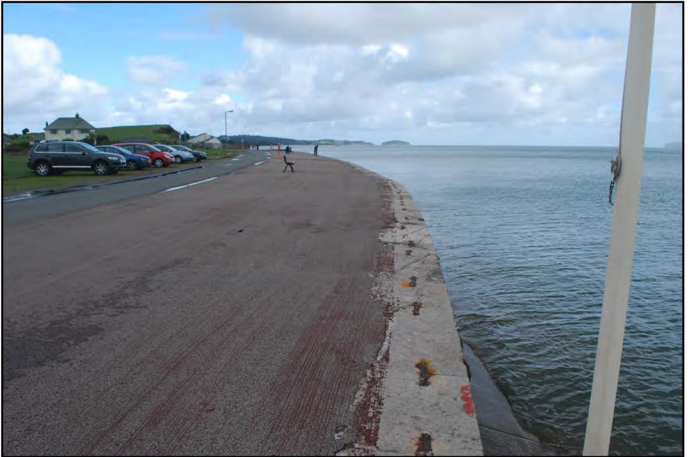
Plate 05 - View of the flood defence wall at the Green (Area 3, Feature 1). View from the south
