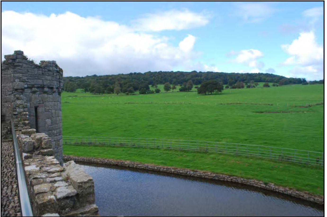
Plate 07 - View across the meadow to the north ofg Beaumaris castle from the outer curtain wall (Area 2), looking towards Baron Hill
