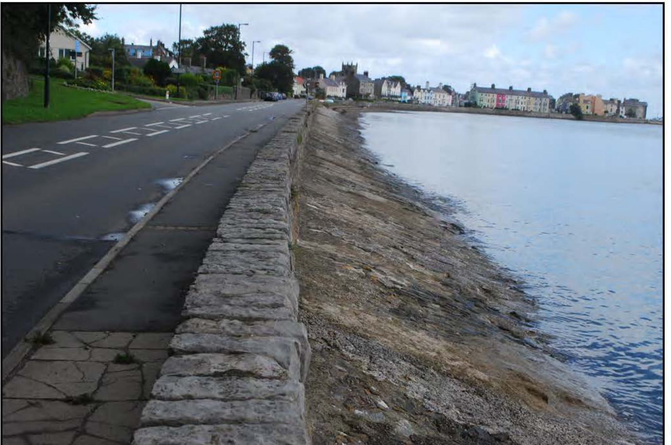
Plate 02 - View of the flood defence wall near Townend (Area 4, Feature 1). View from the south-east
