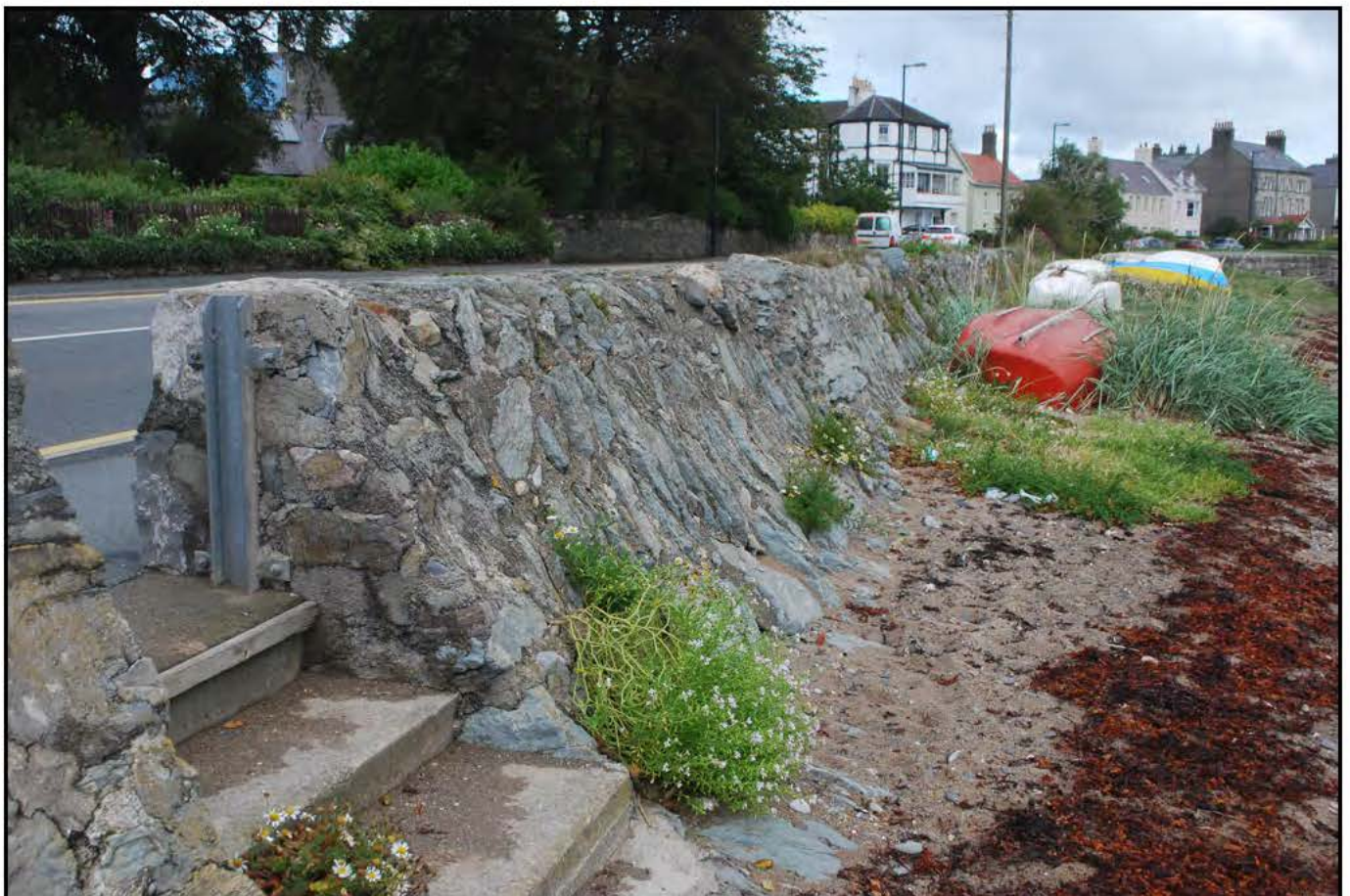
Plate 04 - Detail showing the batter on the flood defence wall in Area 4 (Feature 1). View from the north east
