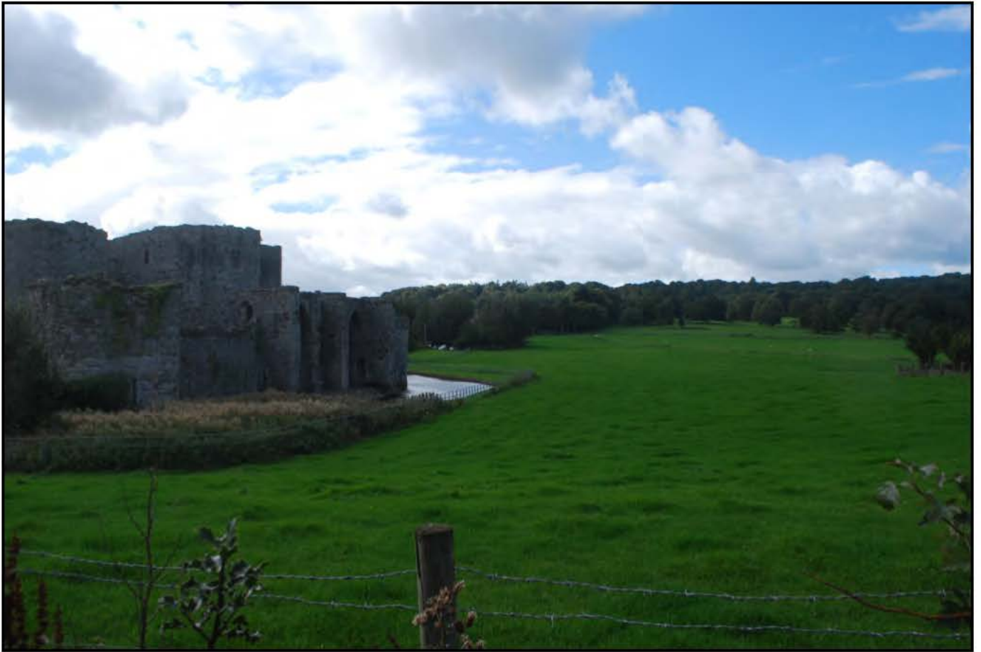
Plate 11 - View of Beaumaris Castle and the meadow to the north, taken from the east
