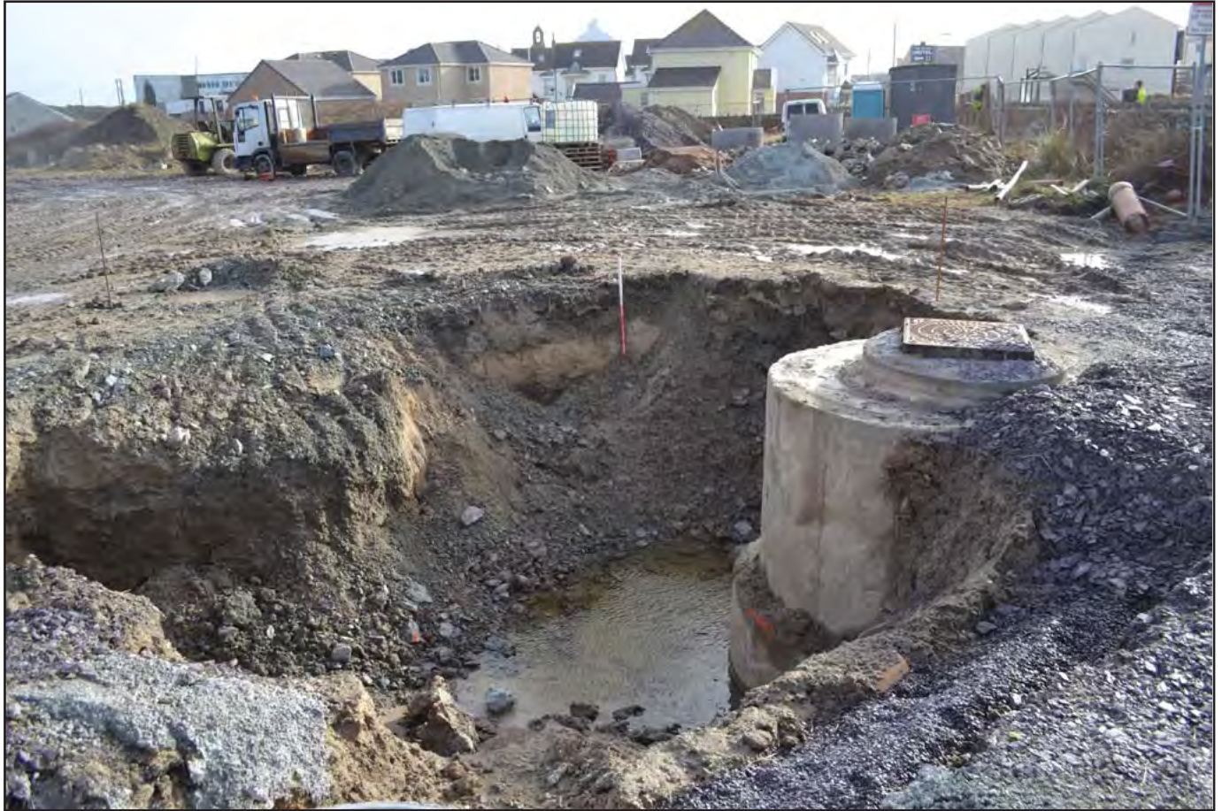
Plate 03- View southeast of exposed Dwr Cymru inspection chamber (completed 2008) and associated disturbance. The excavation zone around the chamber was re-dug to accommodate the 2013 drainage works for housing development. Mean depth was 1600mm (Scale in background is 1000mm).
