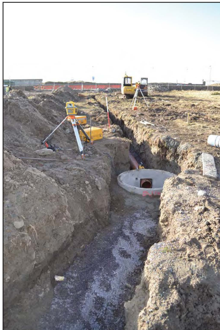
Plate 06 - View west of partly backfilled service drainage trench/new inspection chamber (length: 30.0m; depth: 1000mm). Trench excavated into imported material and not local sand deposits.
