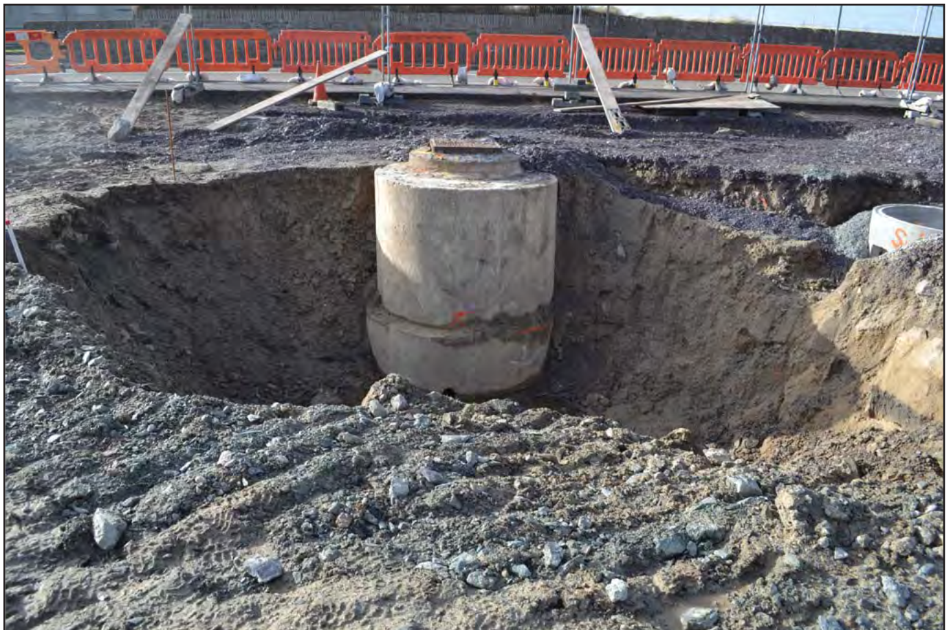
Plate 04 - View south of exposed Dwr Cymru inspection chamber (completed 2008) and associated disturbance. The excavation zone around the chamber was re-dug to accommodate the 2013 drainage works for housing development. Mean depth was 1600mm
