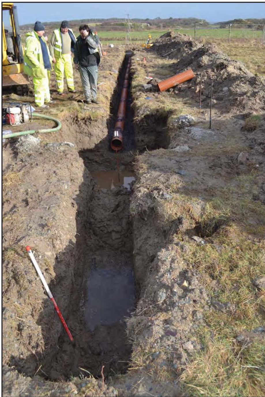
Plate 05 - View northeast of service pipe trench (length: 35.0m; depth: 1000mm). Trench excavated into imported material and not local sand deposits
