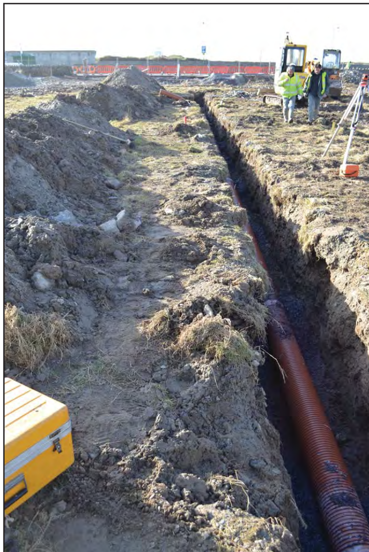
Plate 08 - View west of partly backfilled service drainage trench leading toward Lon St Ffraid (length: 30.0m; depth: 1000mm). Trench excavated into imported material and not local sand deposits.
