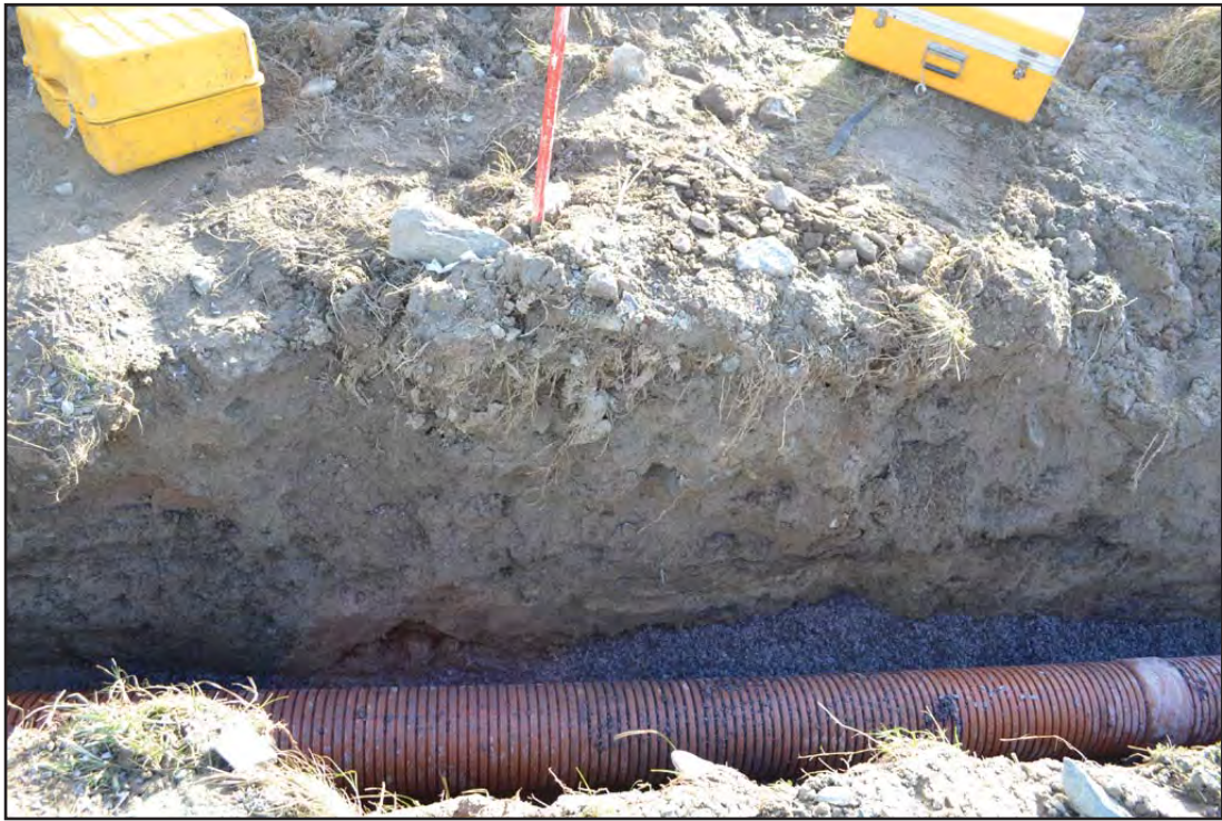
Plate 07 - northwest facing section of new service trench, detailing made ground deposit (imported material). Mean trench depth was 1000mm.
